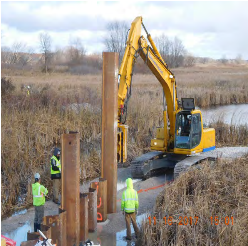
Steel Sheet Pile Segment
