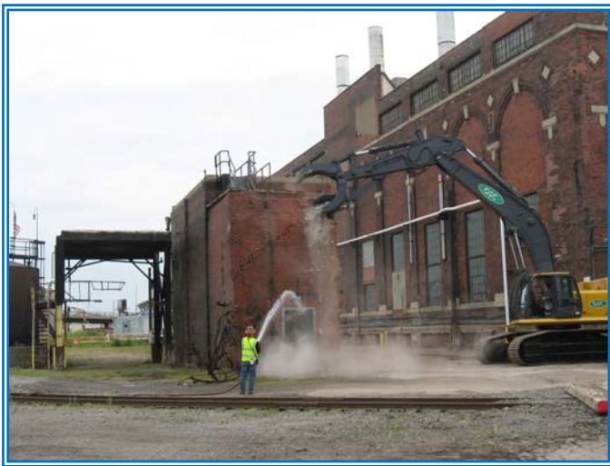
Demolition work at Buffalo Color Site
