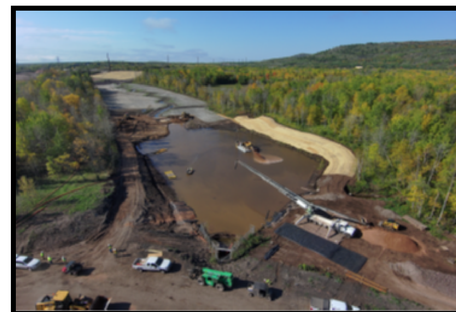
Clean cap material placed in Weir Pond using a spreader barge.
