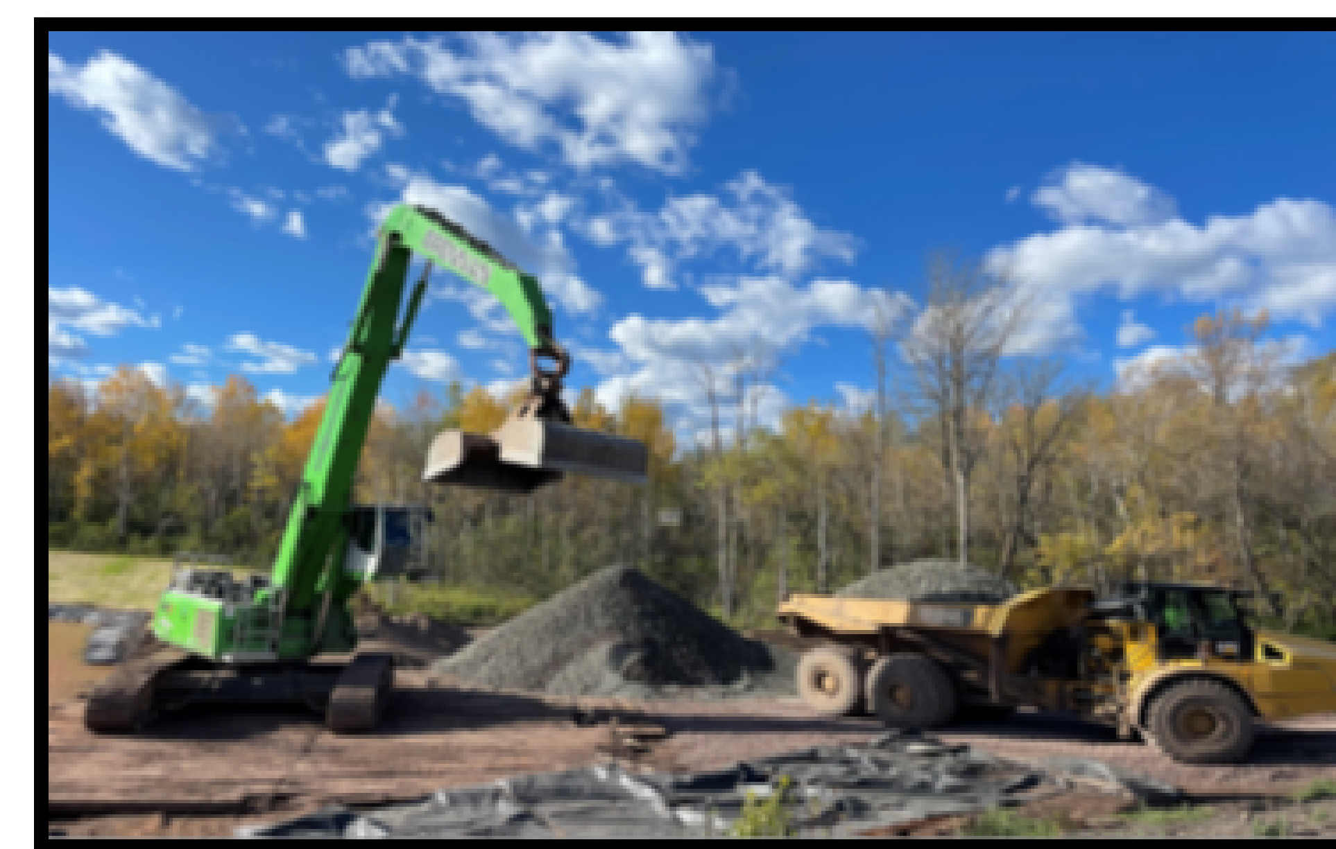
Armor stone is loaded for capping in the Unnamed Creek area.
