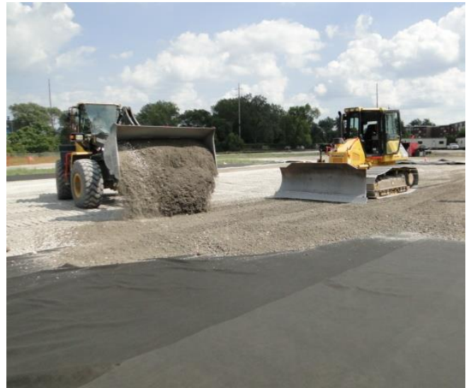
Preparing the Stateline project area for cleanup activities.
