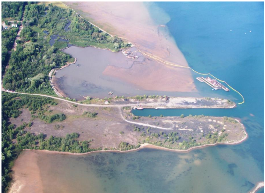
Aerial view of Tannery Bay. The dredging operation platform can be seen on the right.
