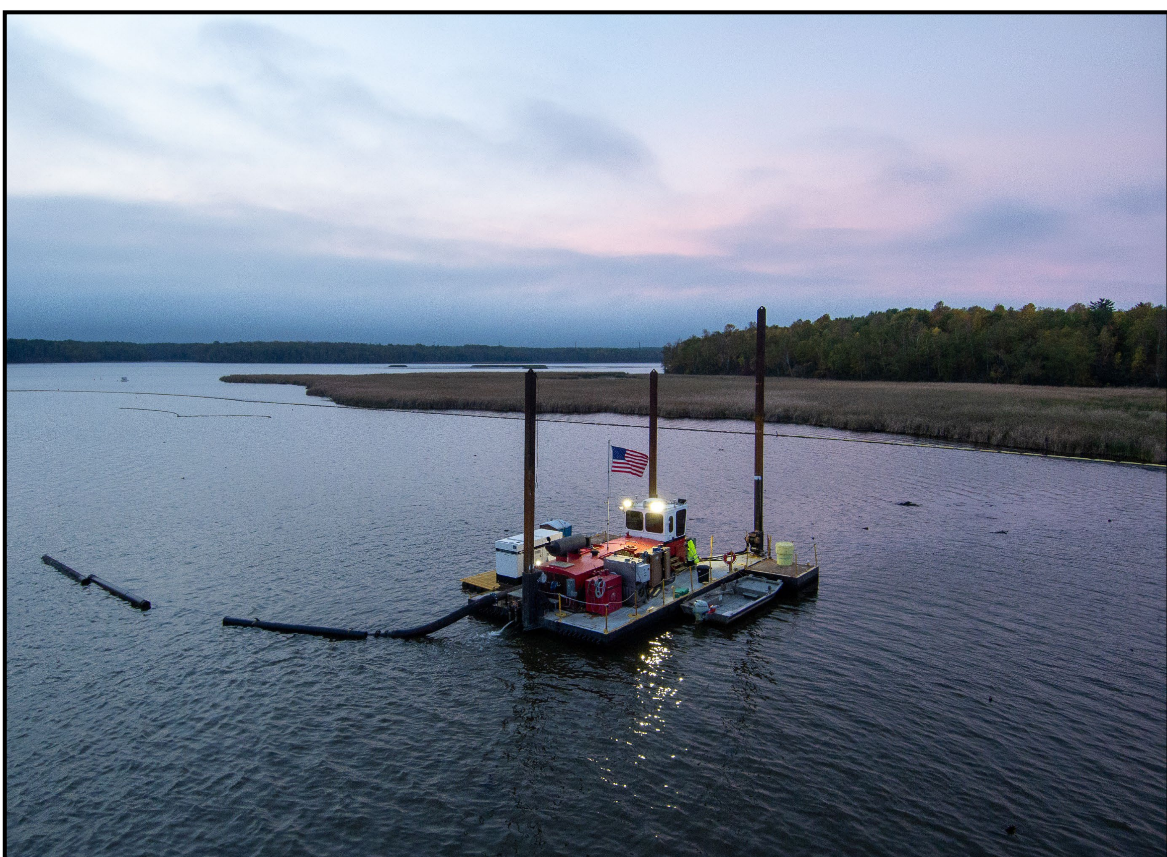
Hydraulic dredge at Spirit Lake.
