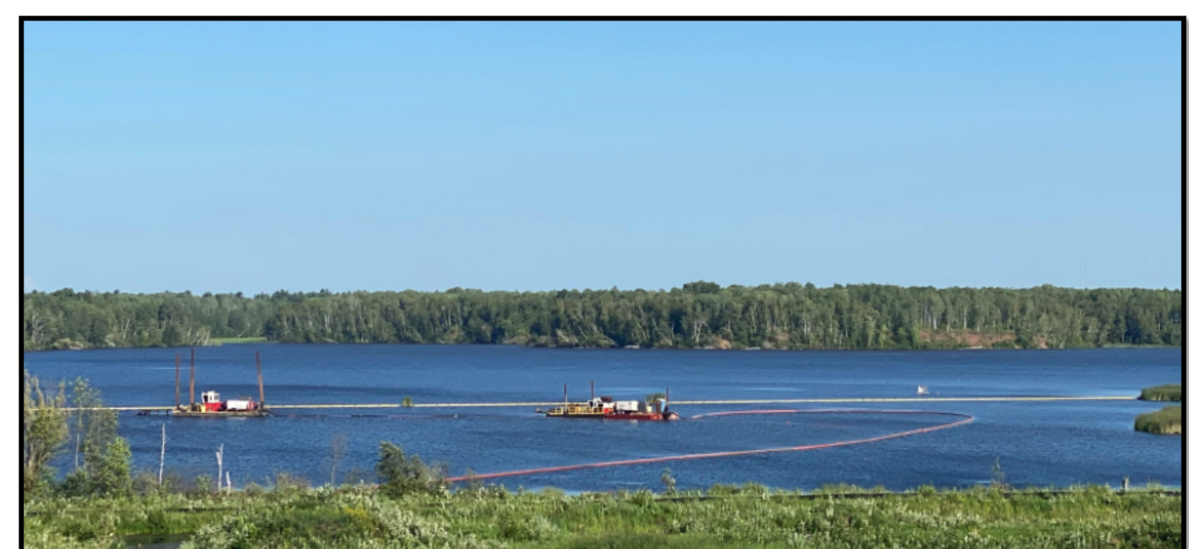
Turbidity curtains deployed during hydraulic dredging in Wire Mill Delta.
