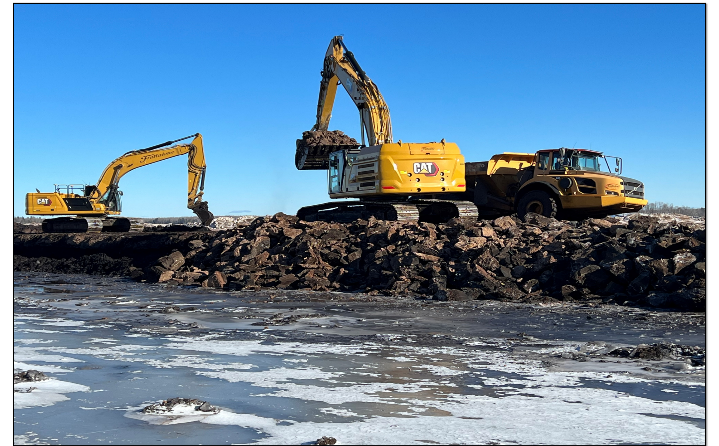
Dredging is conducted with a mechanical dredge in the Shallow Sheltered Bay.
