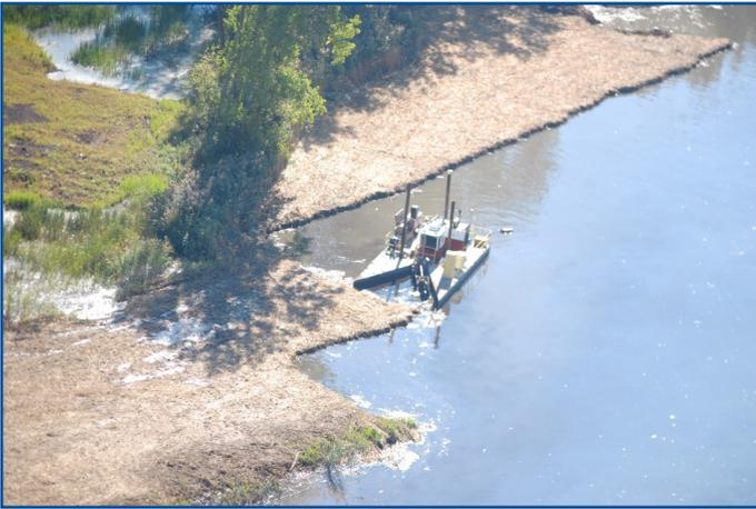
*This photo shows the equipment used to remove the polluted mud. This process is called hydraulic dredging. The mud is removed from the river and pumped through a pipeline that sends it to a separate area to dry out.*
