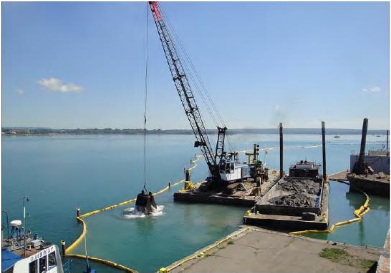
Dredging with machinery like this clamshell bucket will remove approximately 160,000 cubic yards of contaminated sediment from the portion of the Sheboygan River running from Kiwanis Park to the 8 th Street bridge as part of the Great Lakes Legacy Act dredging project. Similar equipment will remove approximately 170,000 cubic yards of additional sediment downstream of the 8 th Street Bridge.
