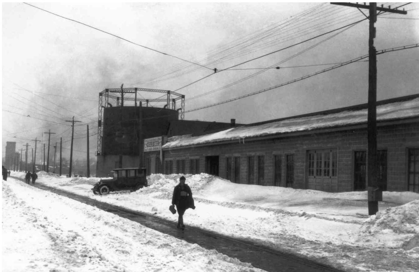
*A 1929 photo shows a cylindrical “gas holder” that was part of the manufactured gas plant on the St. Marys River. The building in the foreground is not part of the plant. Photo courtesy of Consumers Energy Co.*
