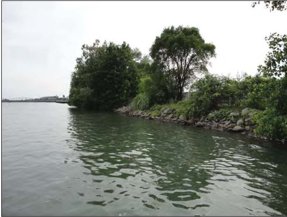
Construction debris rip rap with vegetation
