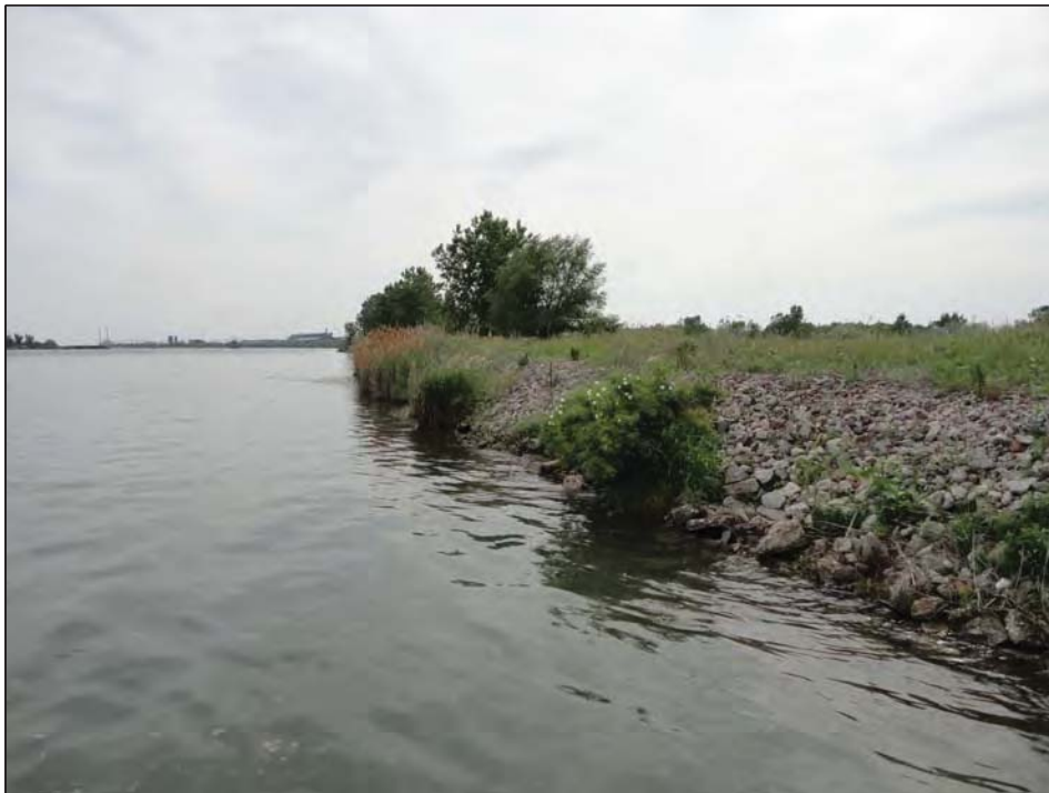
Construction debris rip rap with vegetation
