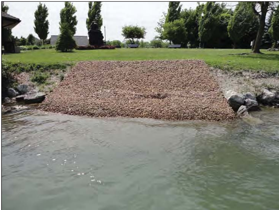
Rip Rap with patch of experimental rocky shoreline
