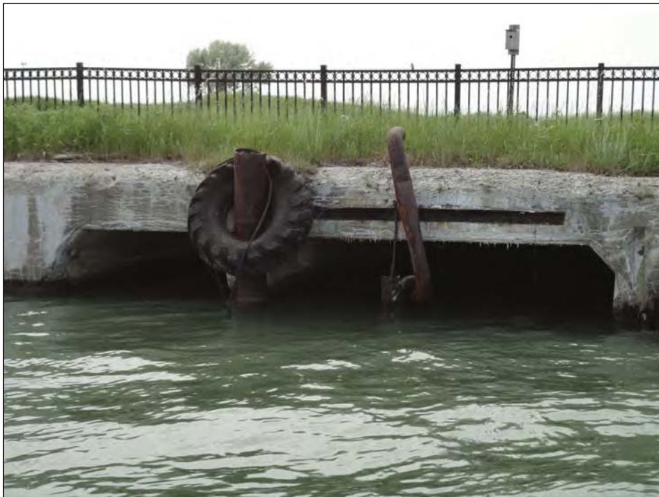
Concrete with two side-by-side box sewers (concrete)
