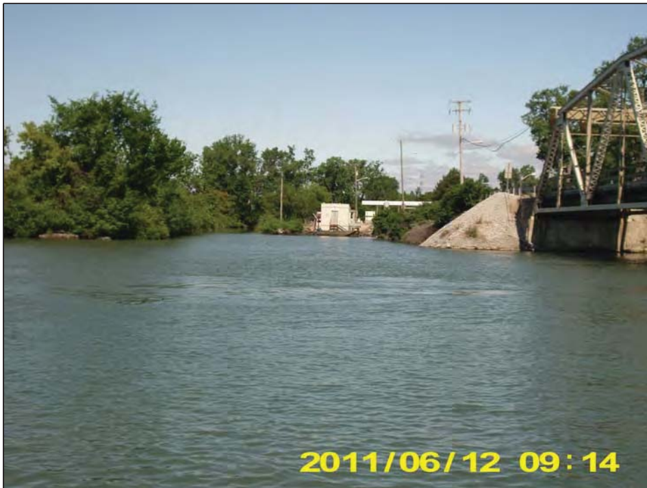
Rip Rap with vegetation
