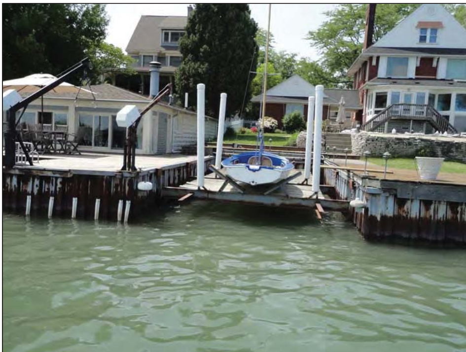
Steel Sheetpile with boatslip
