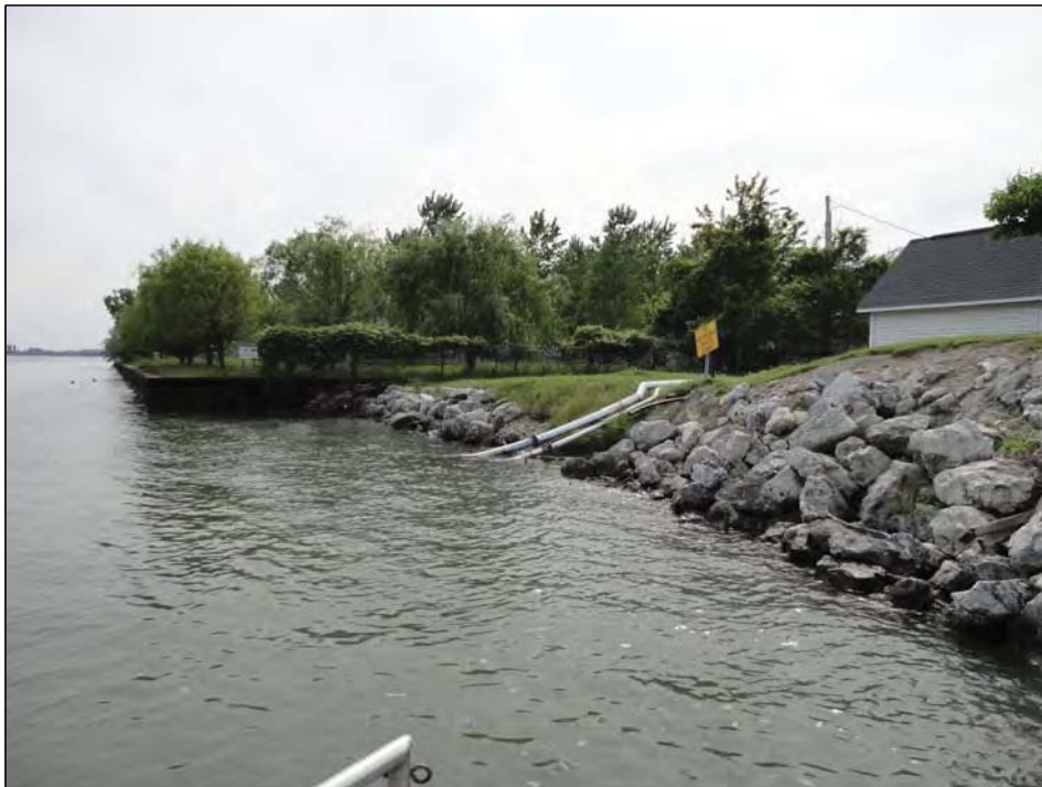
Rip Rap with water intake lines and pump for golf course (PVC, about 4" and 6")
