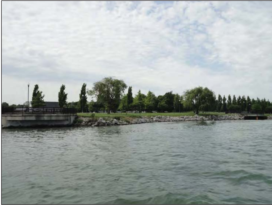
Rip Rap with concrete and steel sheetpile overhanging seating areas
