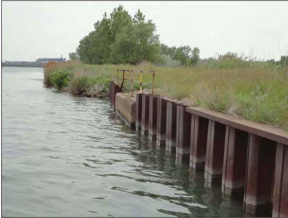
Steel Sheetpile with concrete portion of wall having steel plate/grate access doors on top
