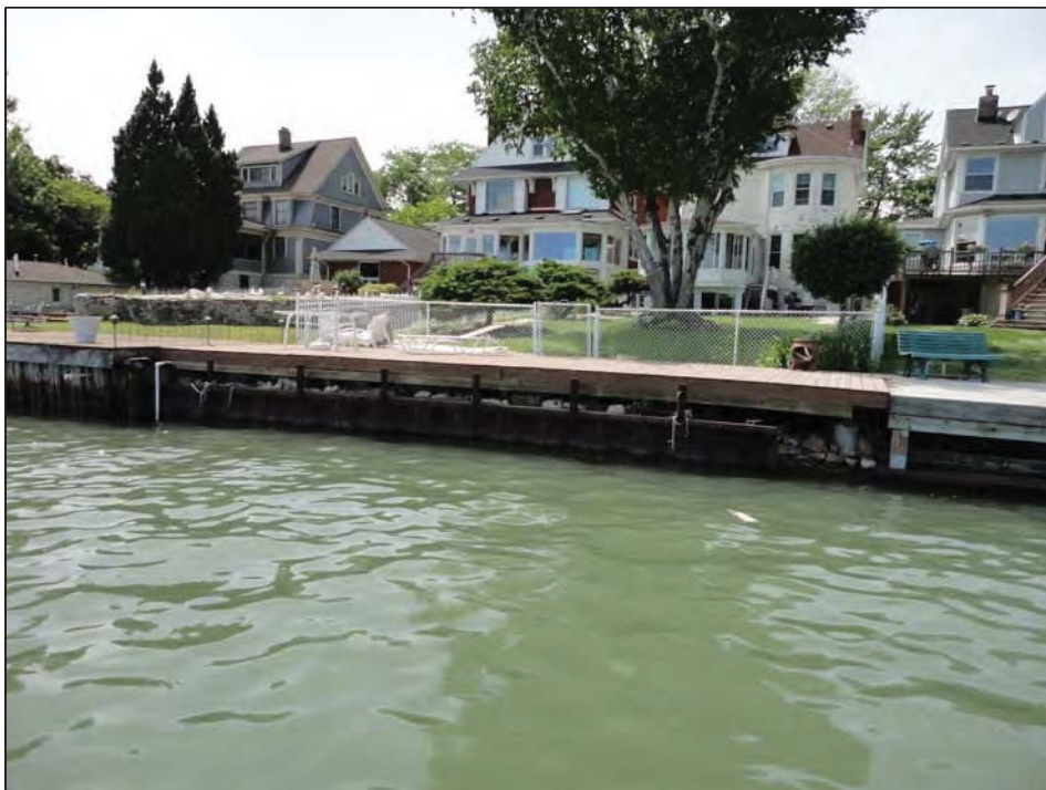
Steel Sheetpile with Rip Rap visible behind
