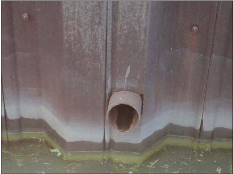
Steel Sheetpile with steel outfall pipe (about 6")
