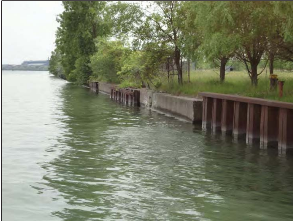
Concrete and Steel Sheetpile
