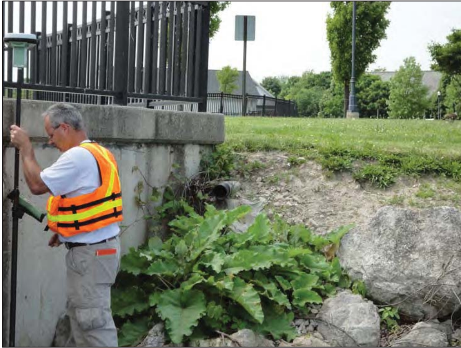
Rip Rap with drain tile outlet pipe at north edge of seething area
