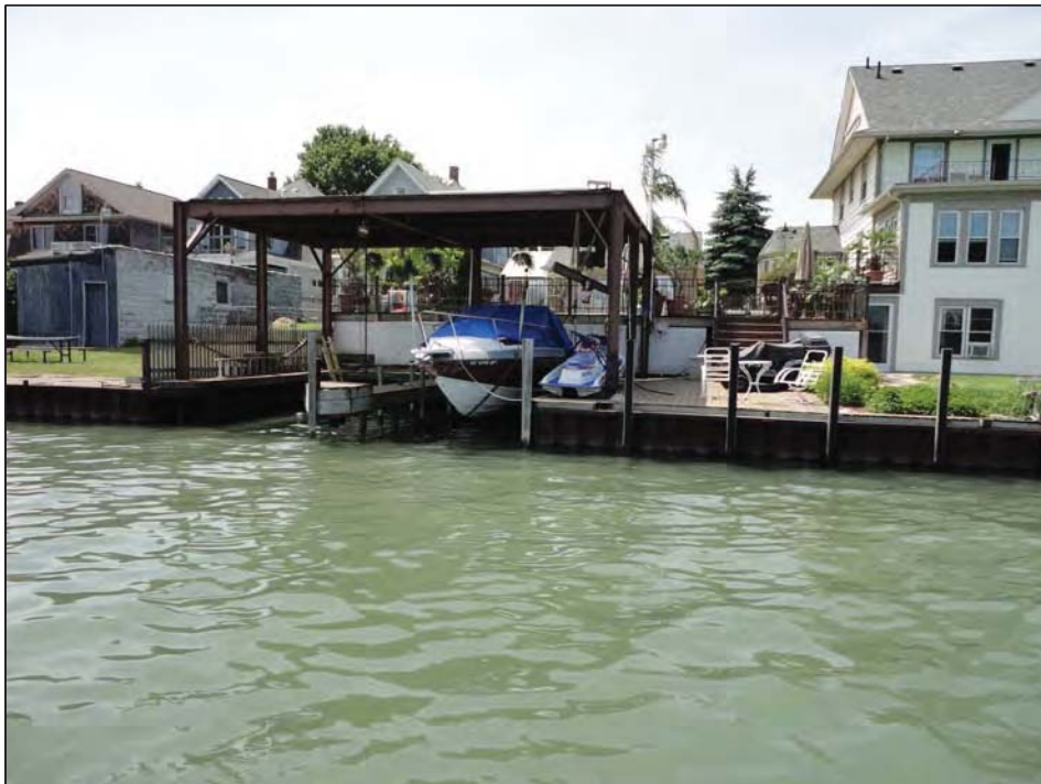
Steel Sheetpile with boatslip
