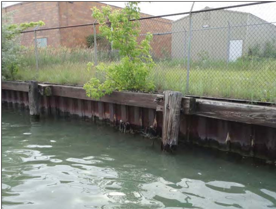
Steel sheetpile with wood pilings in front
