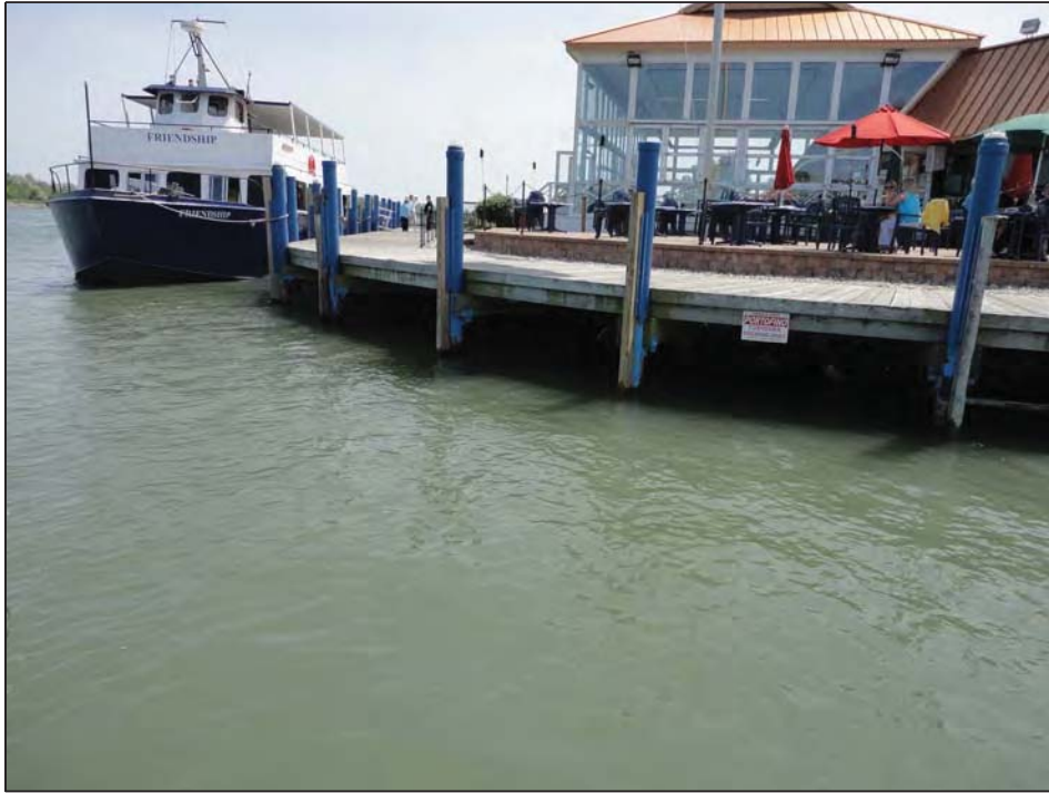
Wood dock on steel piles over rip rap
