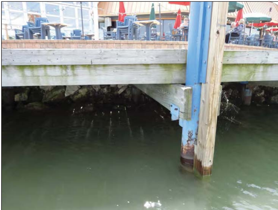
Wood dock on steel piles over rip rap
