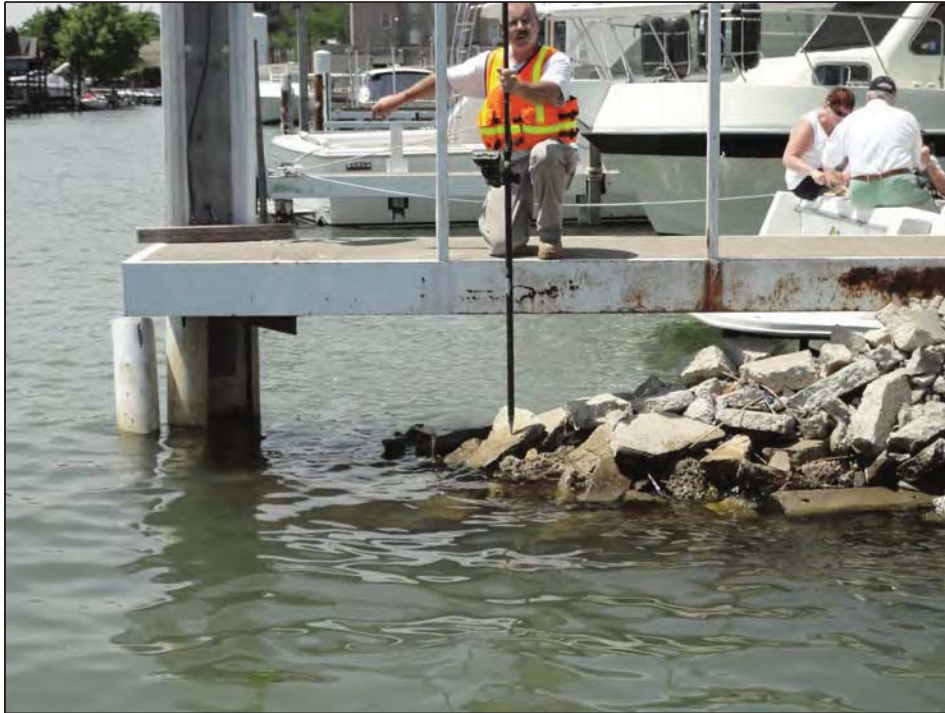
Broken Concrete Rip Rap with concrete boat dock on steel piles
