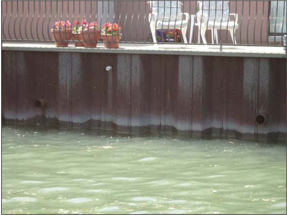
Steel Sheetpile with three outfalls (two steel, about 6" and one PVC, about 1")
