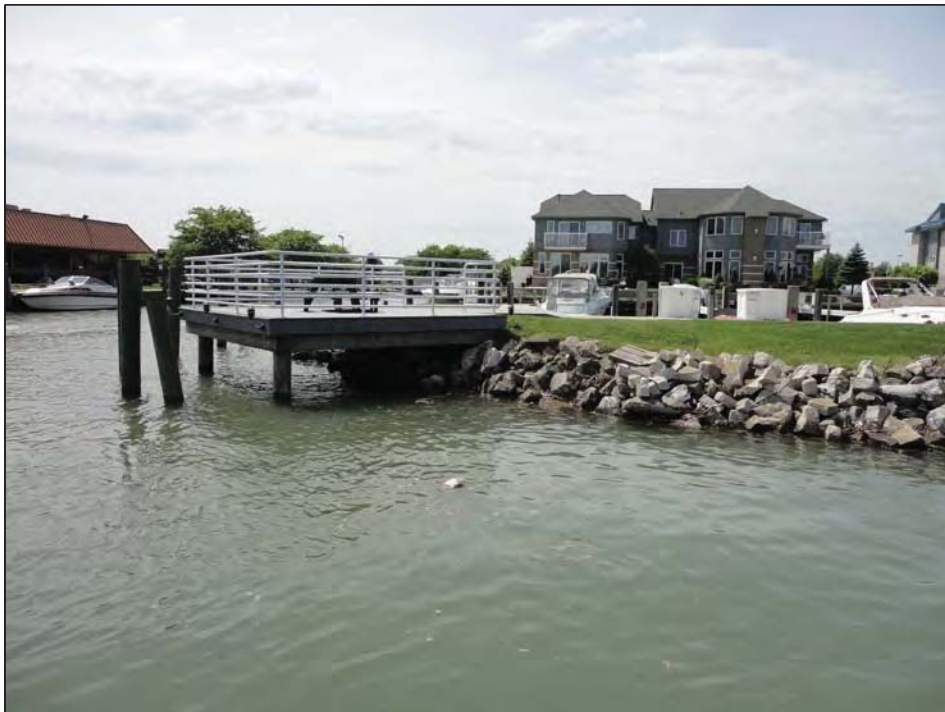
Rip Rap with deck on wood piles extending from berm around condo marina
