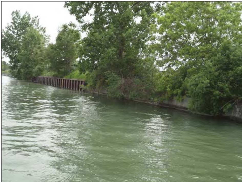
Concrete and steel sheetpile
