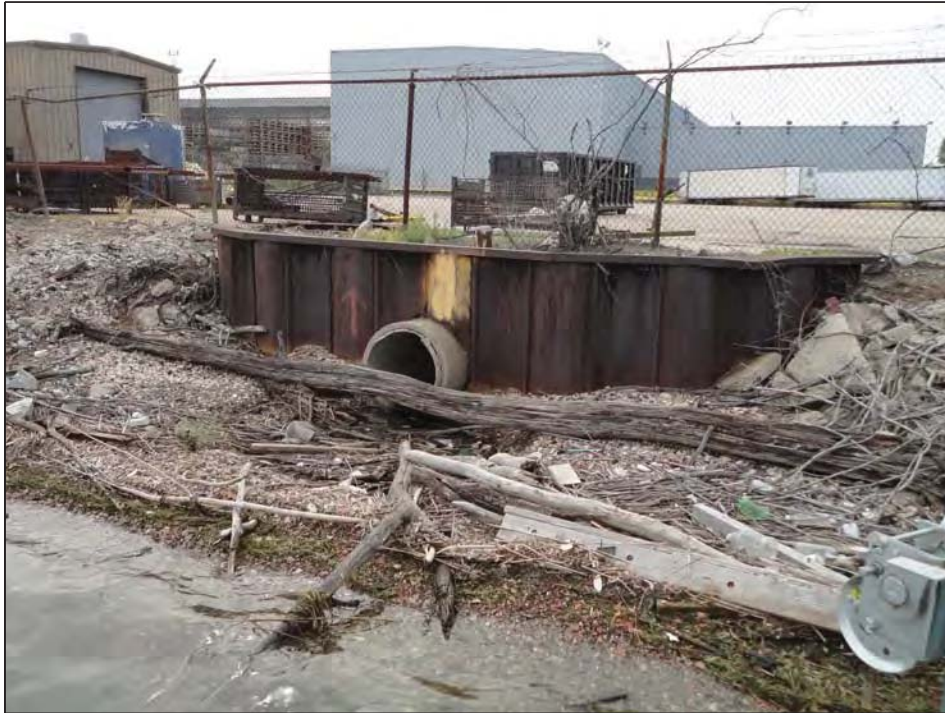
Construction debris and some large concrete pieces with concrete outfall (about 24") surrounded by steel sheetpile
