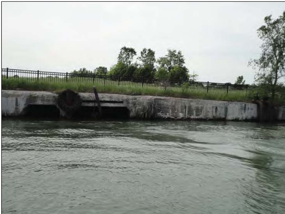
Concrete with box sewer and large pipes
