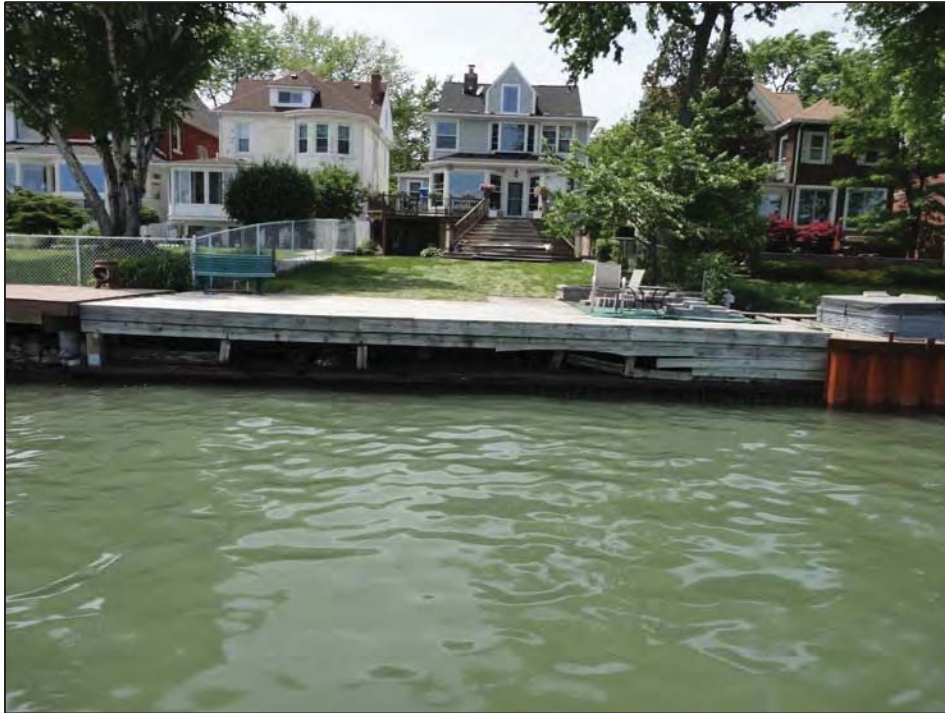
Wood over Steel Sheetpile
