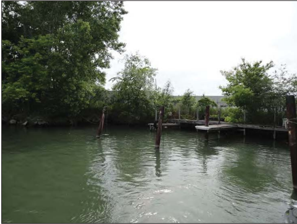
Concrete pieces/debris with dock structure – wood with steel piles
