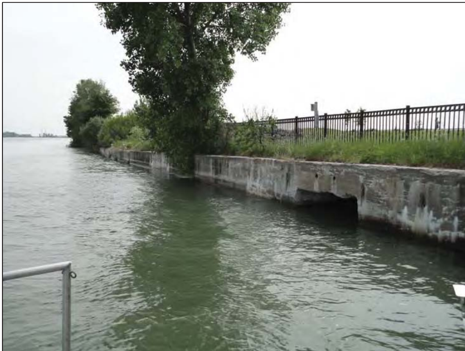
Concrete with concrete box sewer
