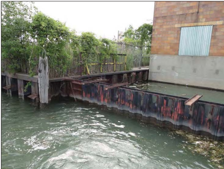
Steel sheetpile with wood pilings in front and old boat inlet with building
