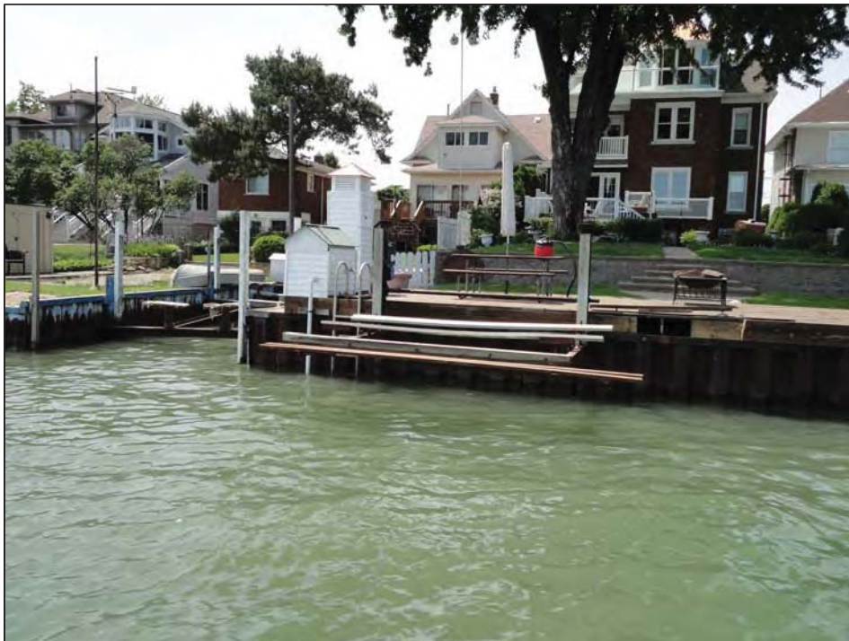
Steel Sheetpile with boatslip
