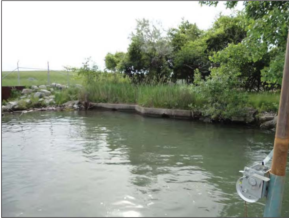
Concrete pieces/debris with two concrete outfalls surrounded by concrete wall
