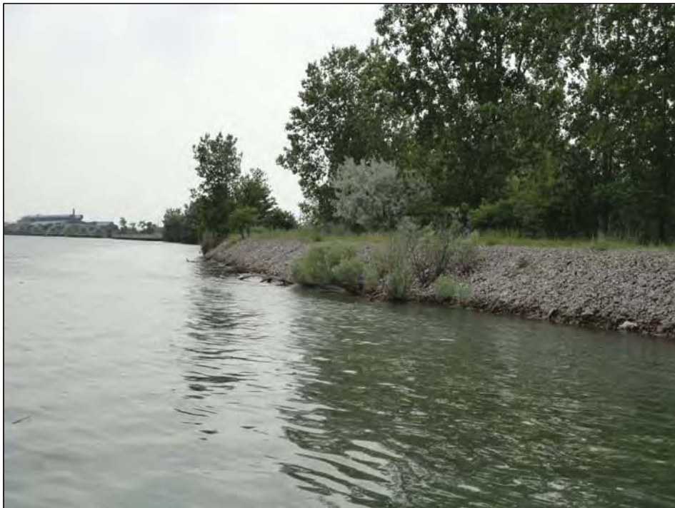
Construction debris rip rap with vegetation
