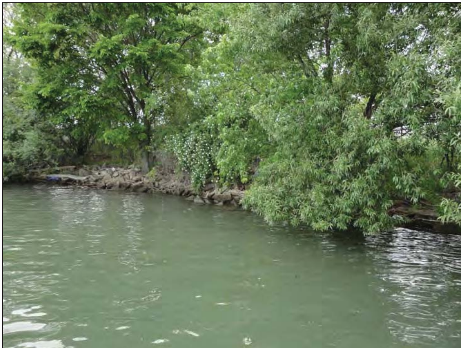
Construction debris rip rap with vegetation
