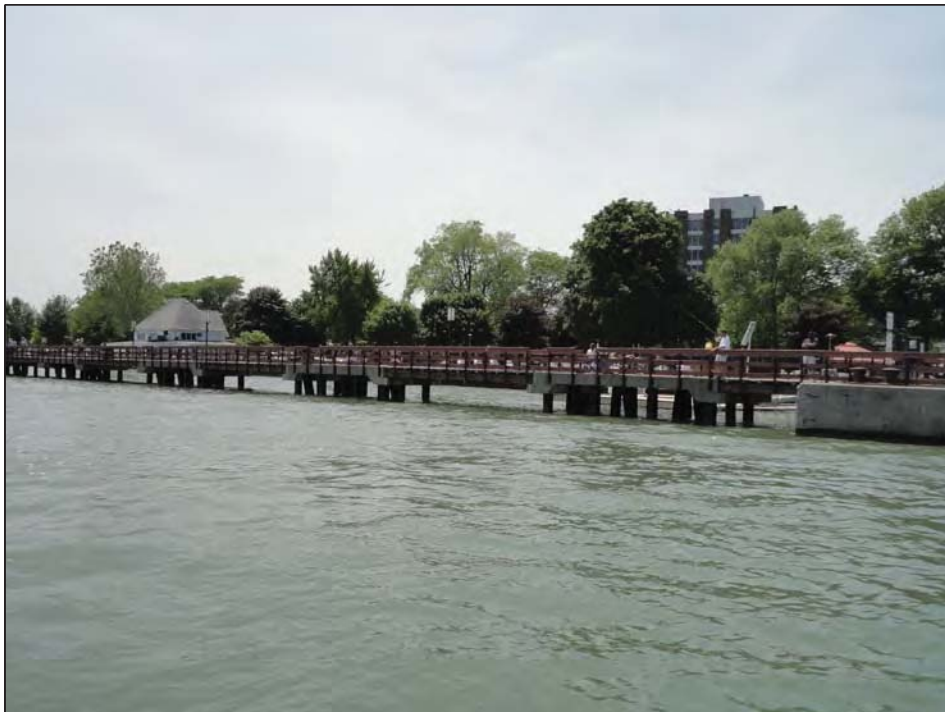
Concrete with fishing pier on steel piles
