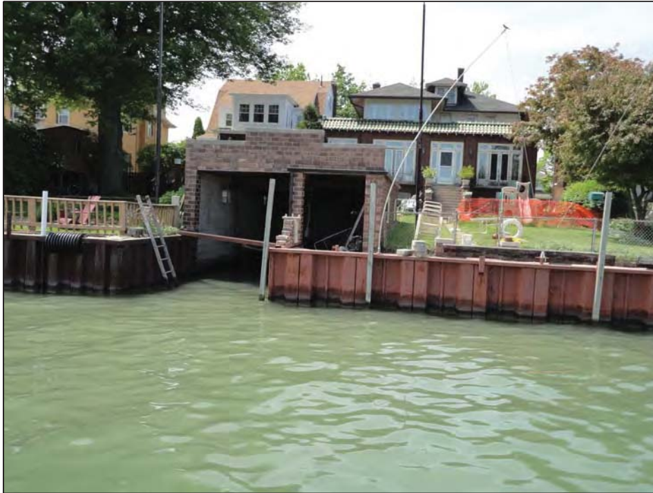
Steel Sheetpile with brick boat house
