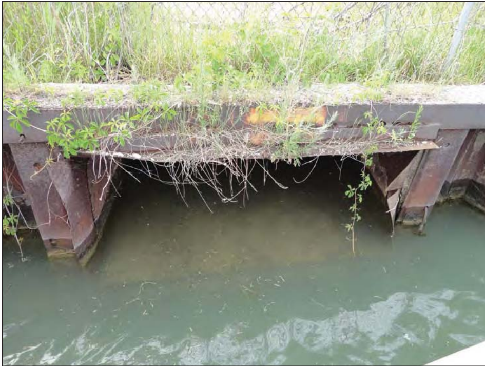
Steel sheetpile with steel box sewer and wood pilings in front
