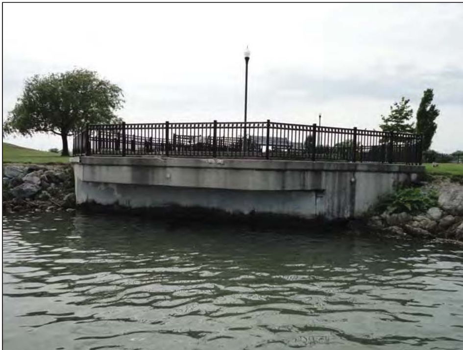
Rip Rap with concrete seating area – overhanging on concrete base
