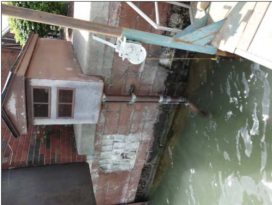
Concrete block and intake with pump house (about 1" and 3" copper pipes)
