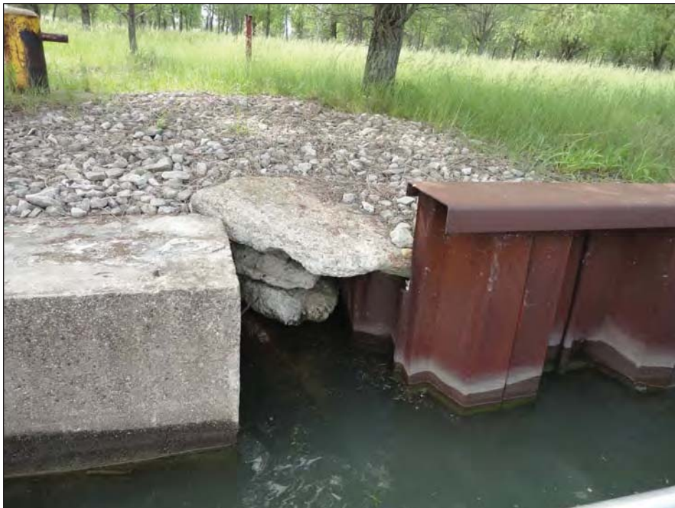
Gap at joint of concrete and steel sheetpile
