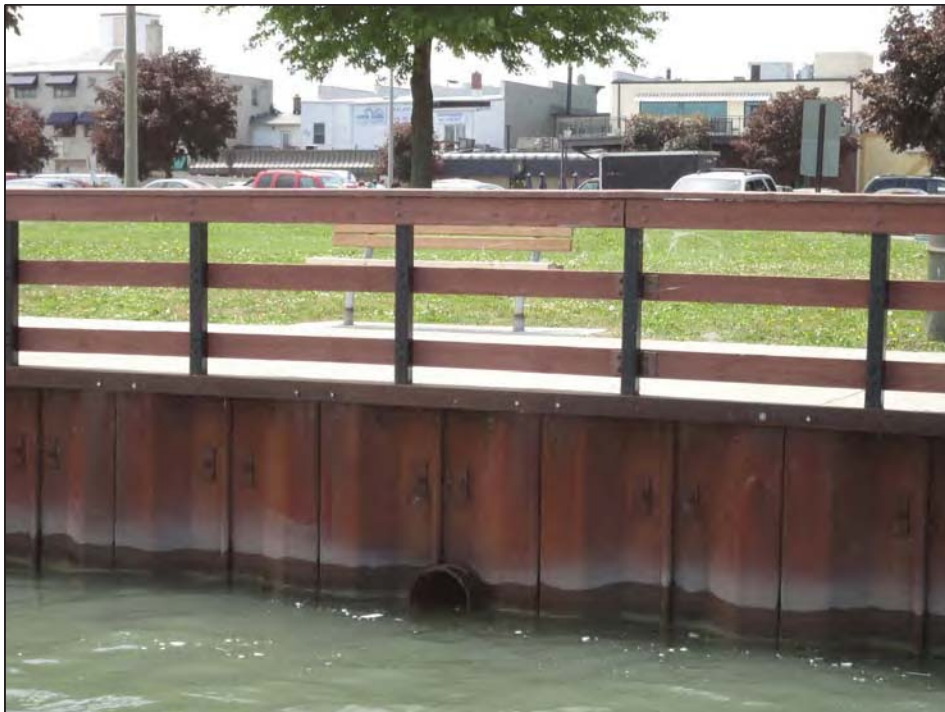
Steel Sheetpile with steel outfall pipe (about 12")
