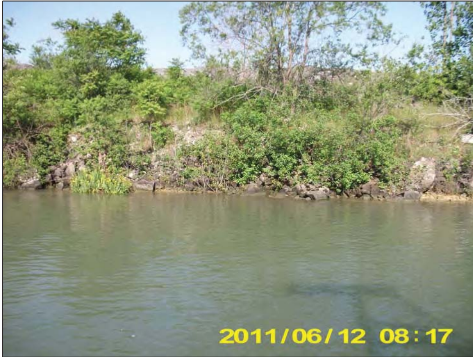
Rip Rap with vegetation
