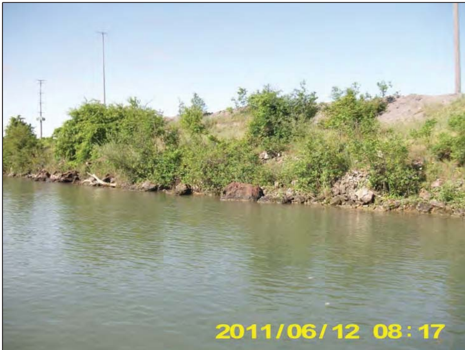
Rip Rap with vegetation
