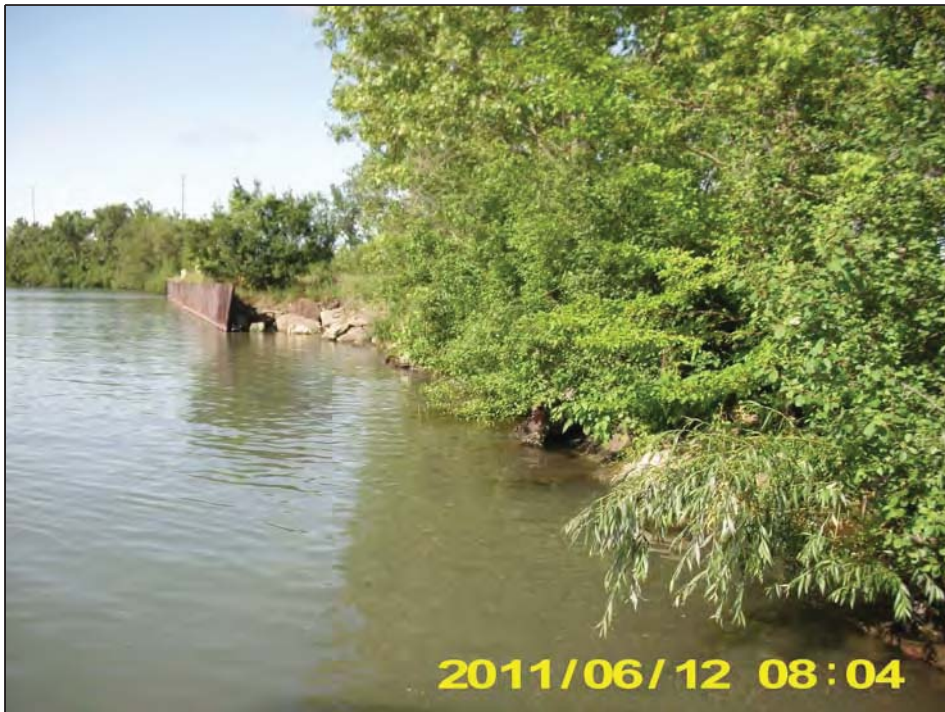
Rip Rap and steel sheetpile with vegetation
