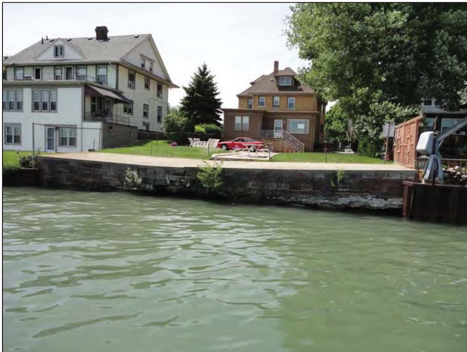
Concrete/block (failing)
