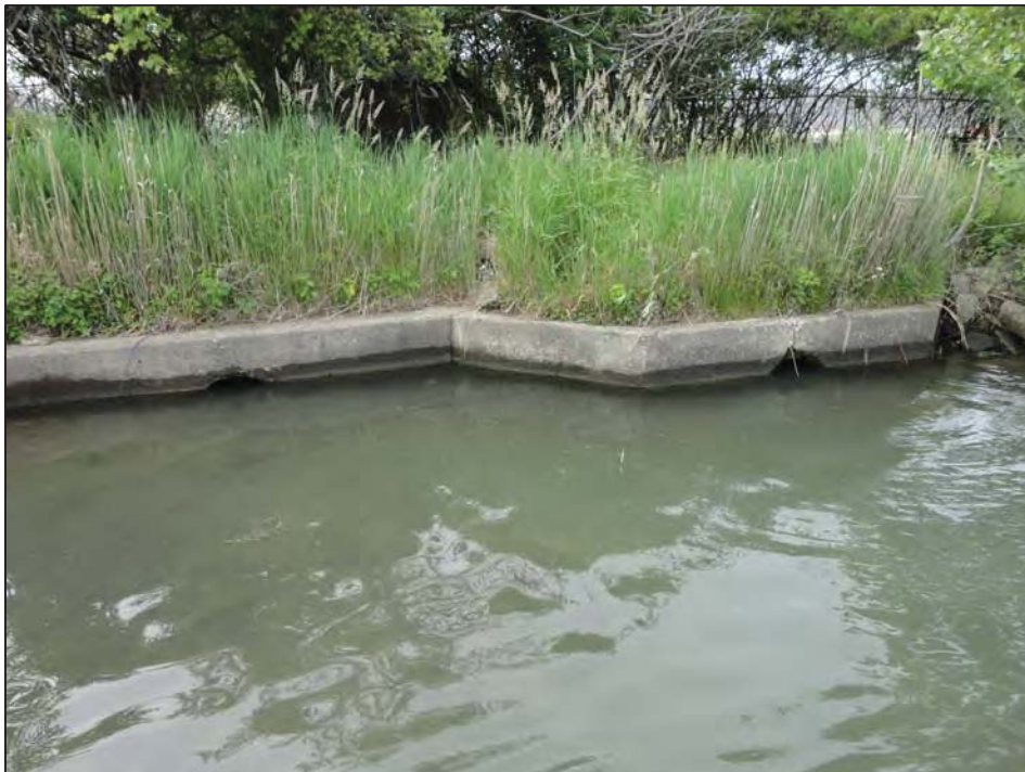
Concrete pieces/debris with two concrete outfalls surrounded by concrete wall
