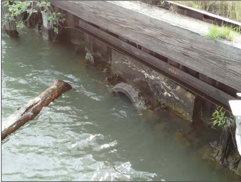
Steel sheetpile with concrete outfall (about 24") and wood pilings in front
