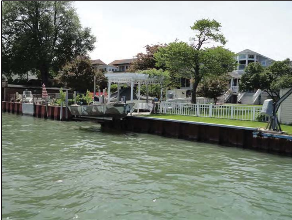
Steel Sheetpile with boatslip
