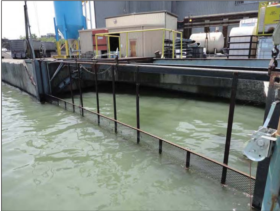
Concrete and water intake with screened metal gate
