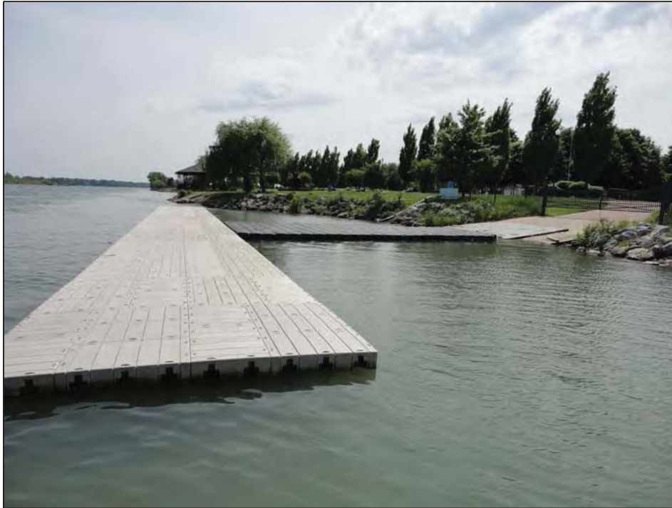
Rip Rap and concrete boat ramp with floating platform
