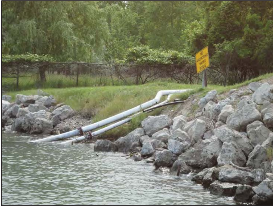
Rip Rap with water intake lines and pump for golf course (PVC, about 4" and 6")
