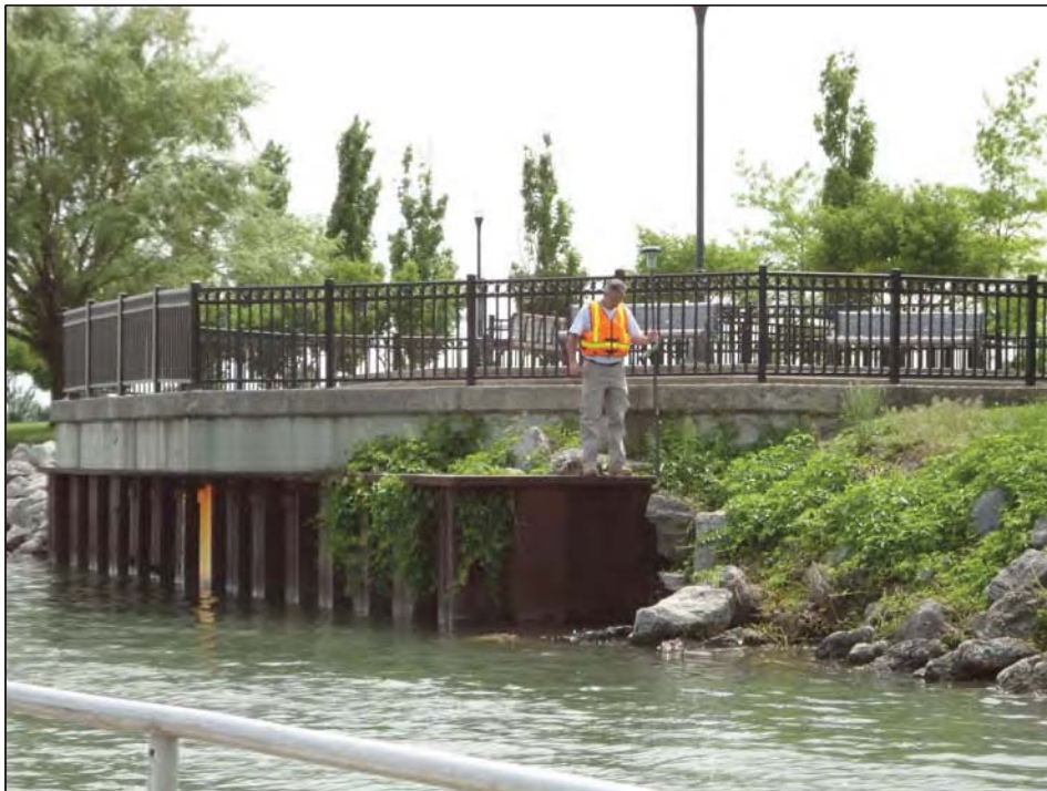
Rip Rap and steel sheetpile with overhanging concrete seating area
