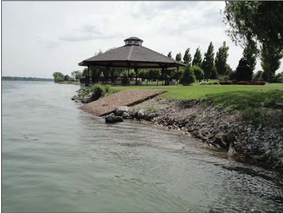
Rip Rap with geotextile fabric visible
