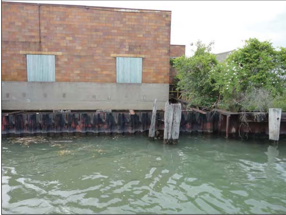
Steel sheetpile with wood pilings in front and old boat inlet with building
