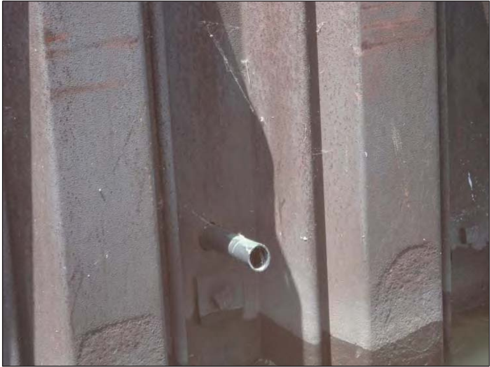
Steel Sheetpile with 2" possible outfall
