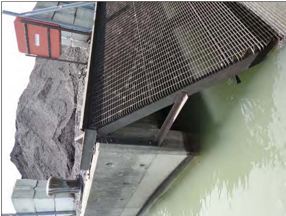
Concrete with screen and space under concrete dock
