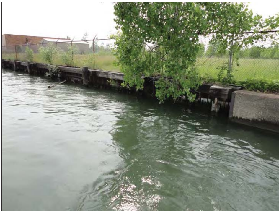
Steel sheetpile with wood pilings in front
