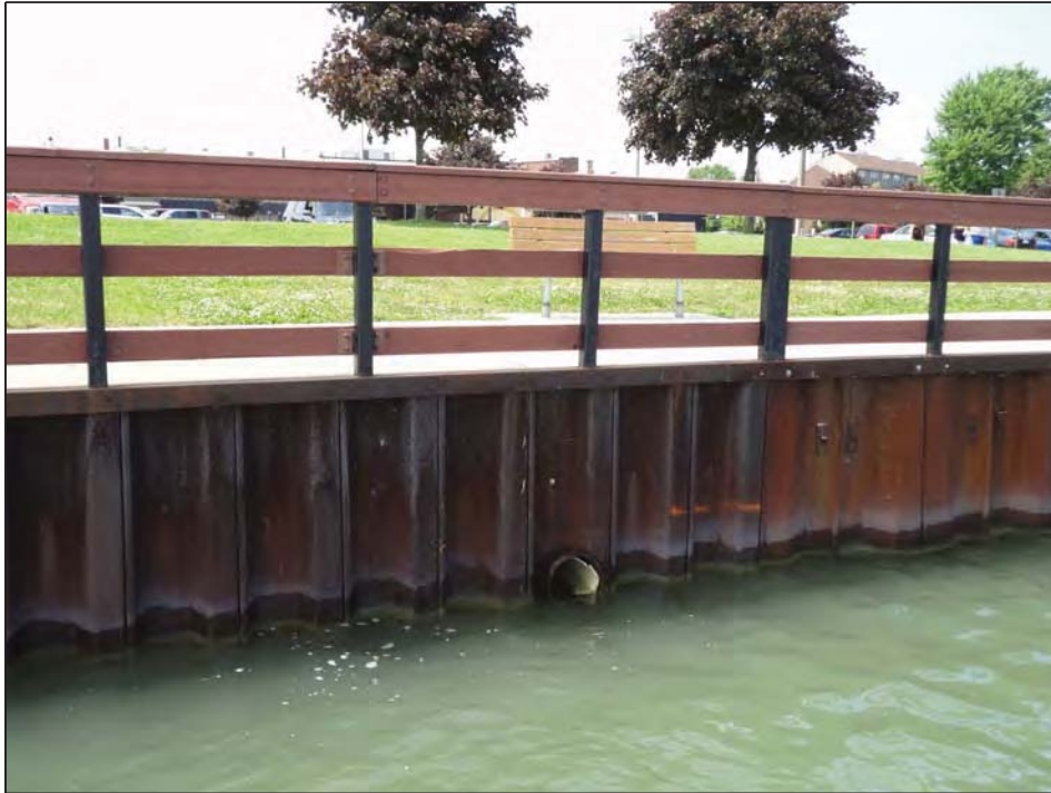
Steel Sheetpile with outfall pipe (about 12", steel lined with PVC)
