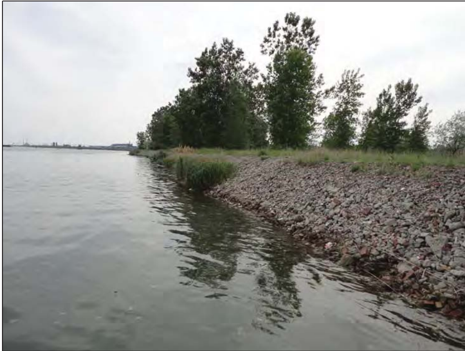
Construction debris rip rap with vegetation
