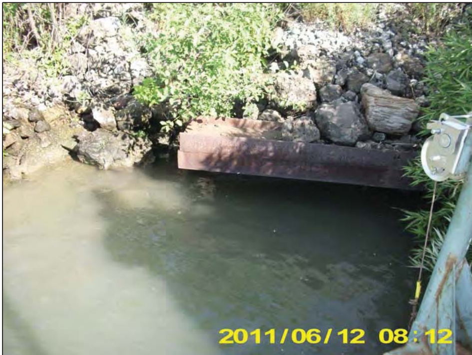
Low Steel Sheetpile with rip rap and vegetation
