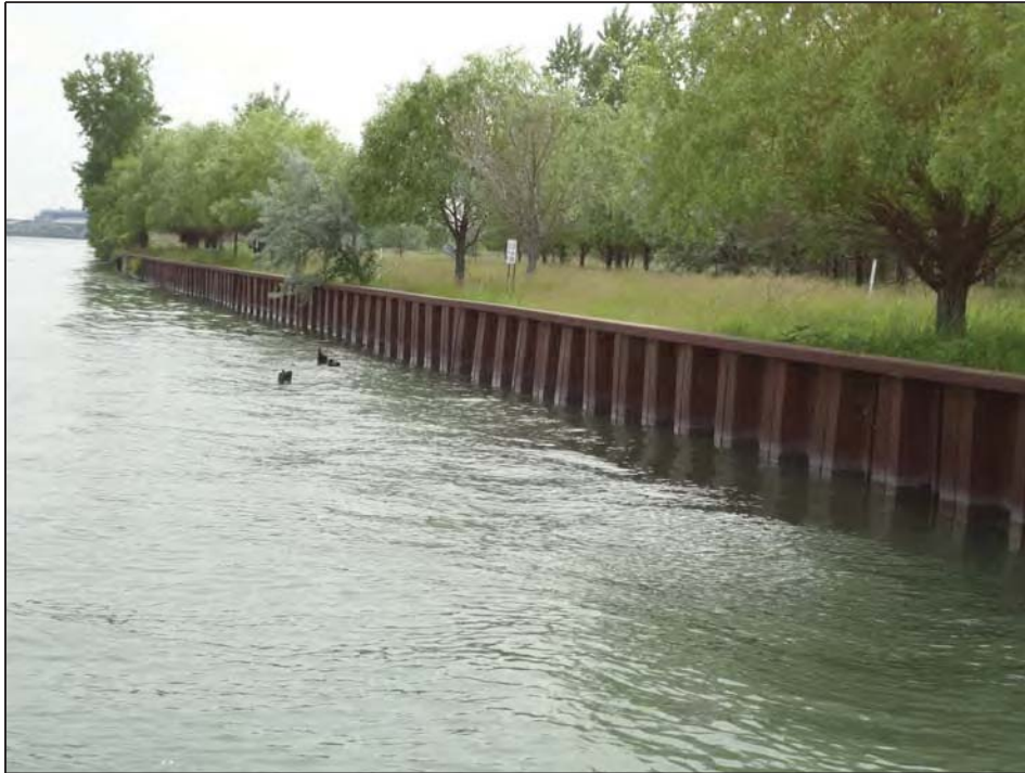
Steel Sheetpile with wooden piles
