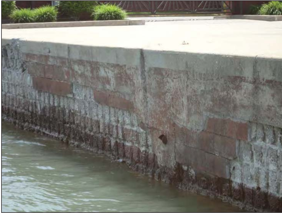
Concrete block with outfall (broken end, about 6", steel)
