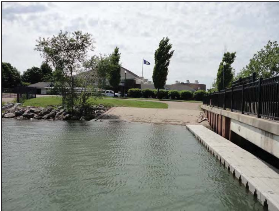
Rip Rap and concrete boat ramp
