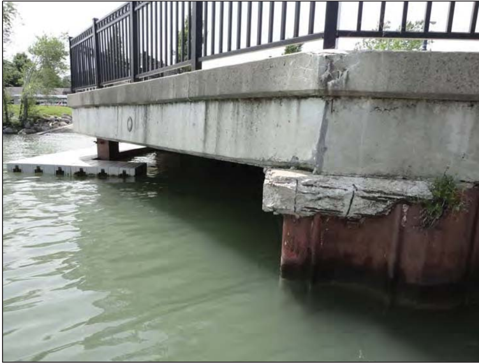
Rip Rap with octagonal concrete seating area overhanging on steel piles (sides) and concrete with steel sheetpile (front)
