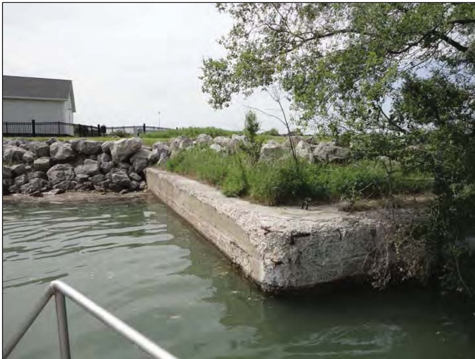
Concrete and Rip Rap
