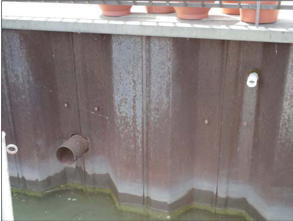
Steel Sheetpile with outfalls (about 1", PVC and about 6", steel)
