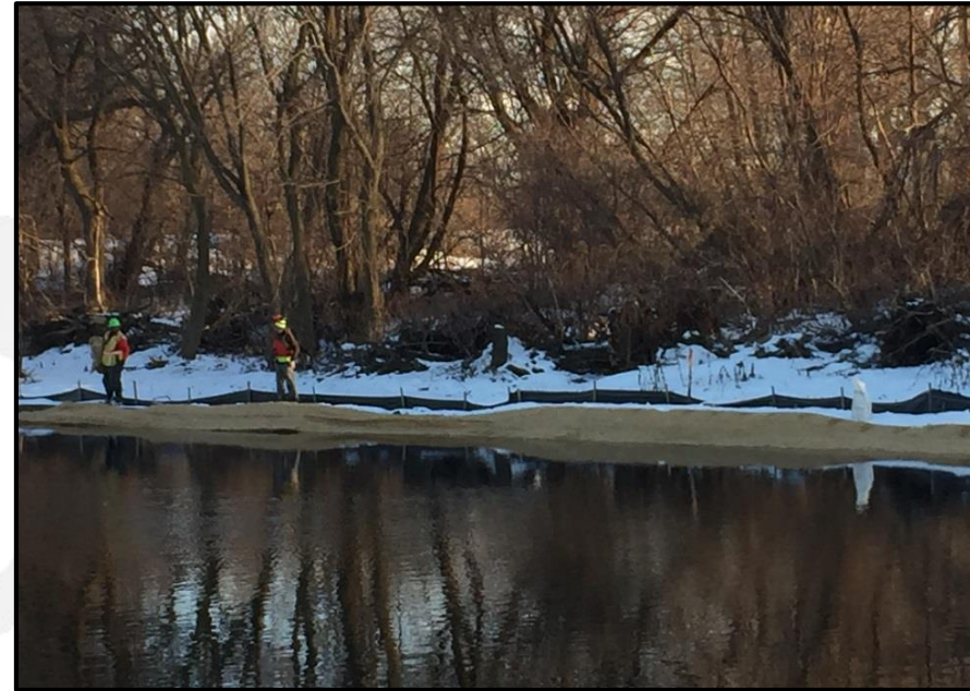
Seeding and placing erosion mats
