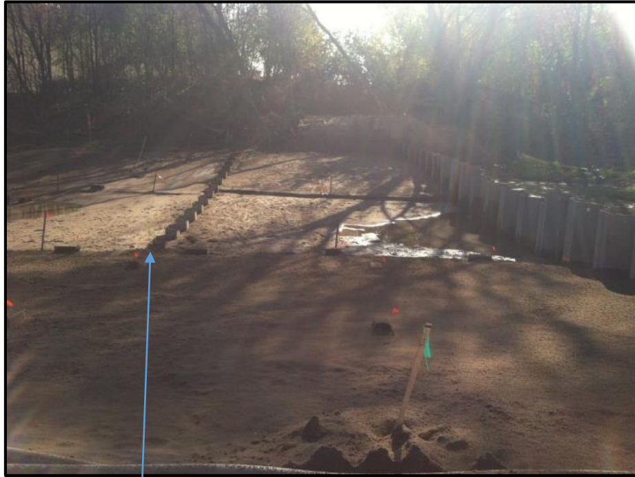
Existing sheet pile
