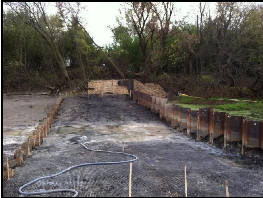
Completing capping at state line boundary
