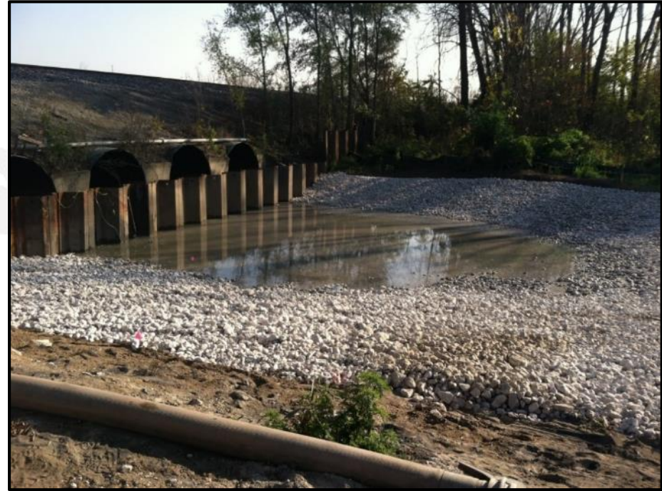
Scour protection west of railroad culverts
