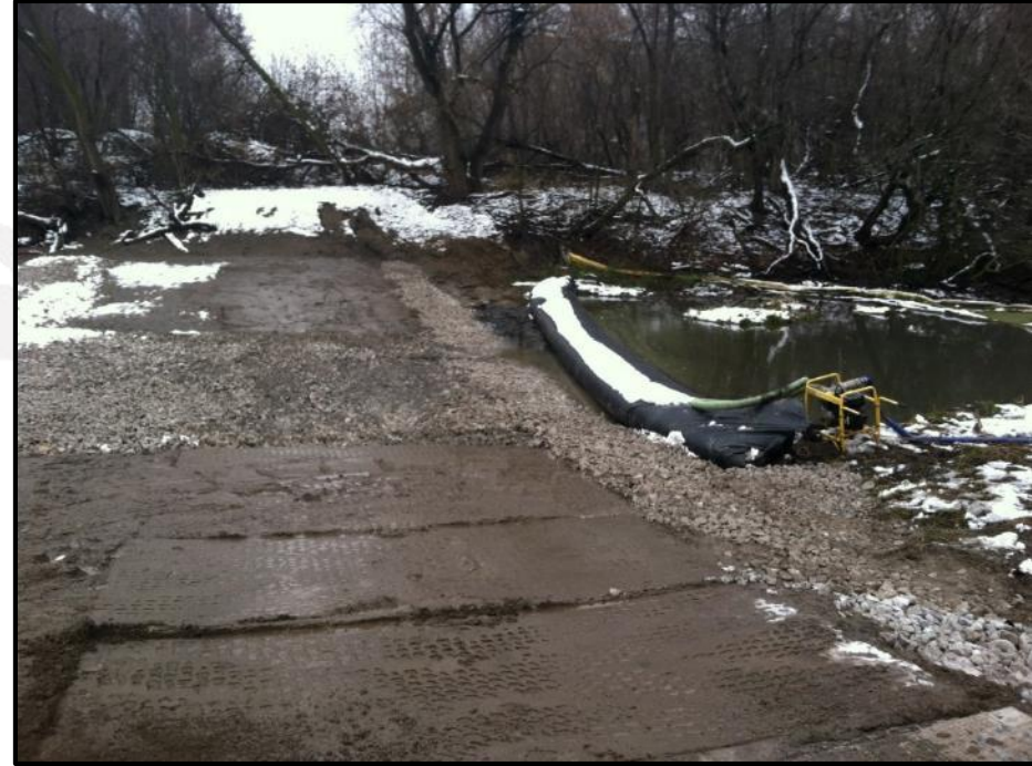
Sheet pile covered with stone
