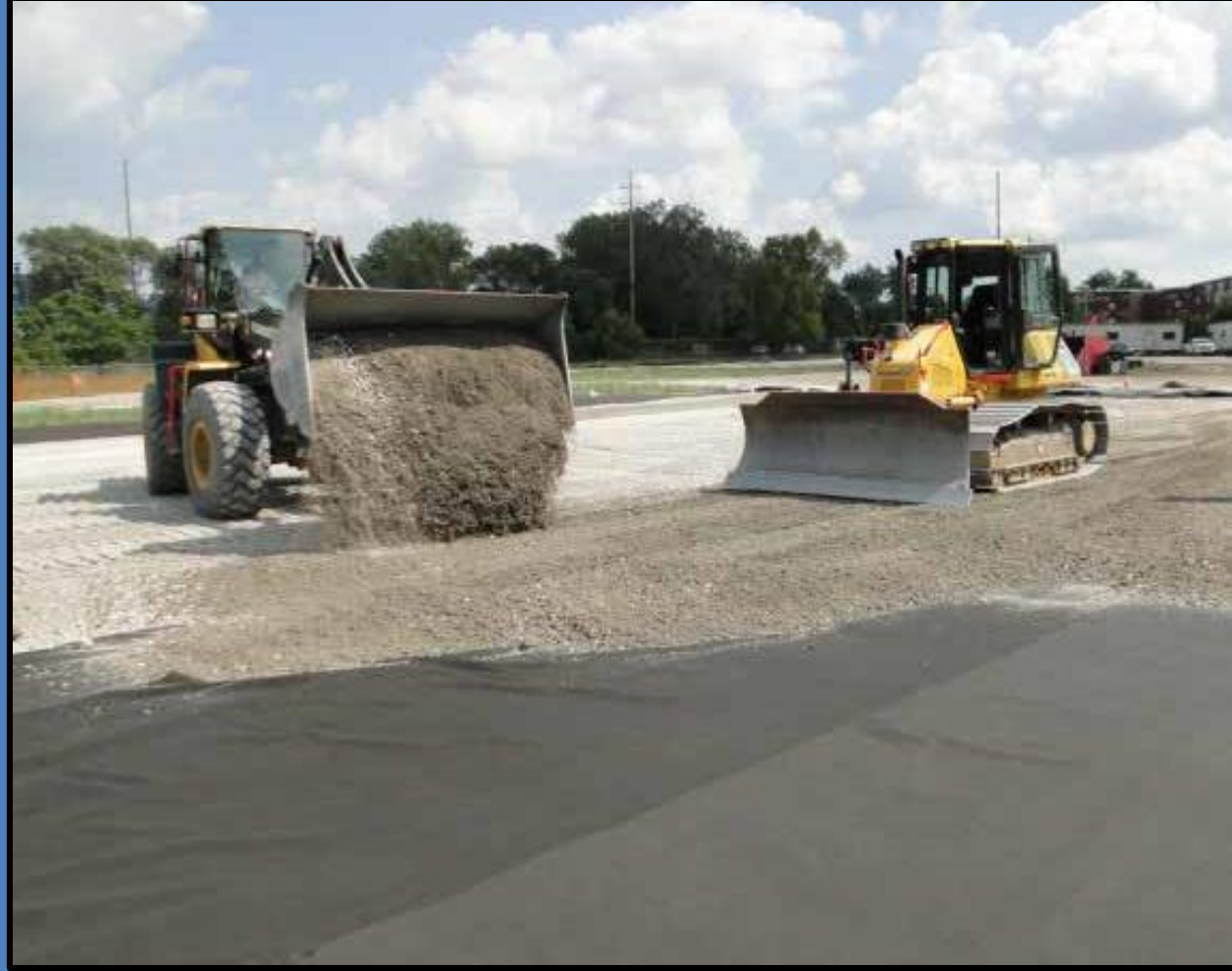
Install sediment processing pad
