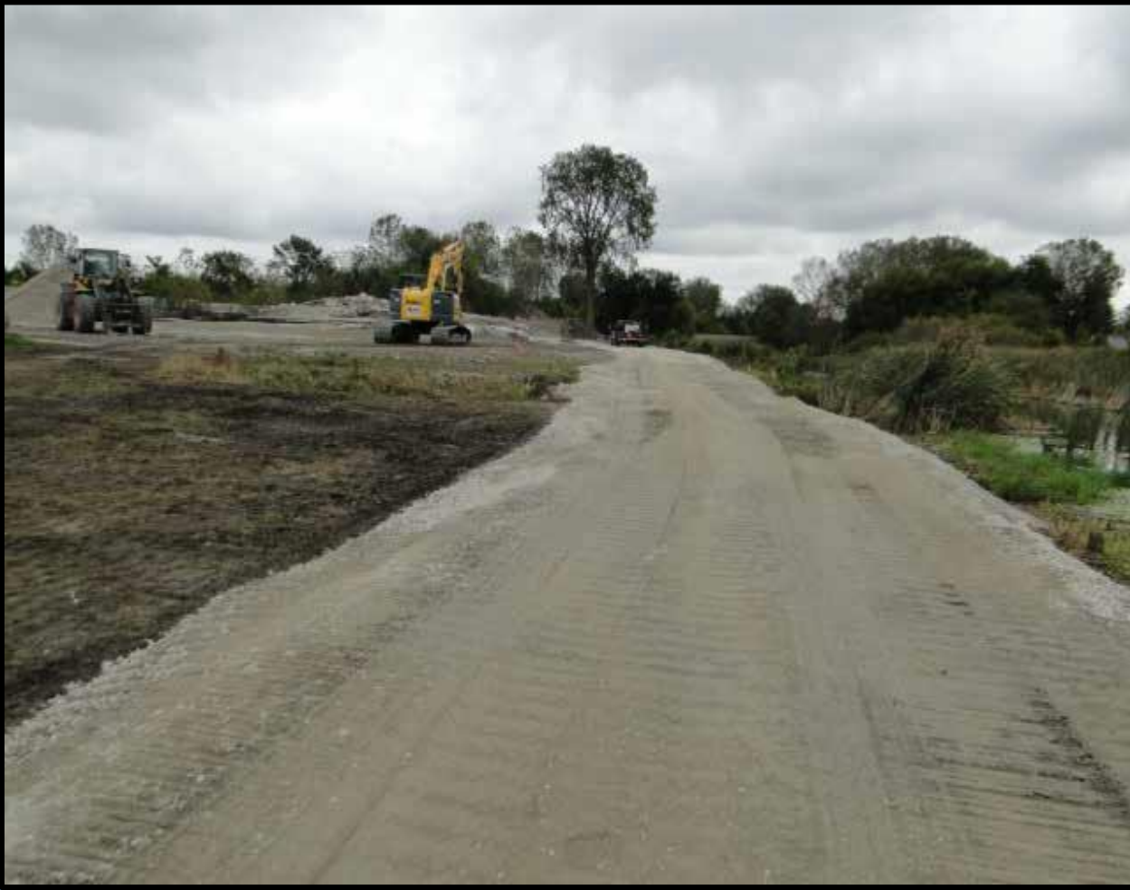
Install temporary roads
