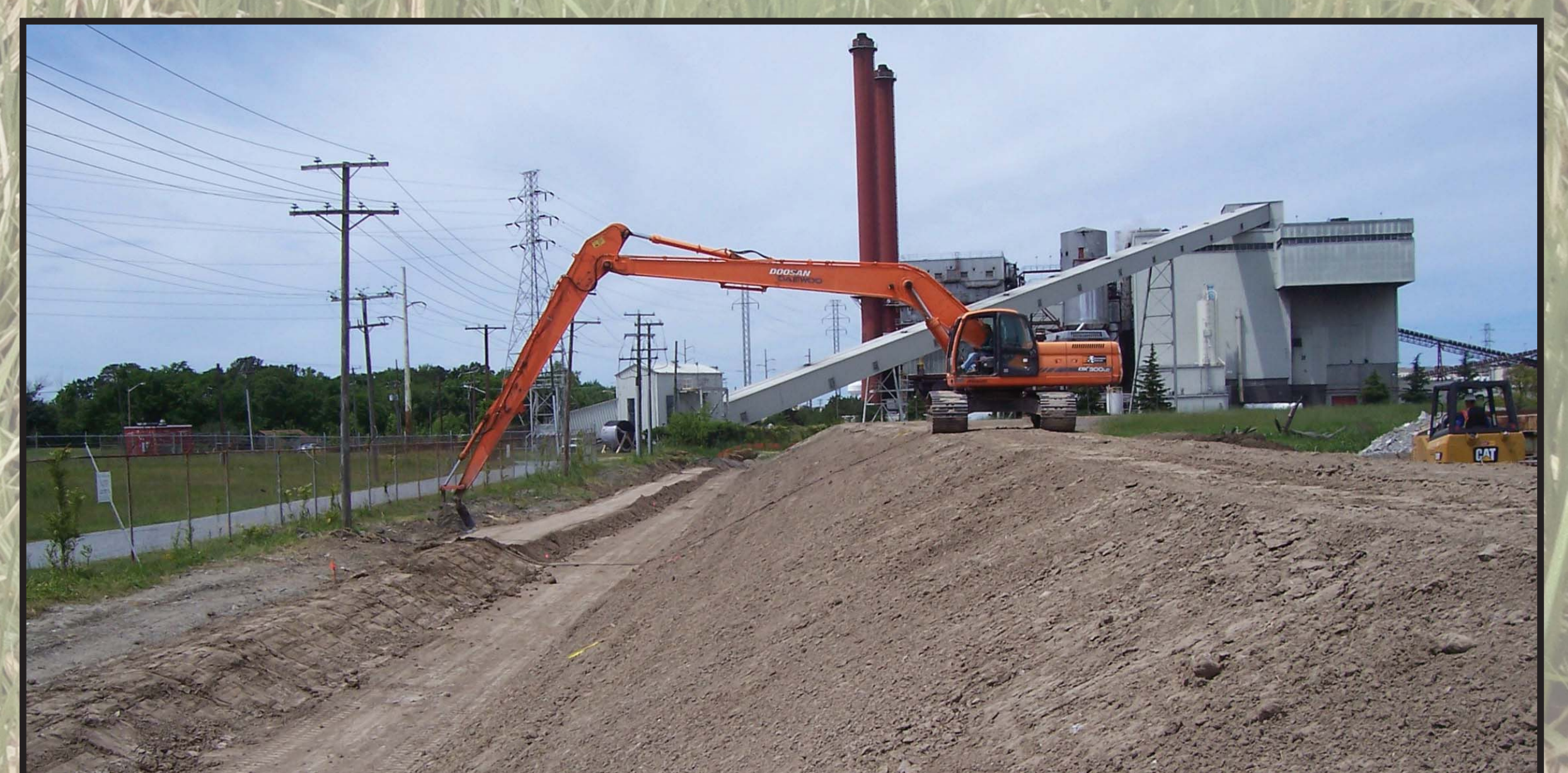
Berm construction
