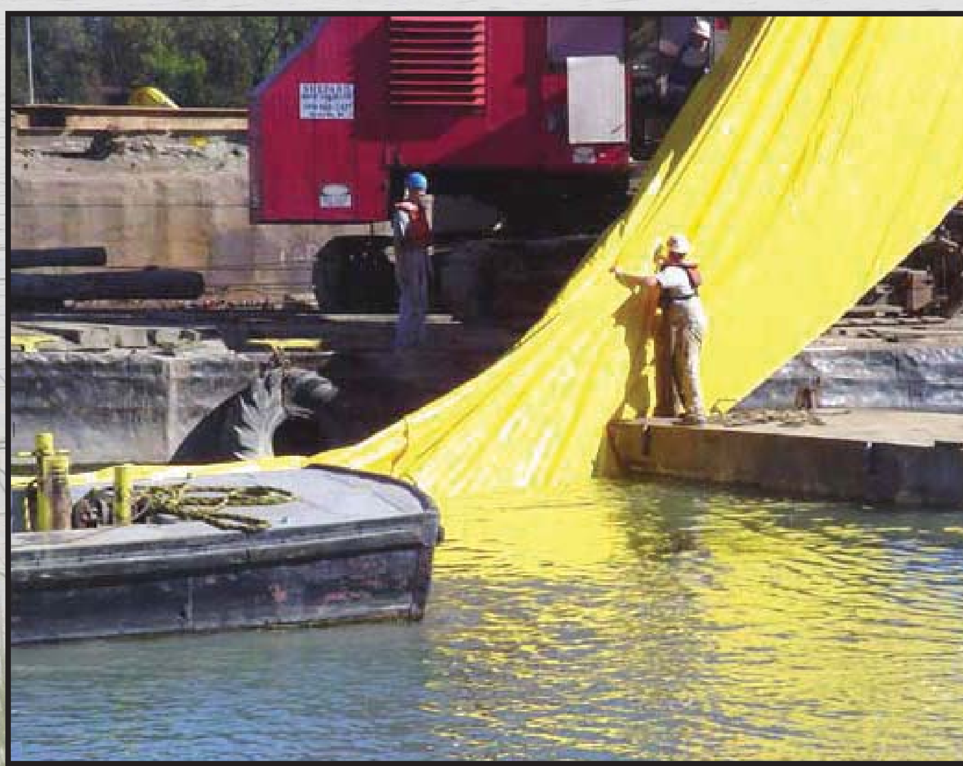
Installation of silt curtain
