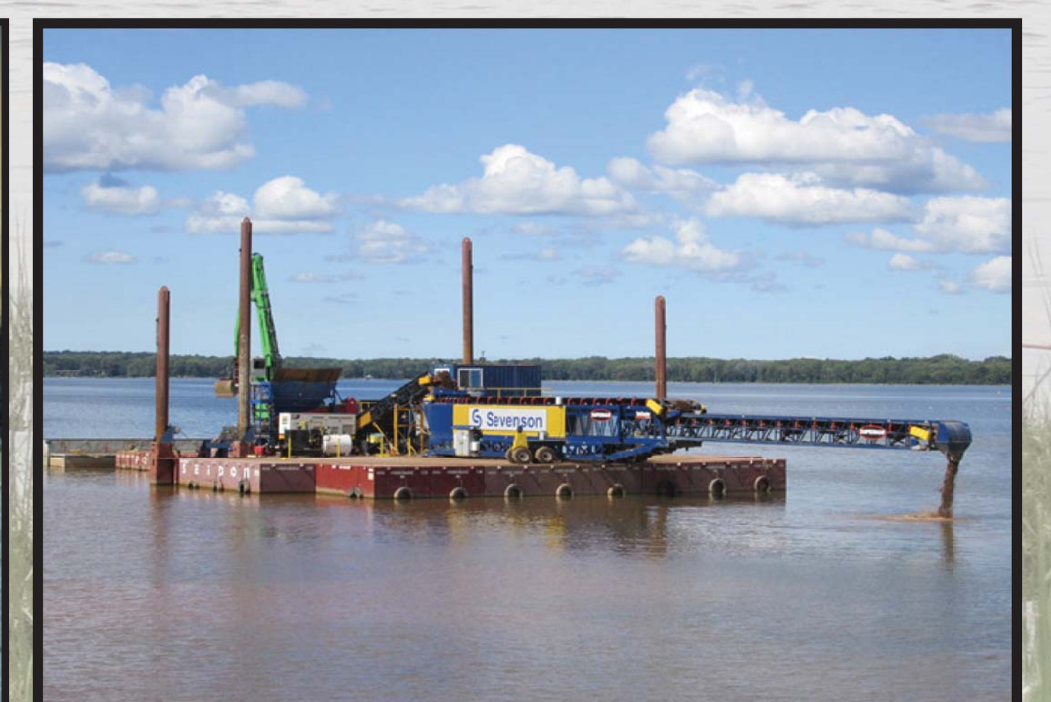
EMNR Cover Construction
