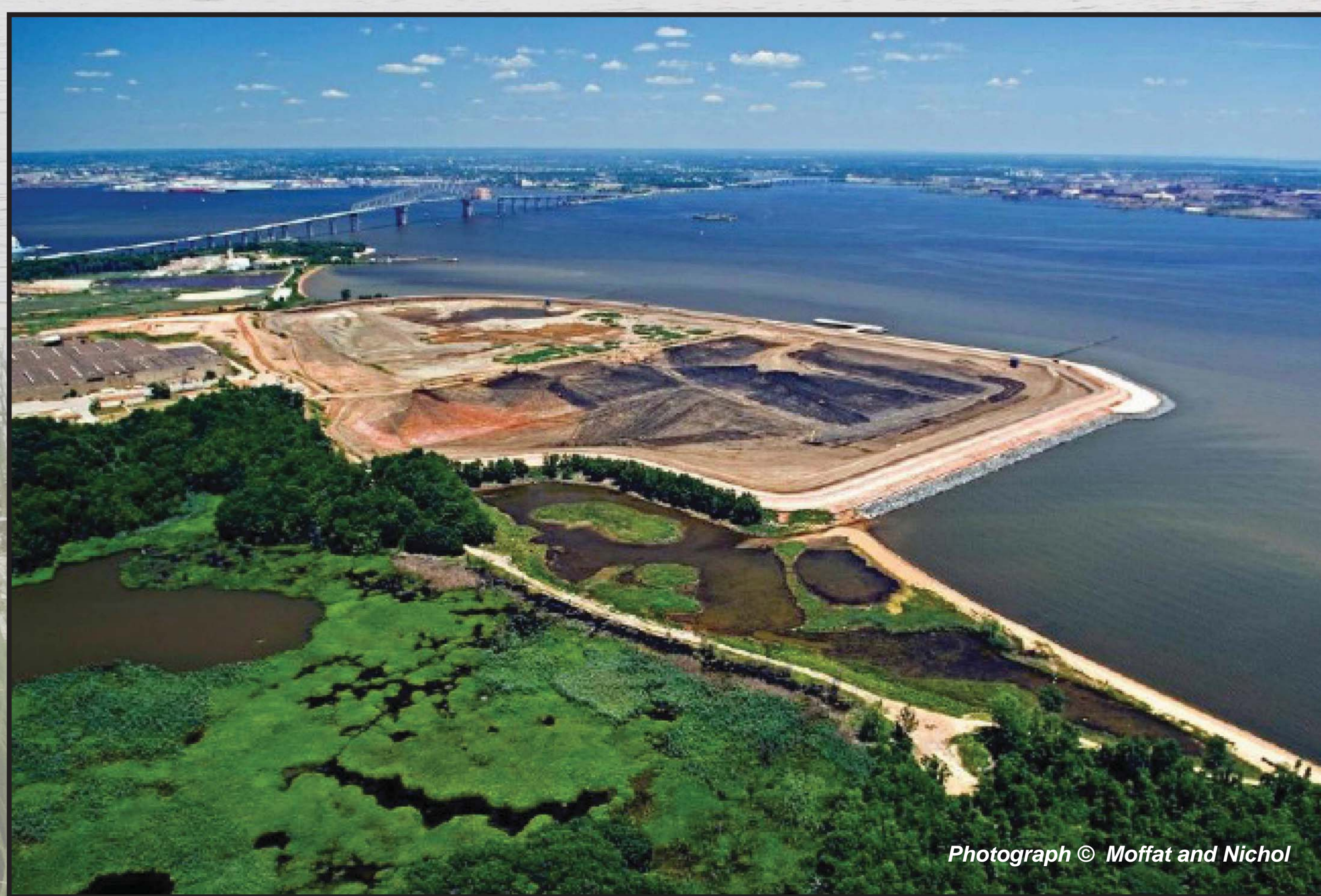
Cox Creek Dredged Material Containment Facility (CDF)
