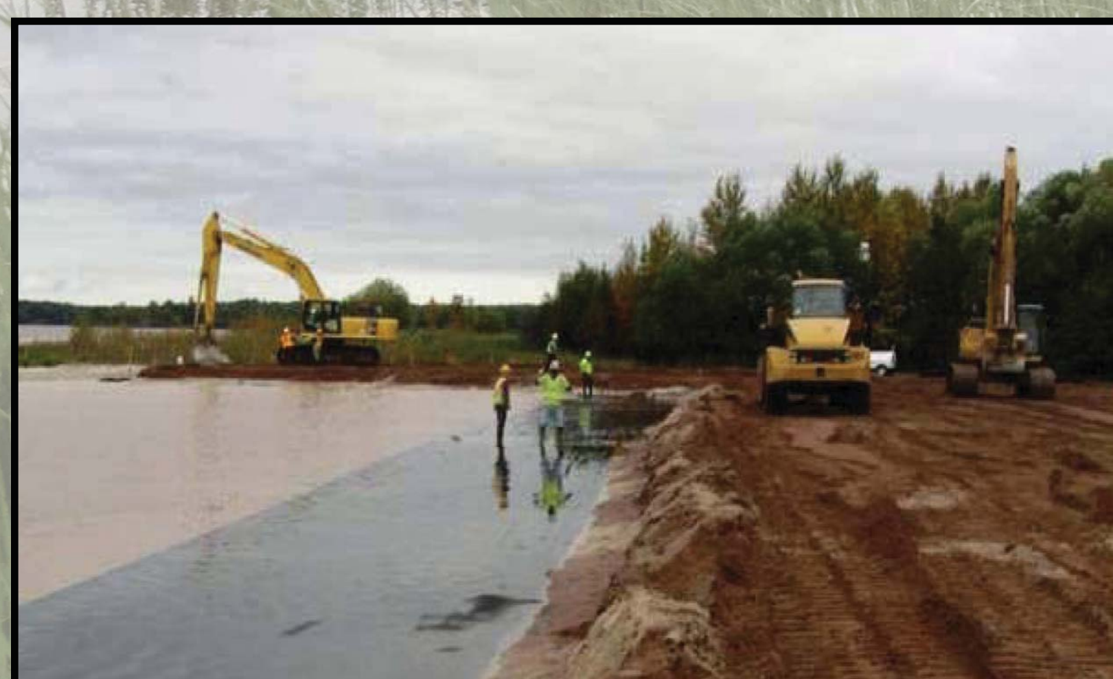
Installing root barrier in cap
