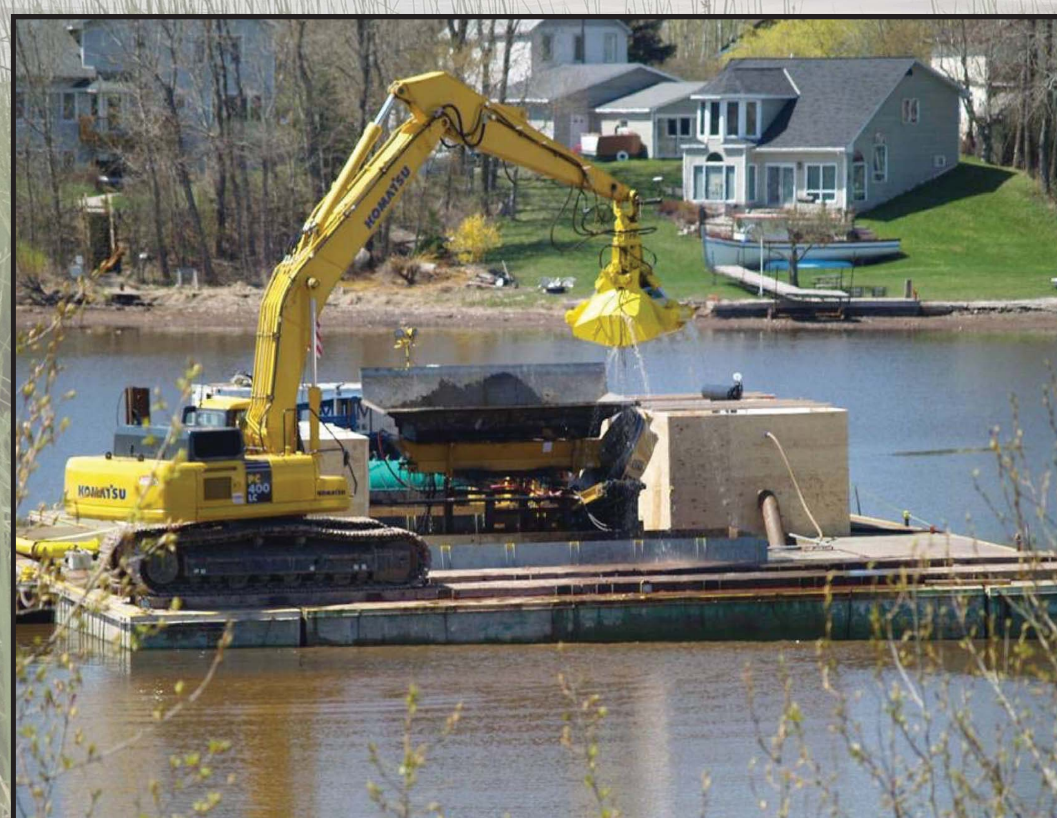
Excavator with environmental bucket
