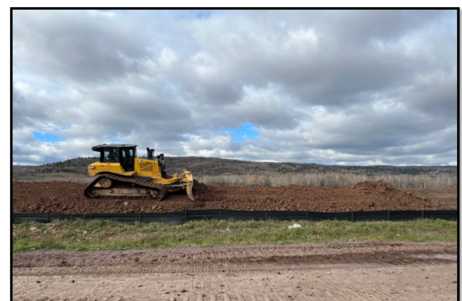
Berm construction for the OU-J CDF at Spirit Lake.
