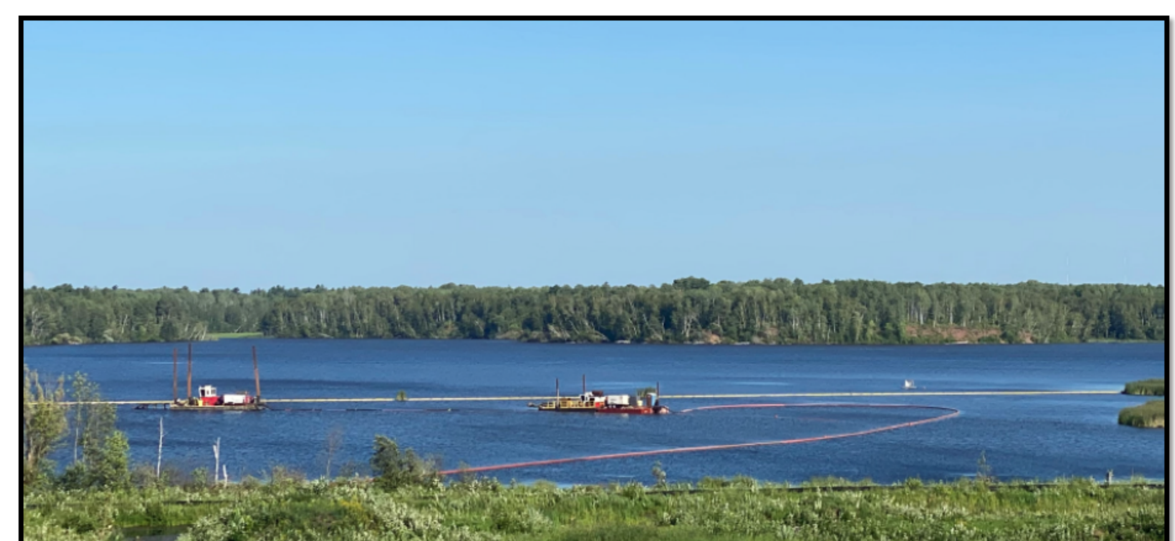
Turbidity curtains deployed during hydraulic dredging in Wire Mill Delta.
