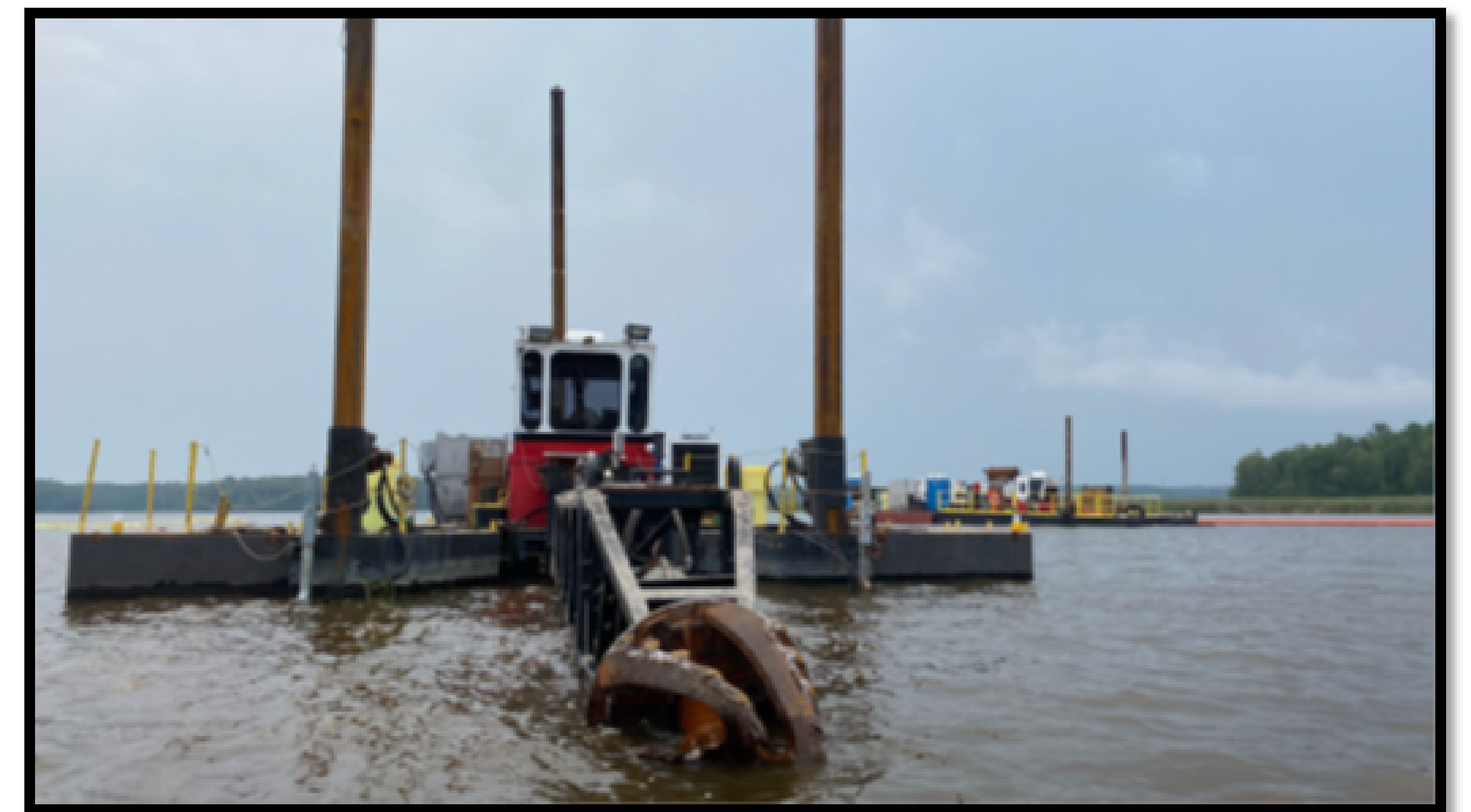
Dredging is conducted with a hydraulic cutterhead dredge in the Wire Mill Delta.
