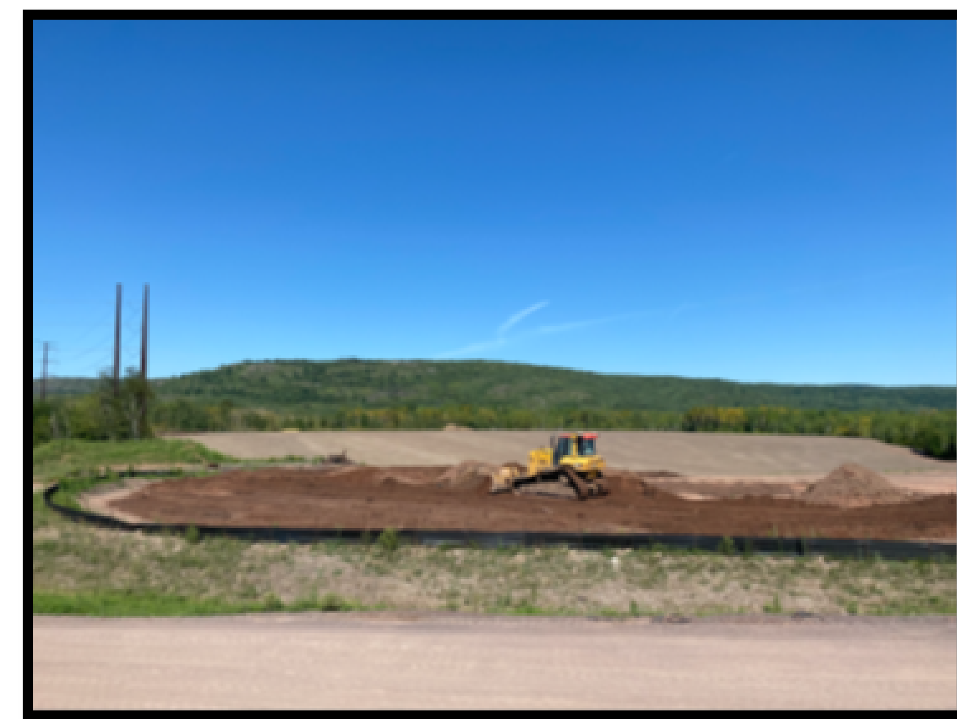
Processed material is placed directly in the OU-J CDF.
