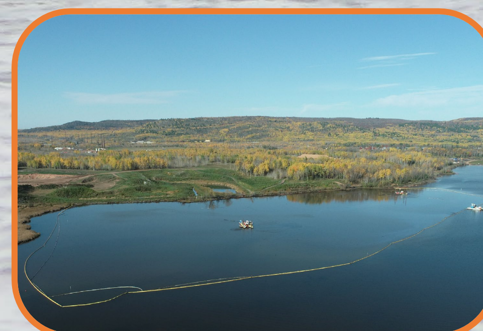
Wire Mill Delta Dredging
