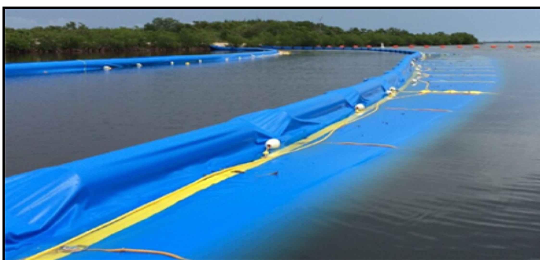
Conceptual example of a typical silt curtain.
