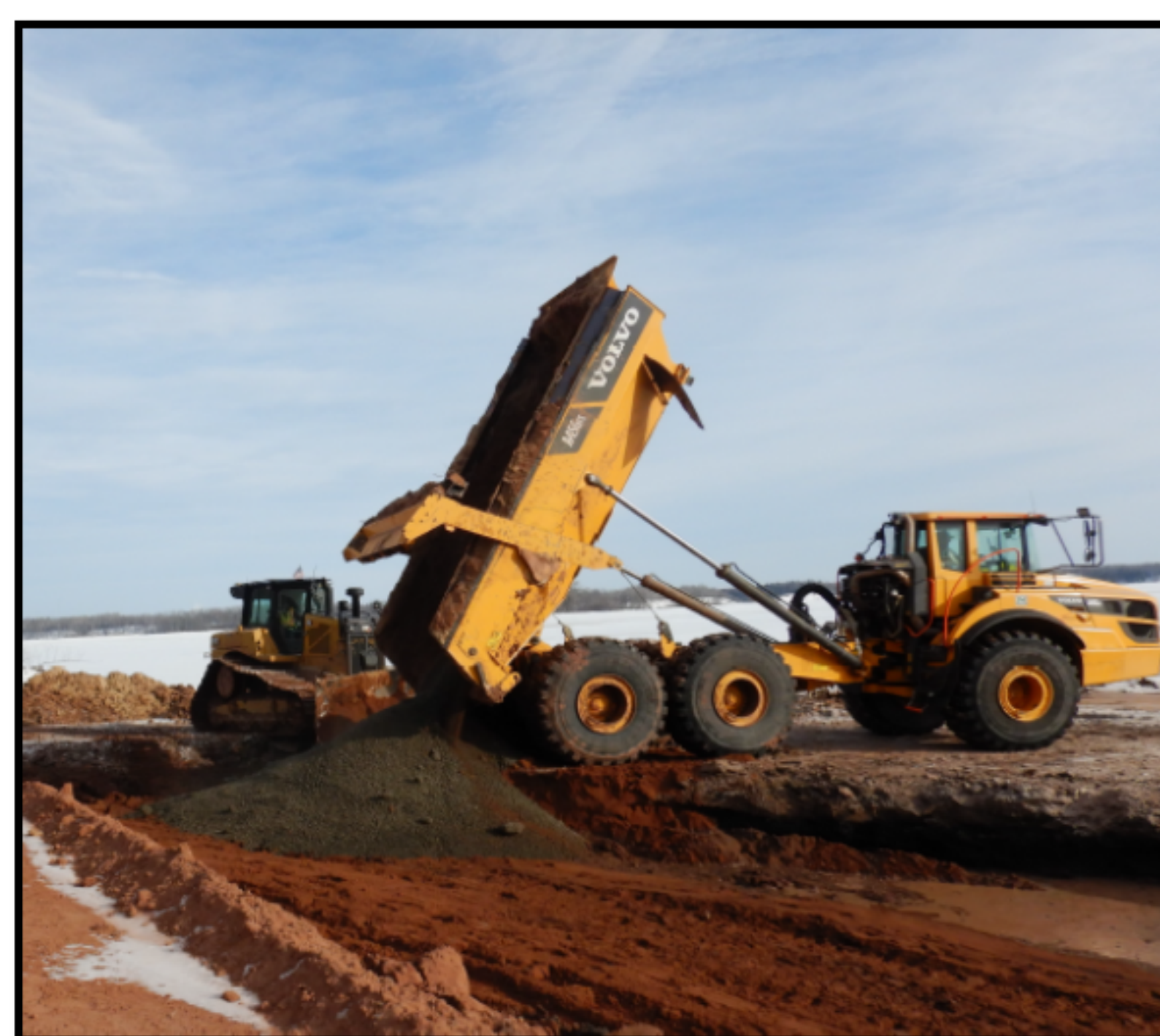
Root barrier being installed in a cap in the Shallow Sheltered Bay Spirit Lake.
