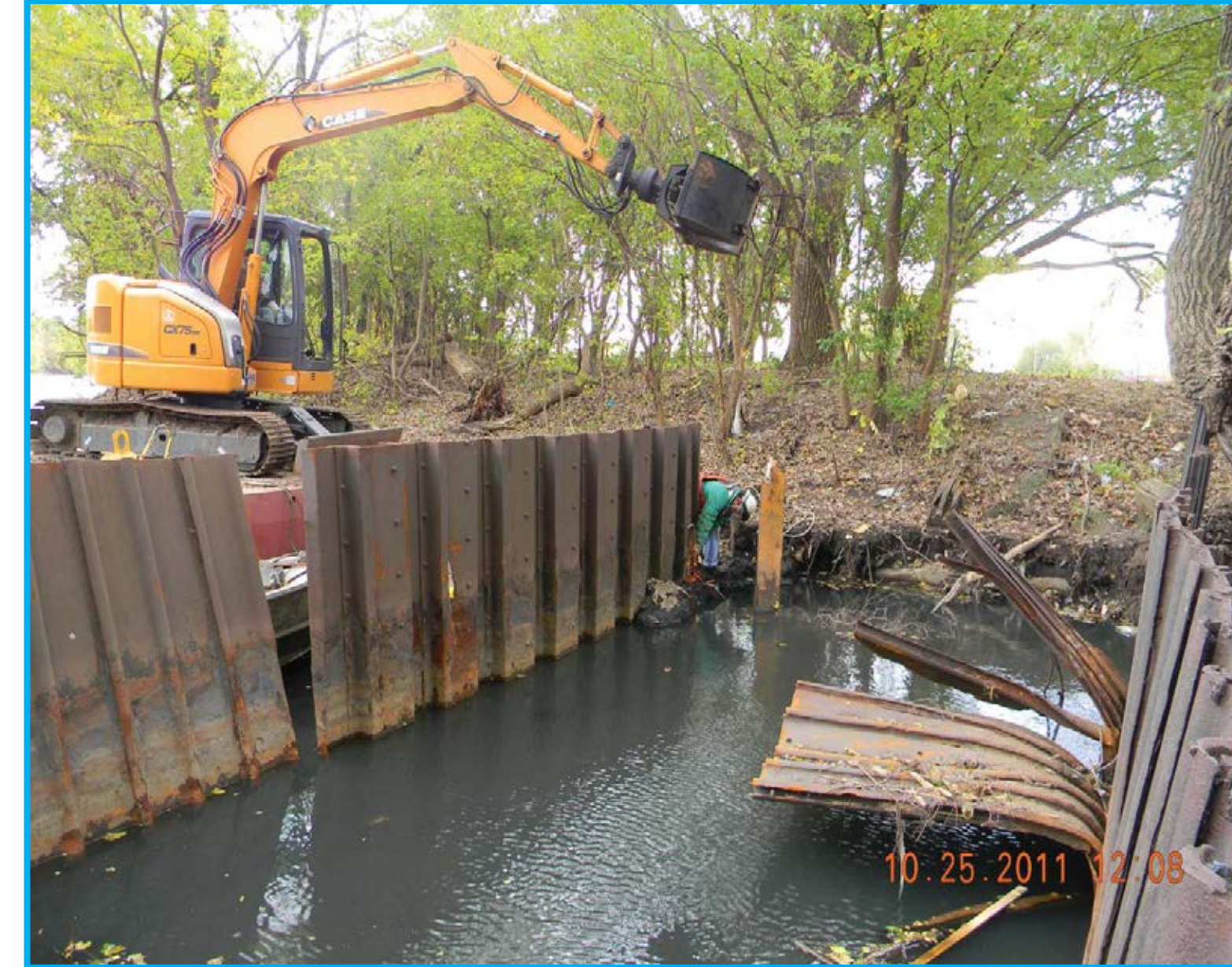
Removing Debris from Banks
