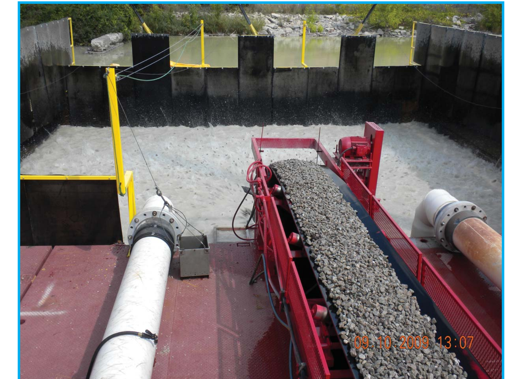
Placing Sand Cap Detail
