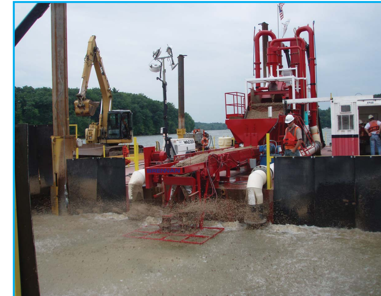
Placing Sand Cap
