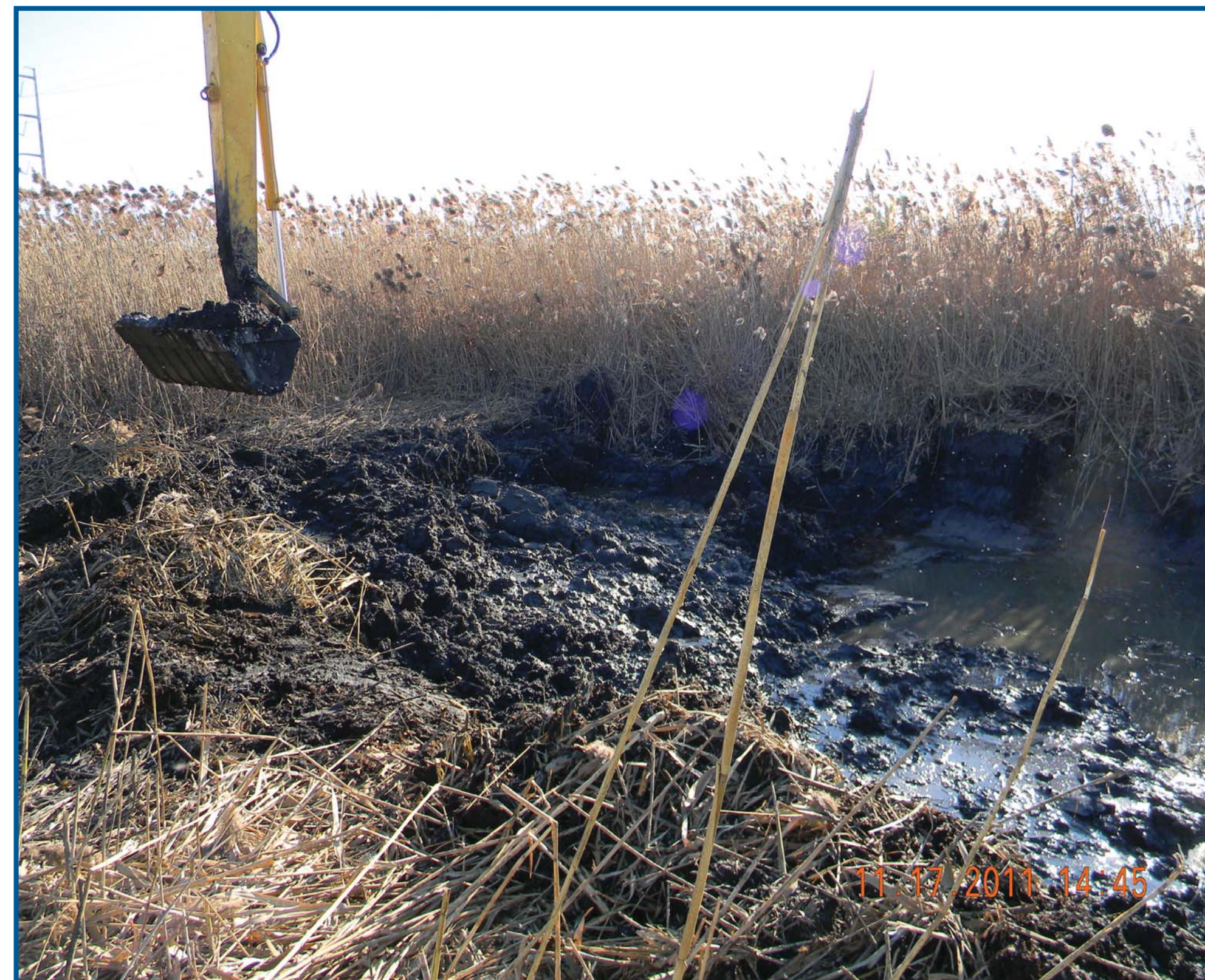
Excavating Marsh Sediment
