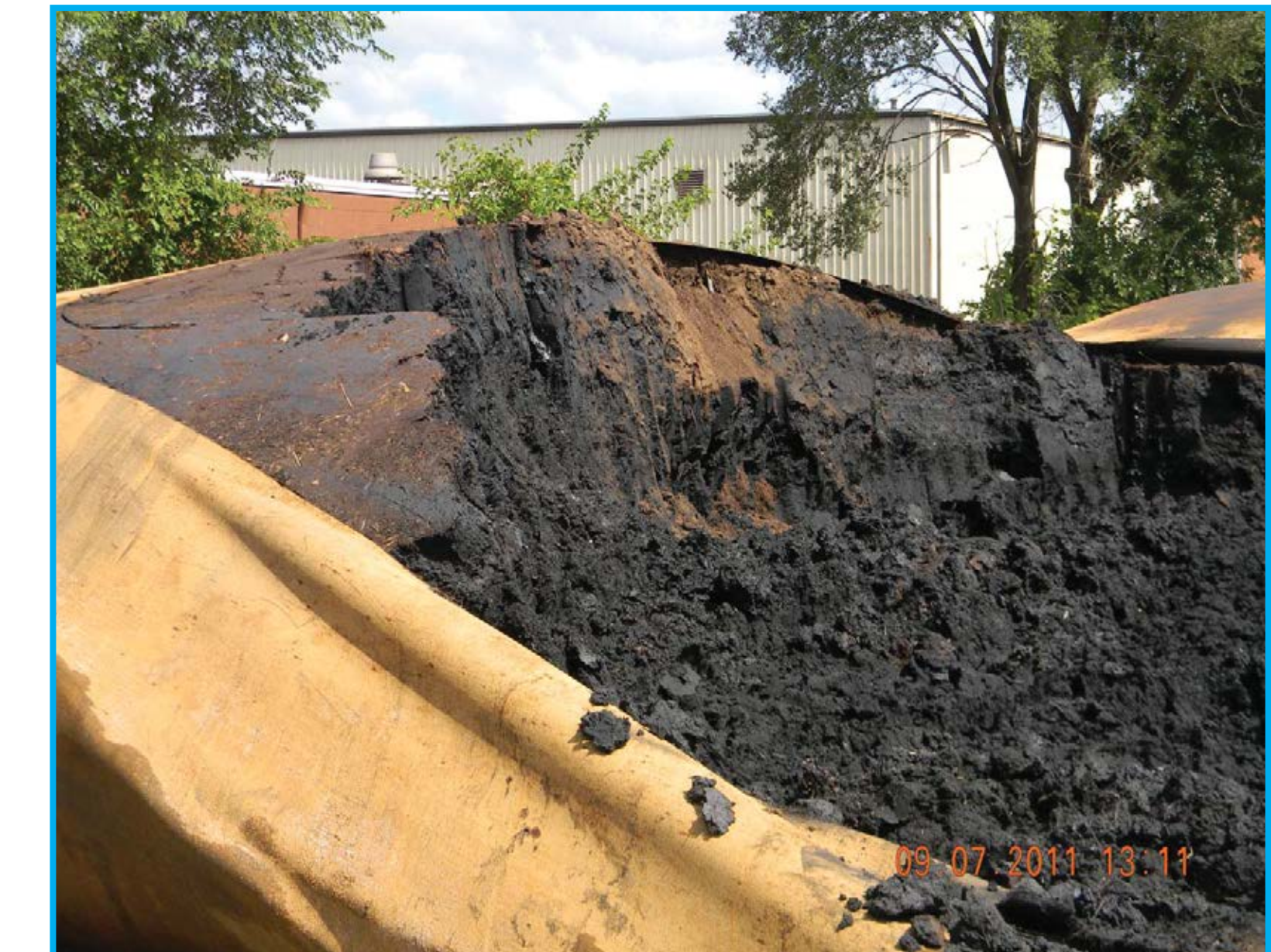
Sediment in Geotextile Tubes
