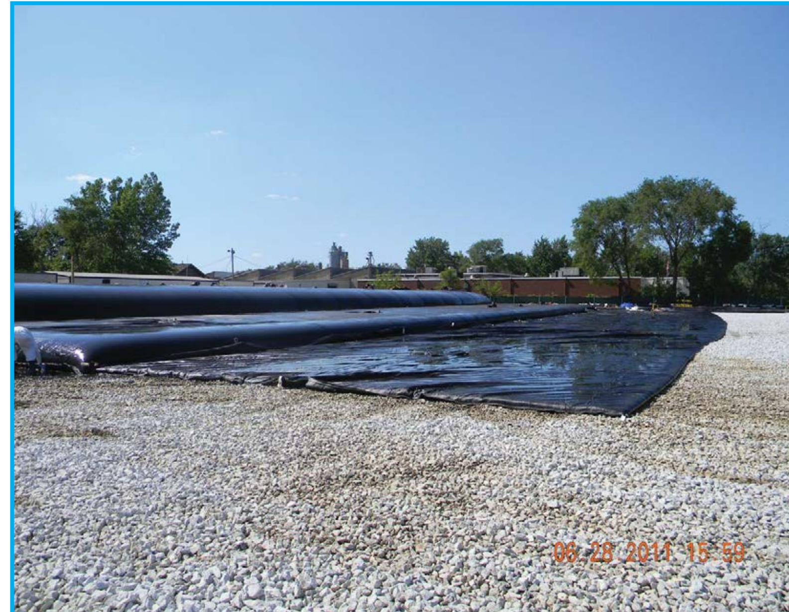
Unrolling Geotextile Tube
