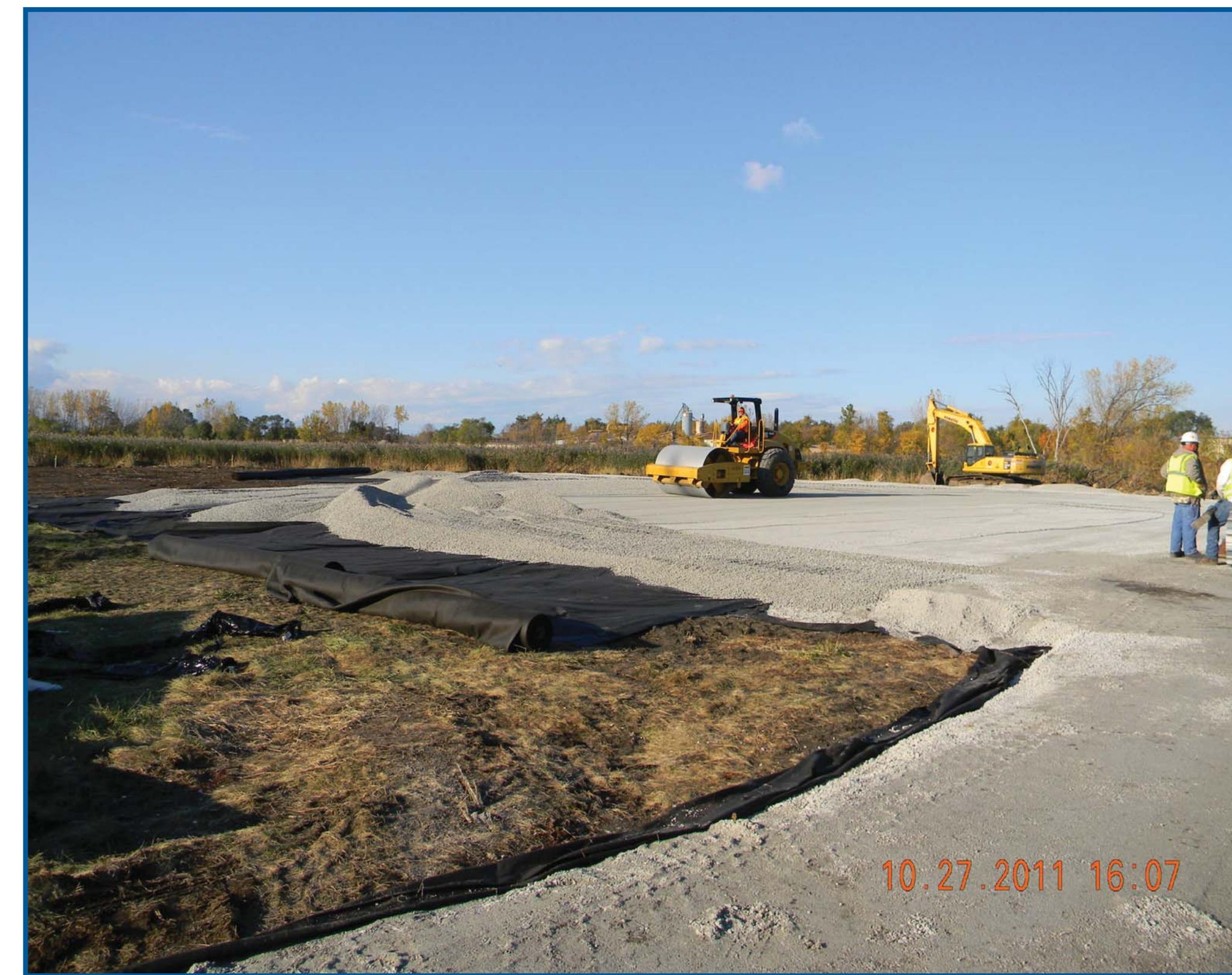
Preparing Sediment Dewatering Area
