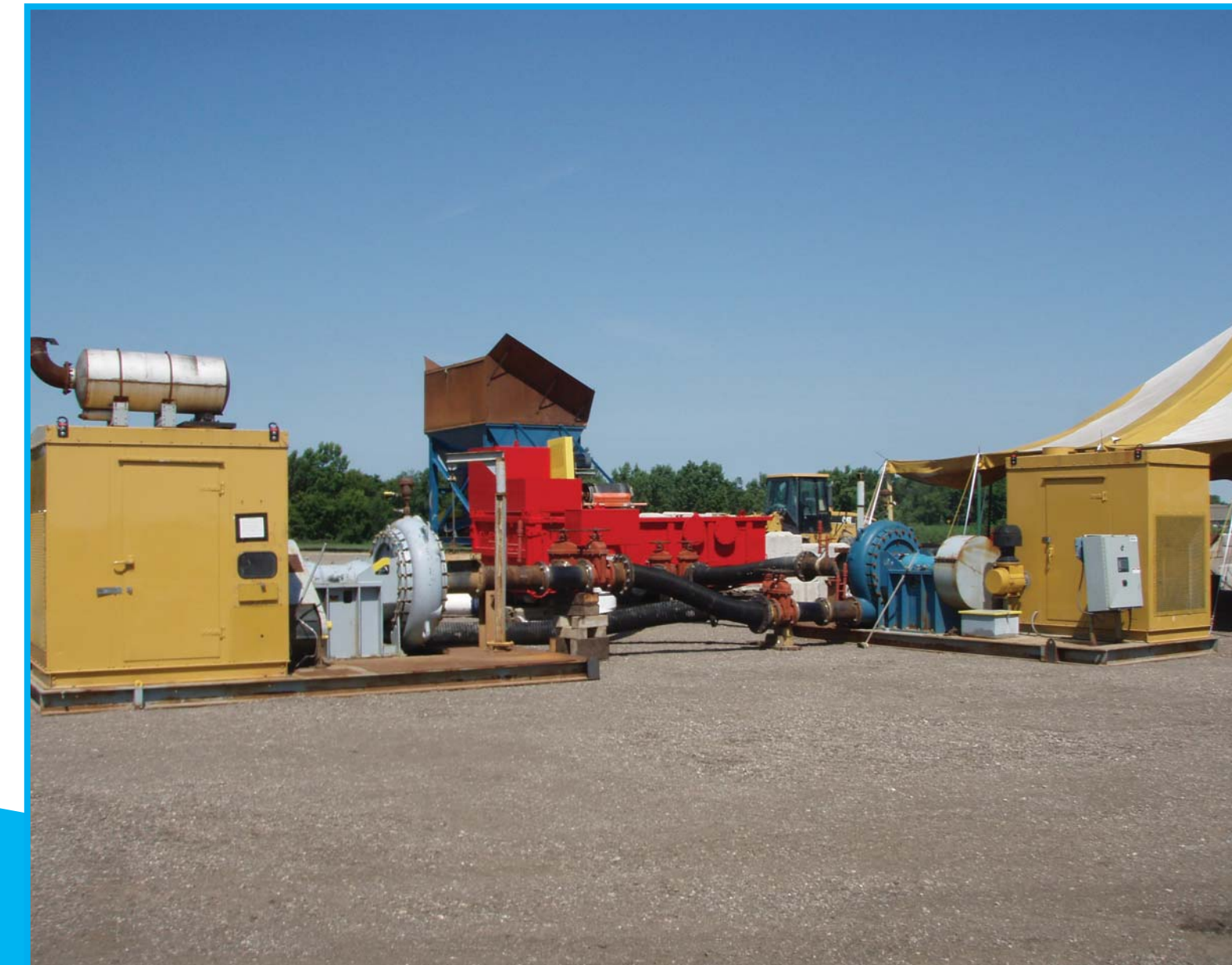
Installing Cap Plant
