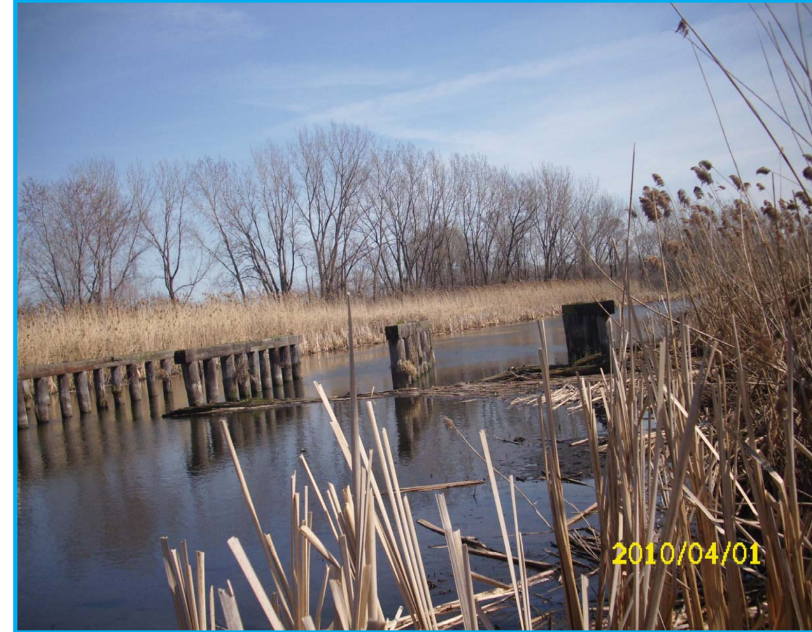
Removing Old Pilings from River
