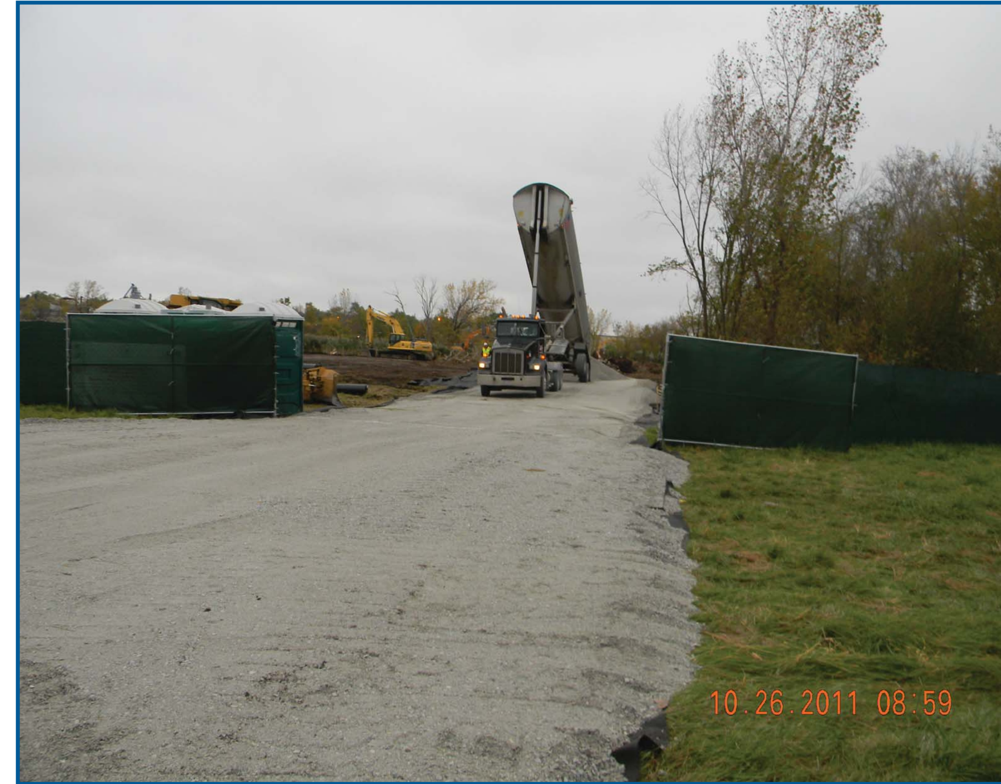
Constructing Staging Area
