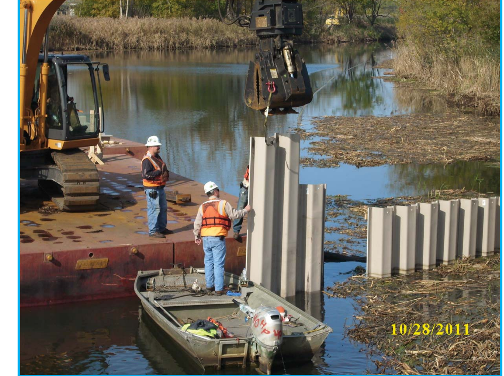
Installing Sheet Pile Weir
