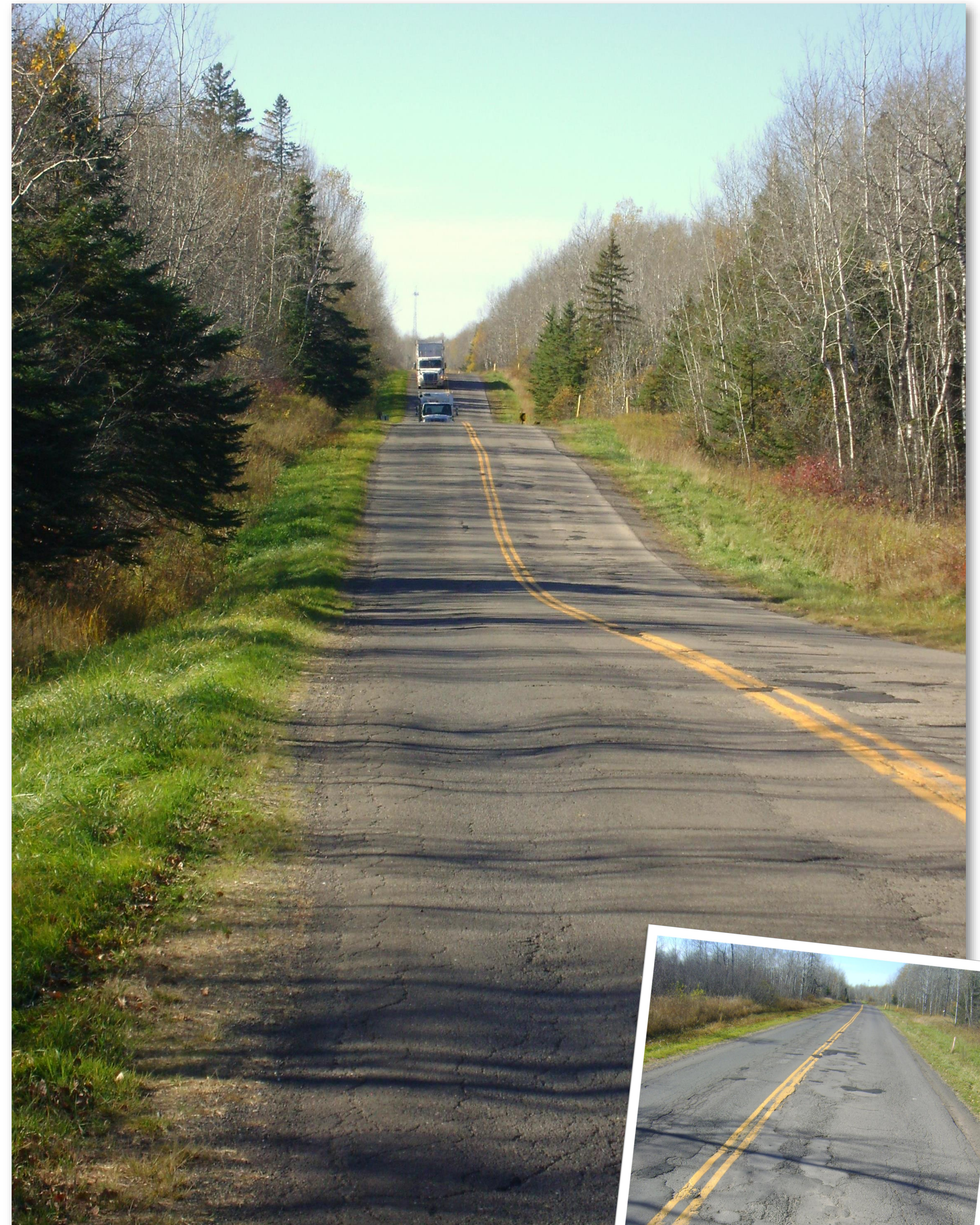
Moccasin Mike Road is the only road leading to the City's landfill, and Wisconsin Point. This road sees intense use by heavy trucks hauling garbage Monday-Saturday. All this traffic has taken a toll, as shown in the photos. Moccasin Mike Road will be re-paved following project completion. Plans to fully reconstruct the road are tentatively set for 2025 after the landfill closes.
