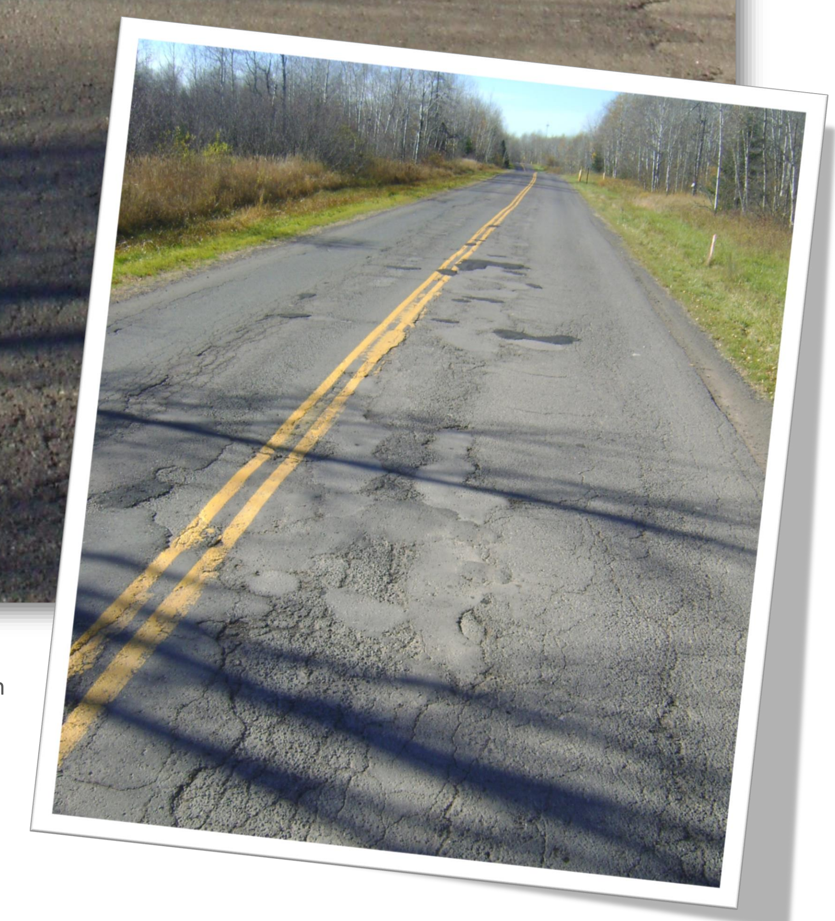
Moccasin Mike Road is the only road leading to the City's landfill, and Wisconsin Point. This road sees intense use by heavy trucks hauling garbage Monday-Saturday. All this traffic has taken a toll, as shown in the photos. Moccasin Mike Road will be re-paved following project completion. Plans to fully reconstruct the road are tentatively set for 2025 after the landfill closes.
