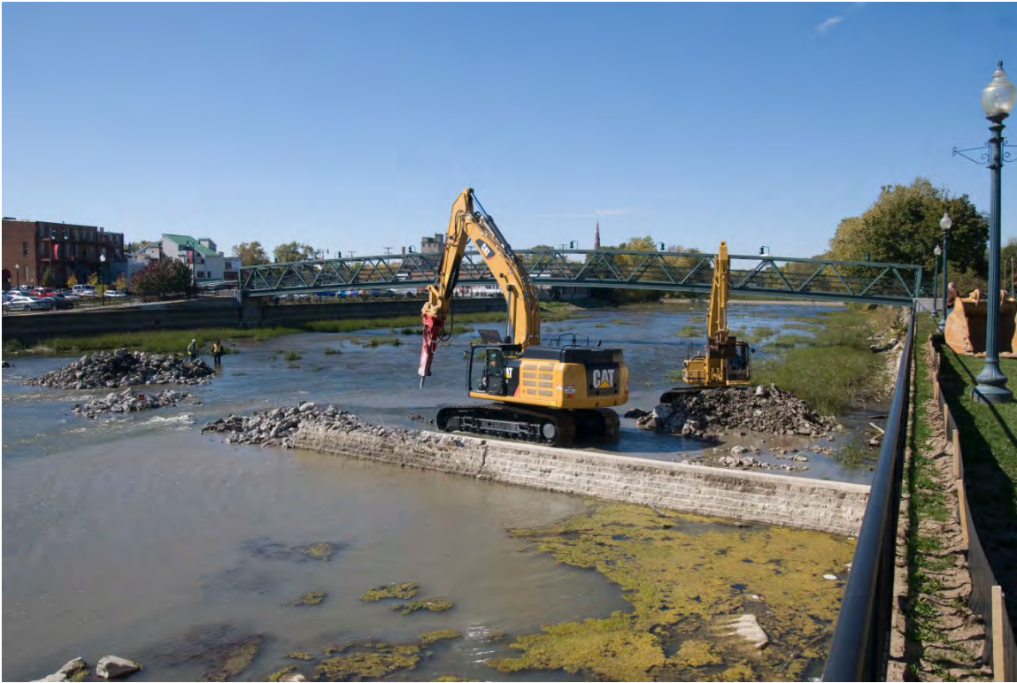
Dam No. 3 during Demolition
