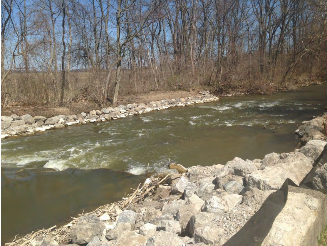
Looking East (Downstream) at the Grape Dam Millrace Improvements
