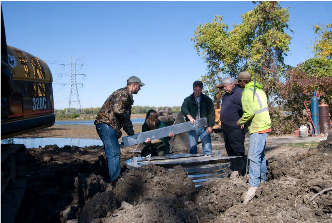
Installation of “Stop-Log” at Water Control Structure
