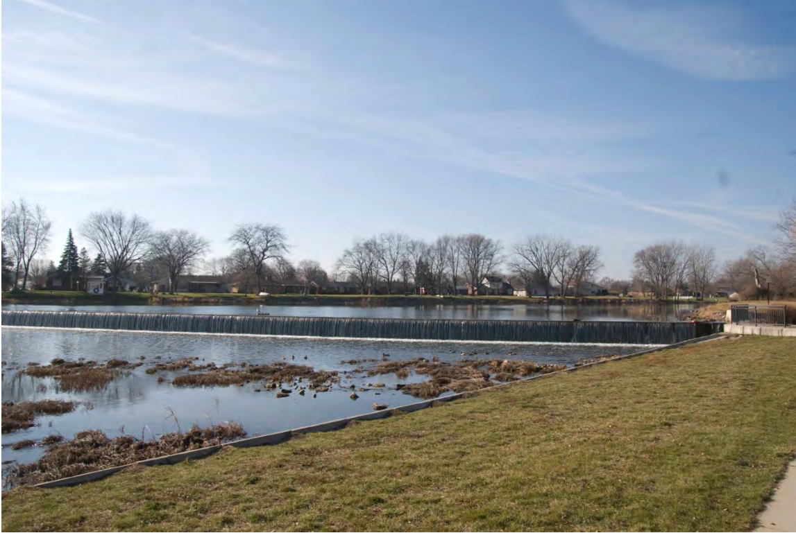
Looking West (Upstream) at the Waterloo Dam (Bypass Channel is to the right of Dam)
