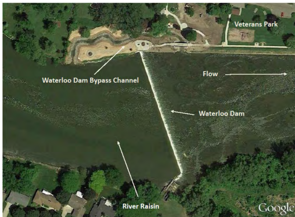
Figure 10: Low Flow Bypass Channel at the Waterloo Dam at Veterans Park
