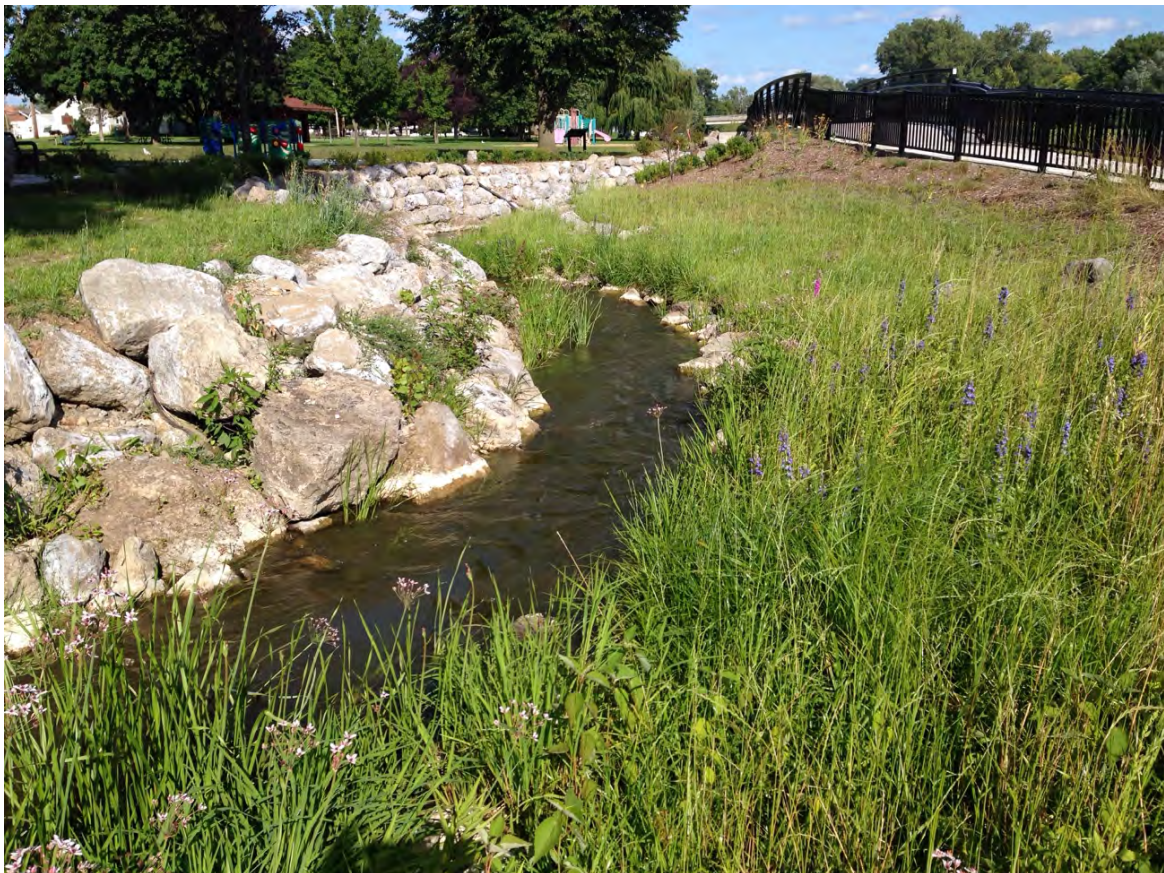
Looking East (Downstream) at the Waterloo Dam Bypass Channel at Veterans Park
