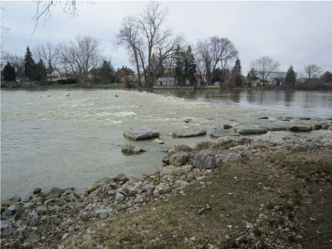
Rock Arch Ramps at Dam No. 5
