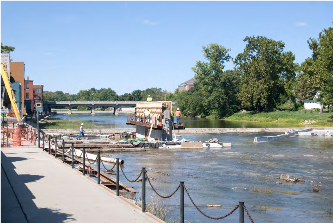
Dam No. 2 Prior to Complete Removal
