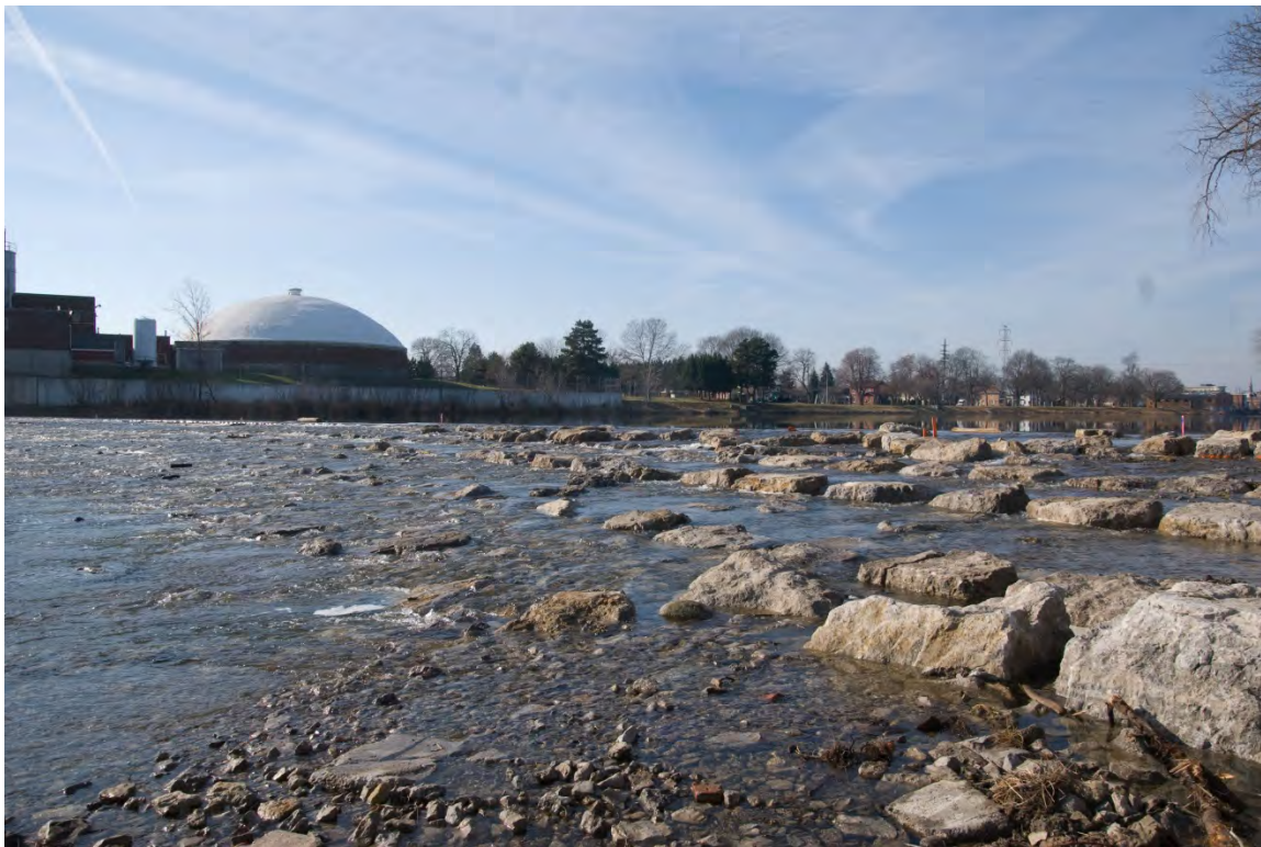
Looking South (and Upstream) at Rock Arch Ramp at Dam No. 1
