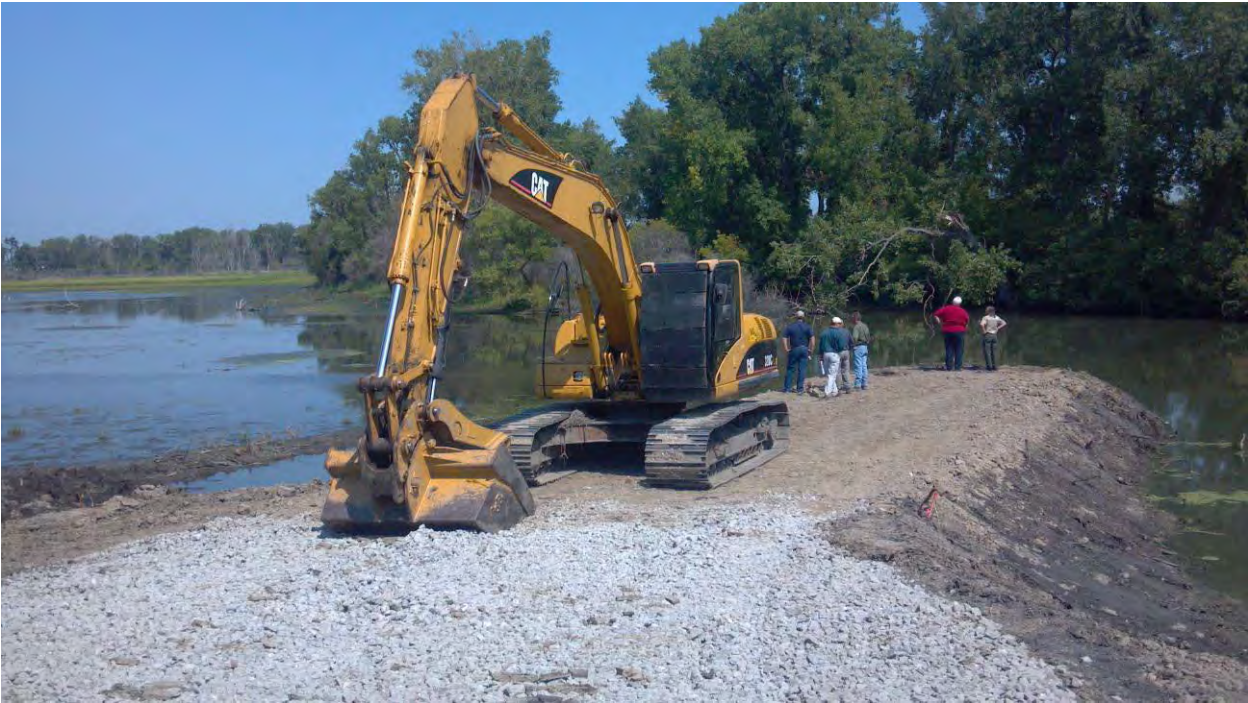
Construction of Union Camp Marsh Dike
