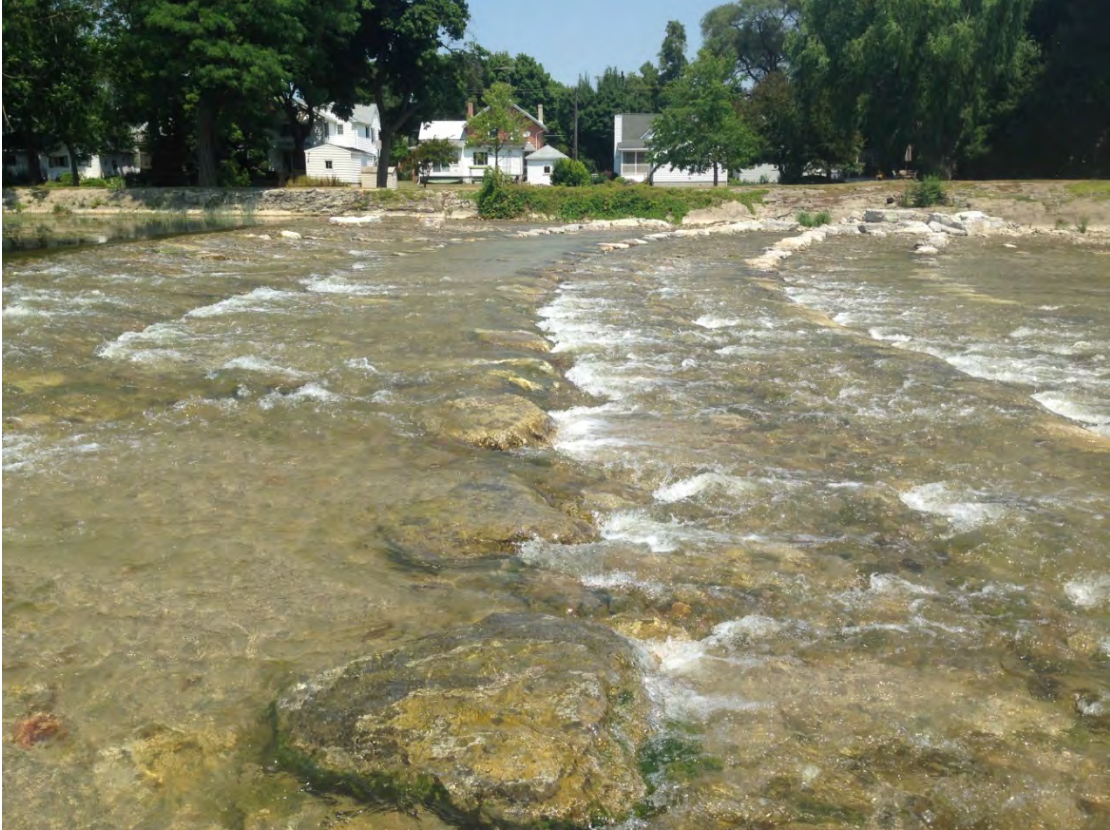
Rock Arch Ramps at Dam No. 4
