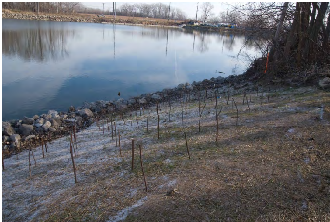
Installation of Live Stakes at Sterling Island
