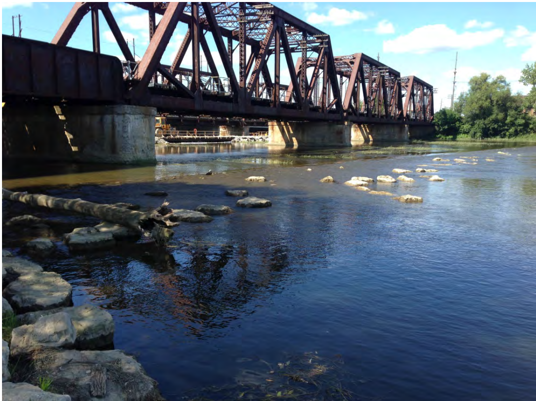
Looking West (Upstream) at Rock Arch Ramp at Dam No. 6
