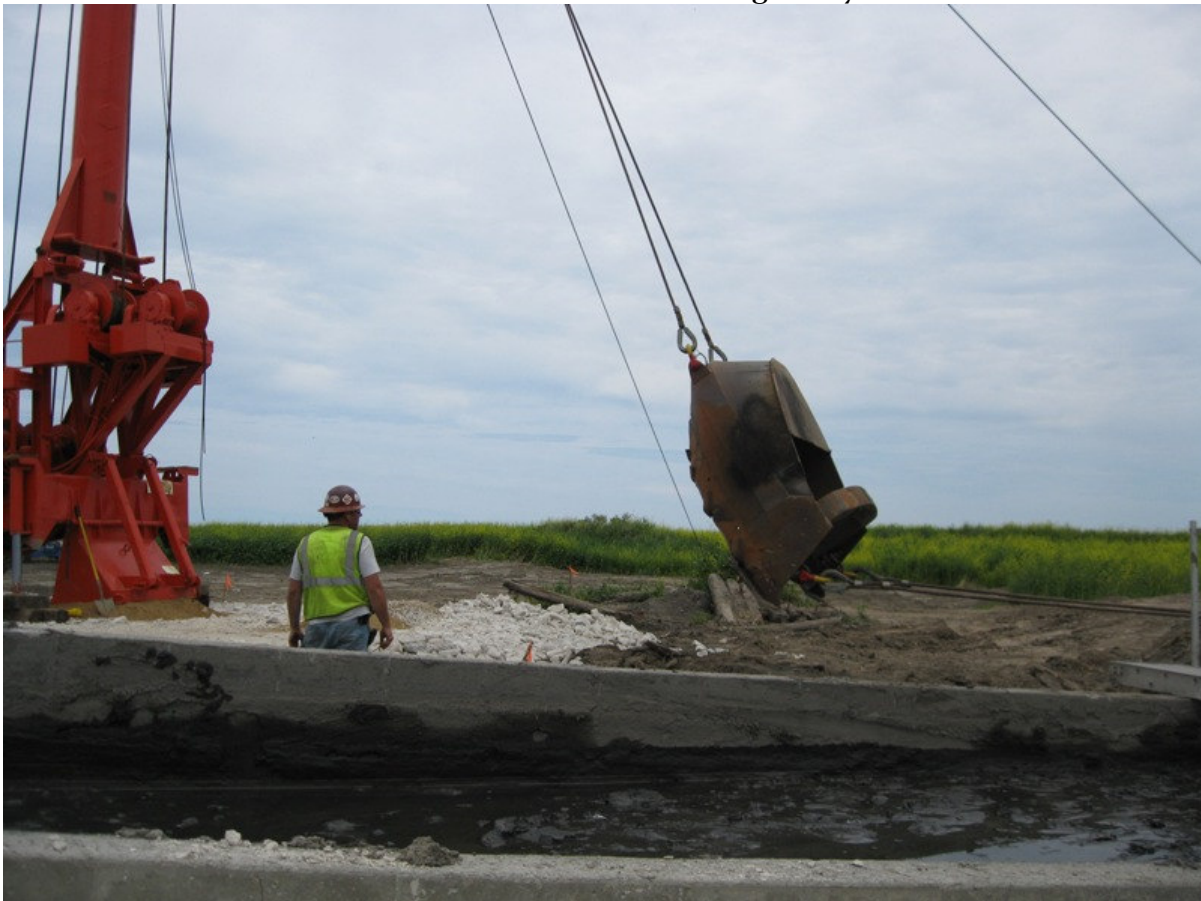
Sauerman bucket installed on dragline system
