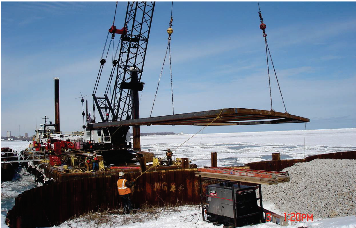
2. The Edward E. Gillen Company (Gillen) constructed the offloading platform at the Milwaukee Harbor CDF. In this photo, the pre-constructed waler system for the offloading platform is being lowered into place as the Gillen employees use taglines to control the load and maintain a separation distance from the overhead hazard.
