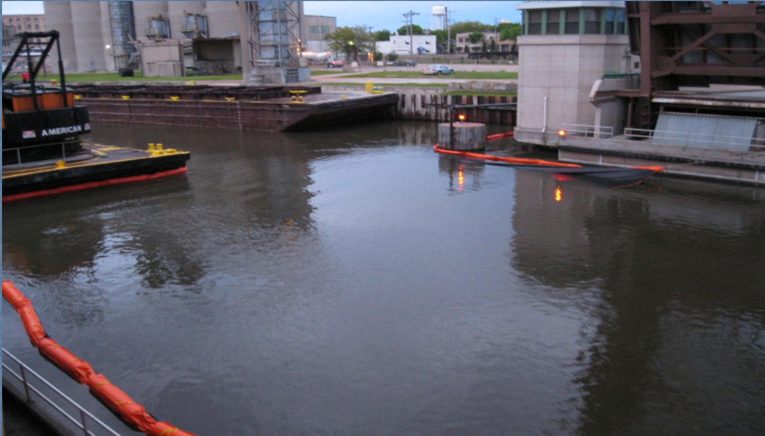
Installation of the turbidity curtain east of the Kinnickinnic Avenue Bridge.
