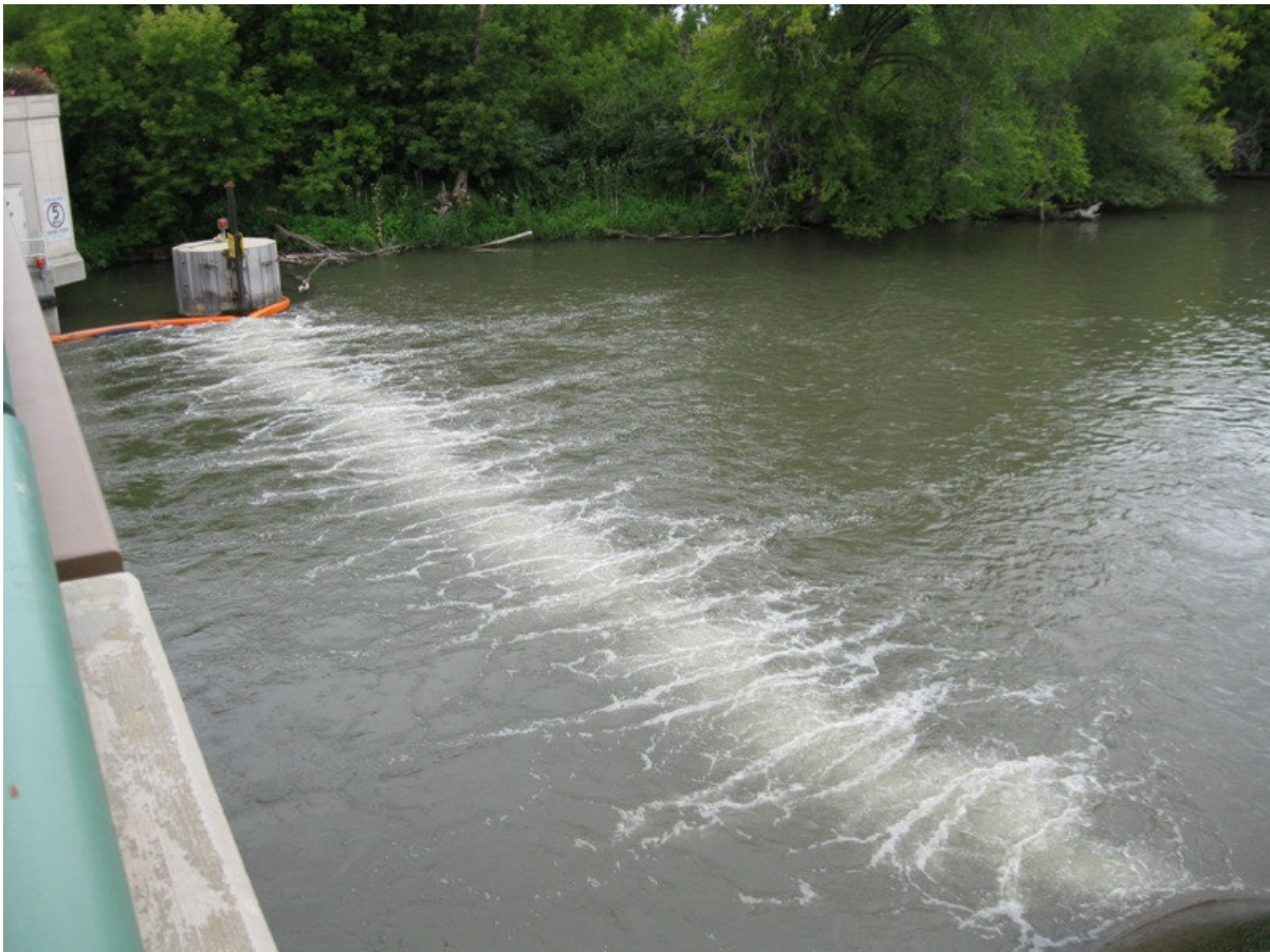
Air Curtain in Operation
