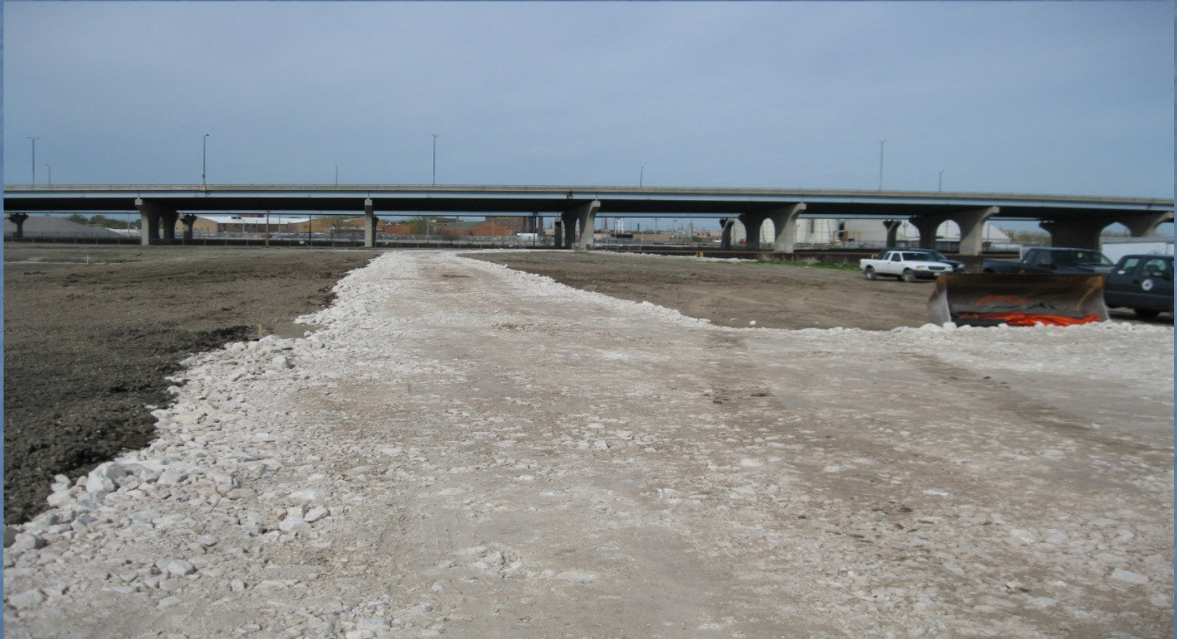
Road constructed to the offloading platform (looking to the west).
