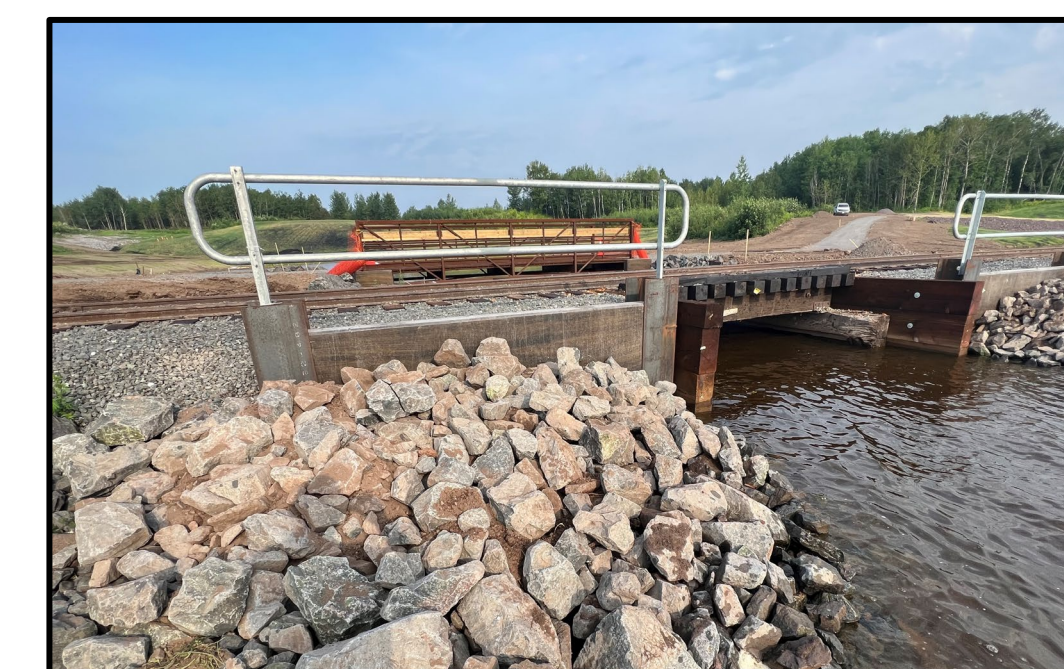
Rock is placed near the bridges for additional shoreline erosion protection.
