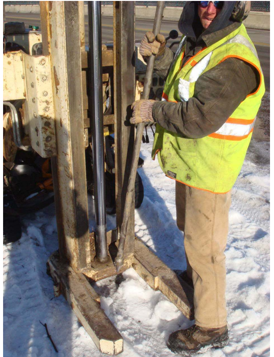
Solid drive-point used for sediment probing with Geoprobe rig
