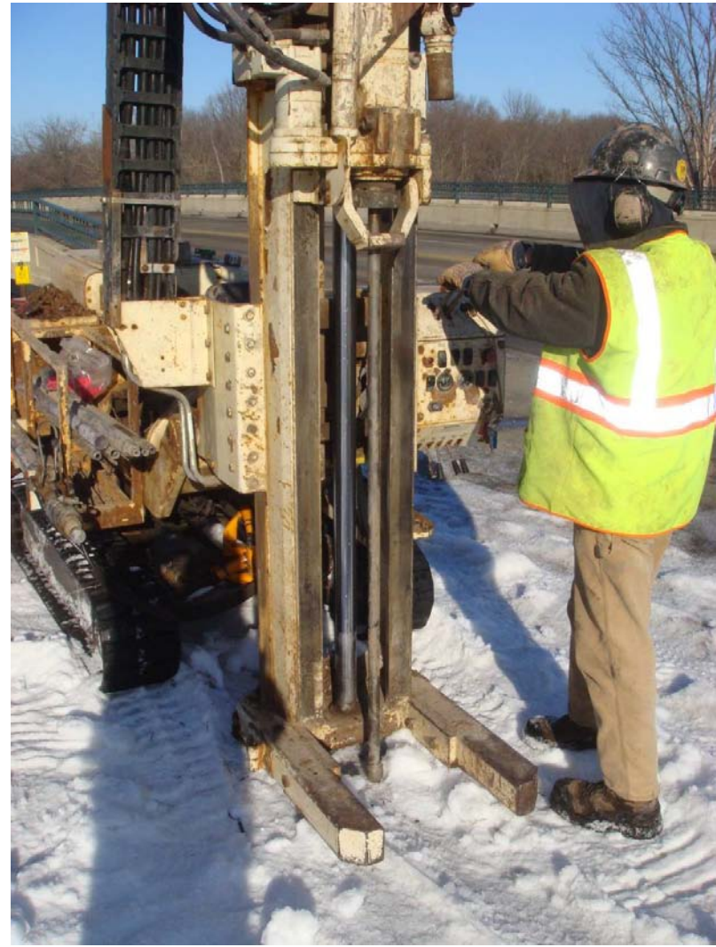
Solid point attached to rods prior to probing.
