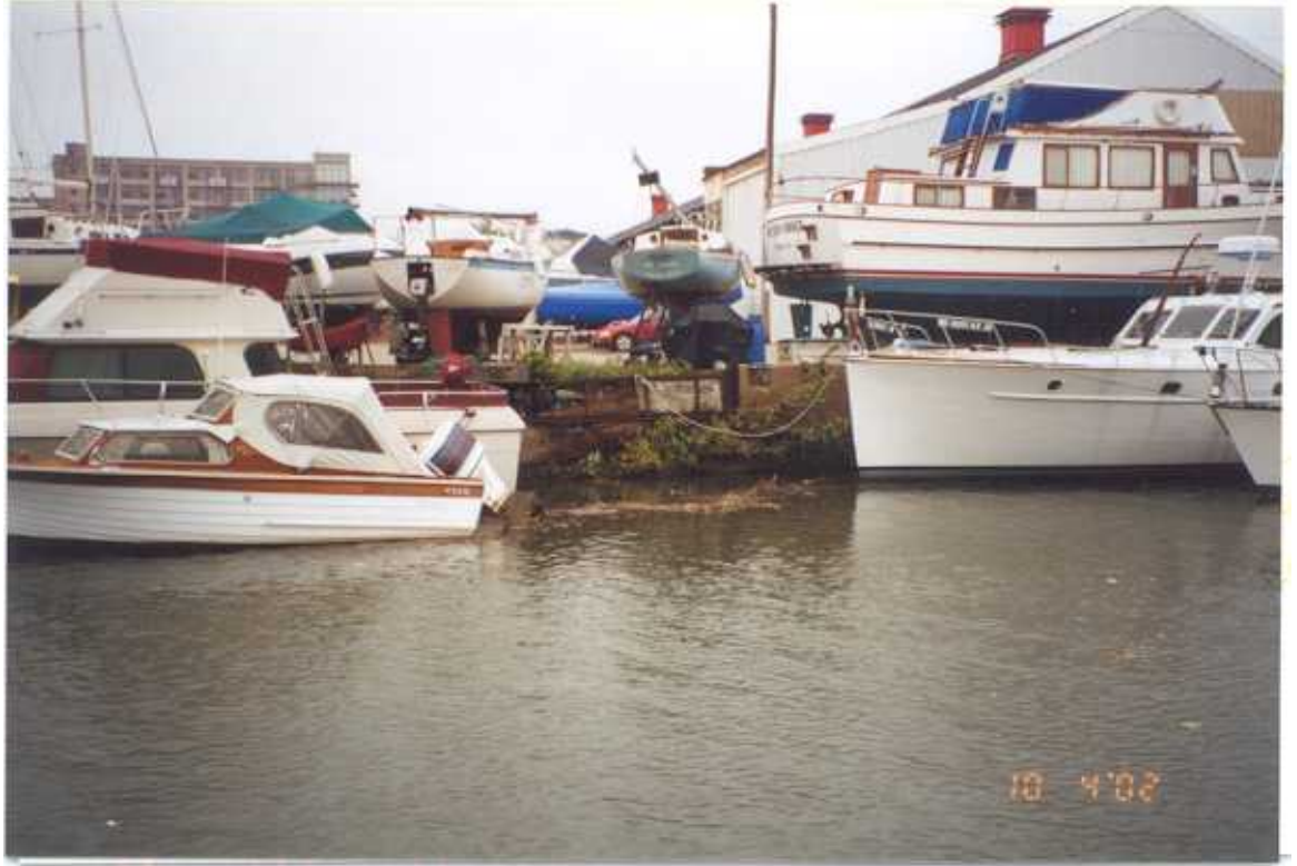
PHOTO 24 – October 4, 2002 – Kinnickinnic River Taken by Tor Hansen, Barr Engineering Downstream end of timber dock and wall at Parcel 426B and upstream end of concrete dock and timber wall at Parcel 426A. Looking north.
