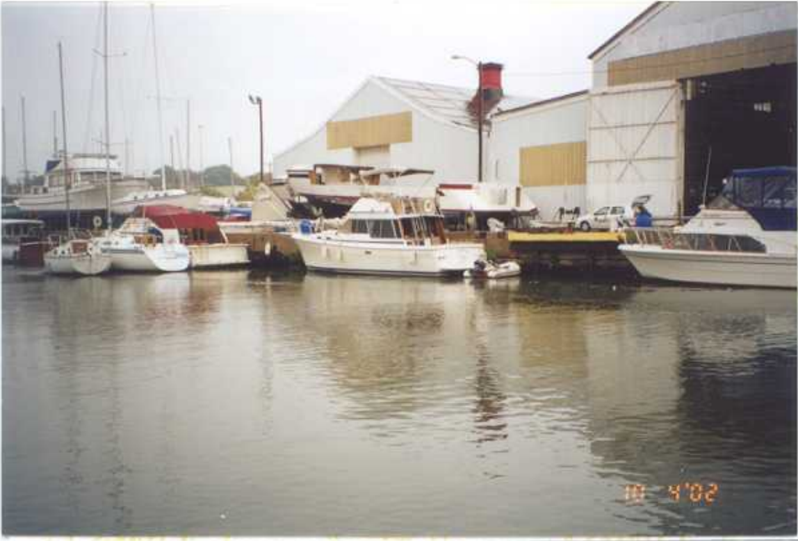
PHOTO 26 – October 4, 2002 – Kinnickinnic River Taken by Tor Hansen, Barr Engineering Concrete dock and timber wall at Parcel 426A. Looking north.
