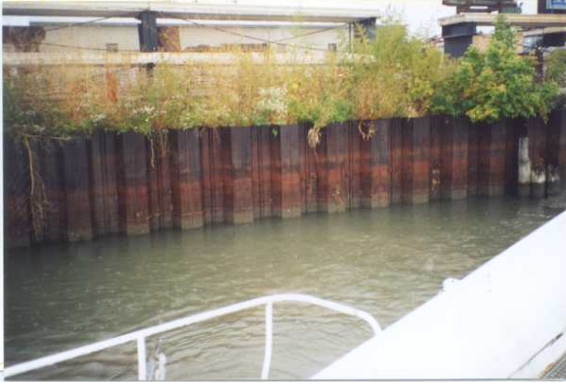
PHOTO 49 – October 4, 2002 – Kinnickinnic River Taken by Tor Hansen, Barr Engineering Steel sheet pile wall along Parcel 433. Looking east.
