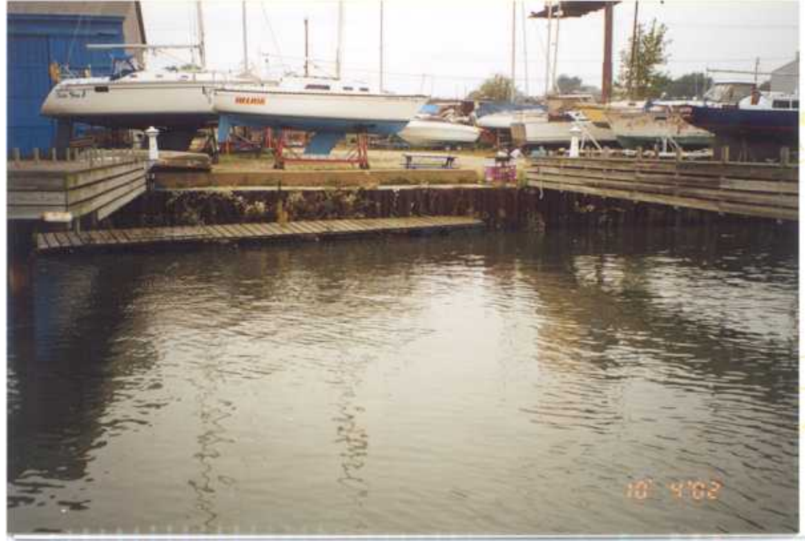
PHOTO 8 – October 4, 2002 – Kinnickinnic River Taken by Tor Hansen, Barr Engineering Steel sheet pile wall along Parcel 429. Looking west.
