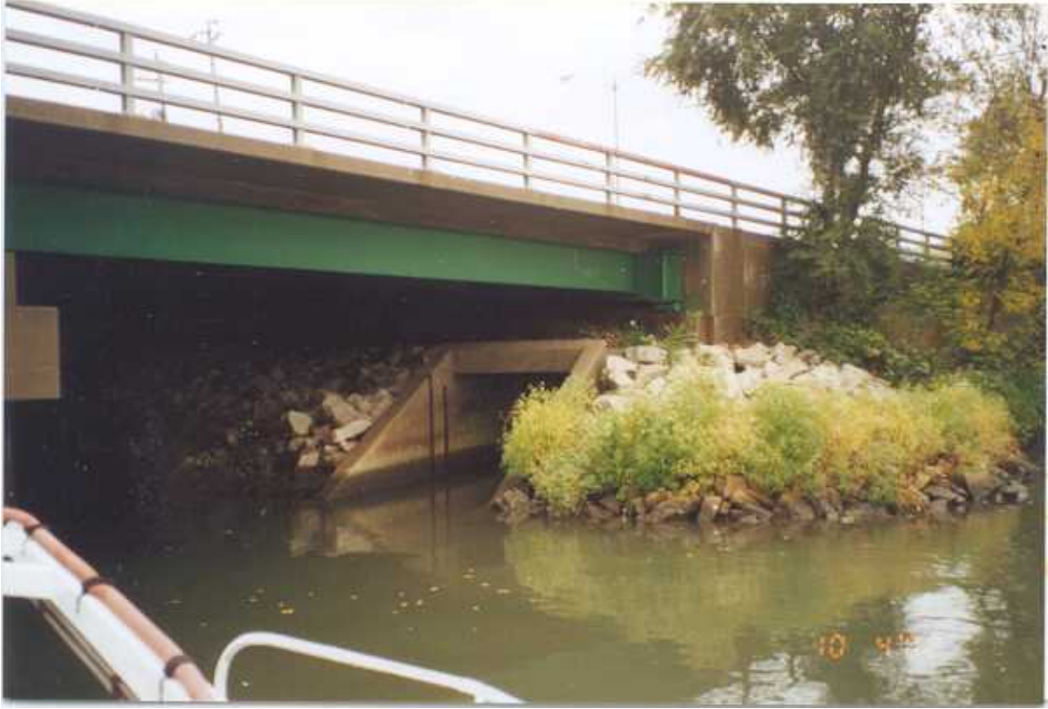
PHOTO 2 – October 4, 2002 – Kinnickinnic River Taken by Tor Hansen, Barr Engineering Left abutment Becher Street Bridge showing concrete box stormwater outlet. Taken from boat in river while looking southwest.
