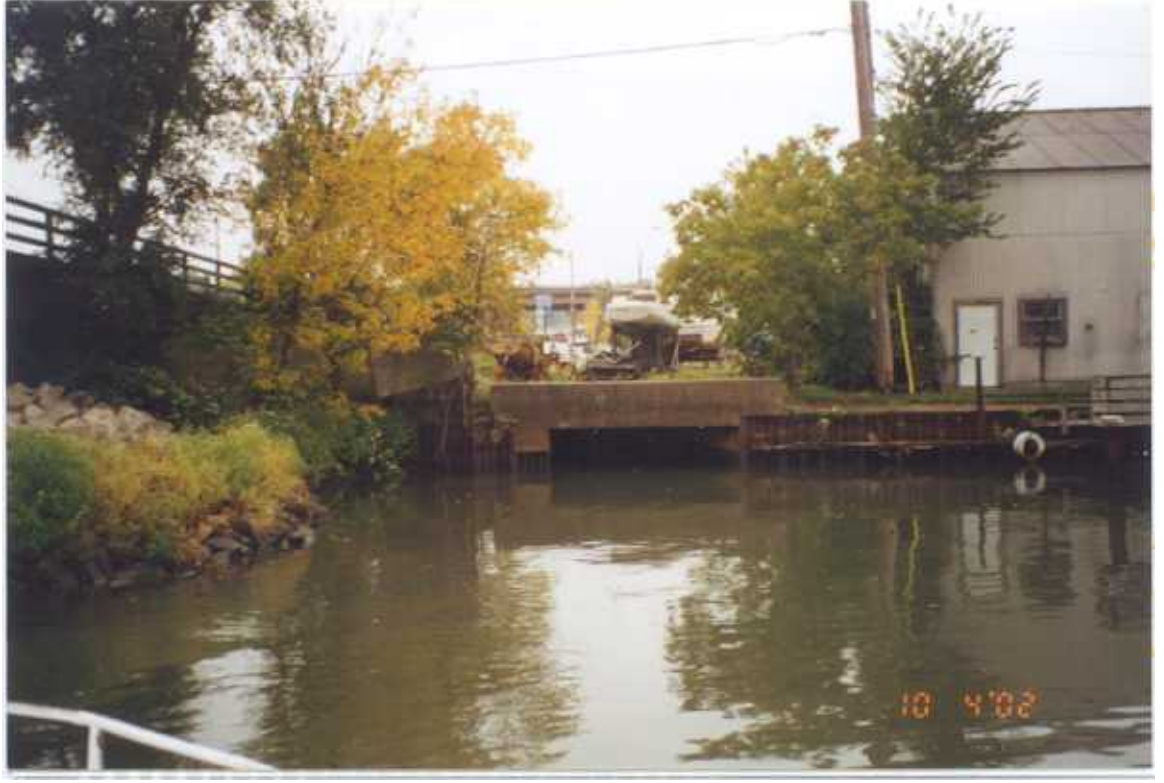
PHOTO 3 – October 4, 2002 – Kinnickinnic River Taken by Tor Hansen, Barr Engineering Concrete box stormwater outlet and upstream end of steel sheet pile wall along Parcel 429. Taken from boat looking west.
