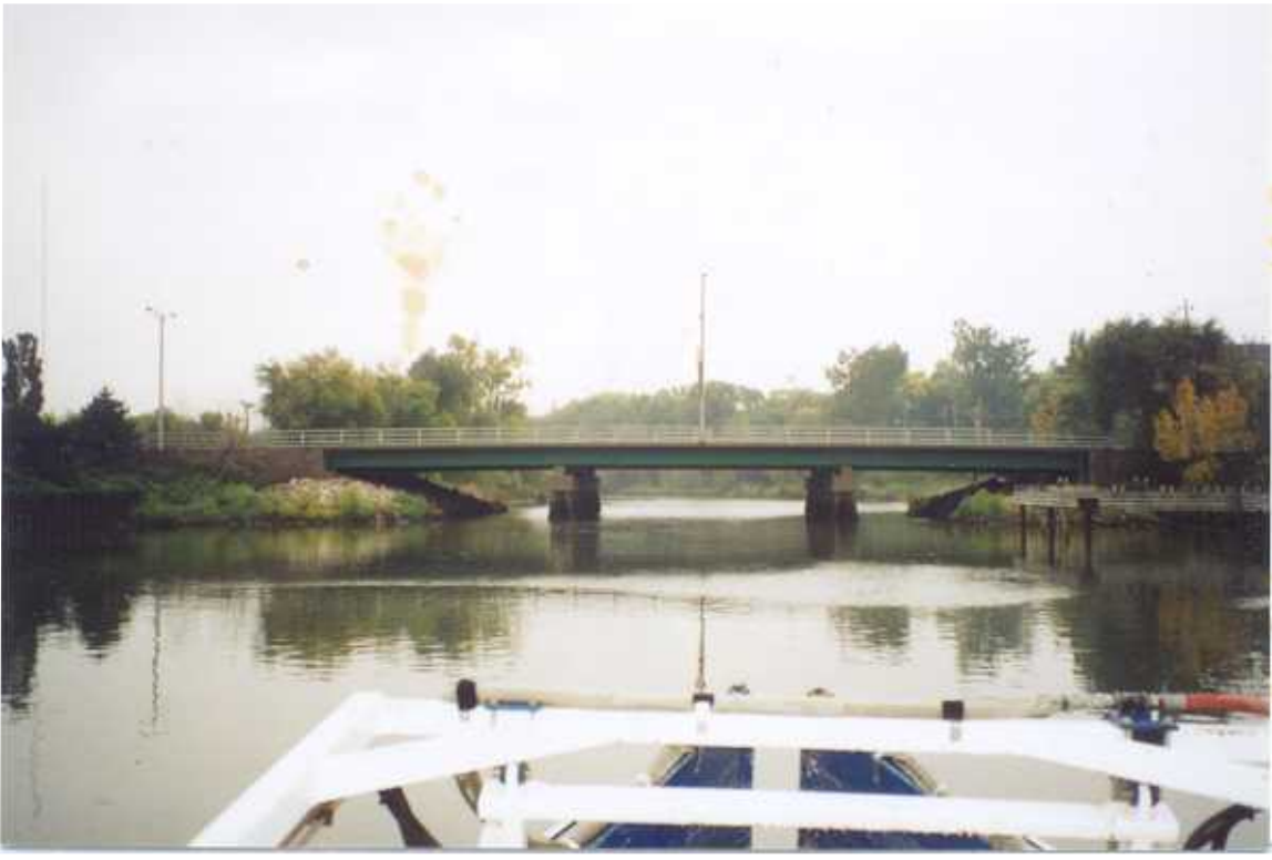
PHOTO 1 – October 4, 2002 – Kinnickinnic River Taken By Tor Hansen, Barr Engineering Becher Street Bridge looking upstream (South)
