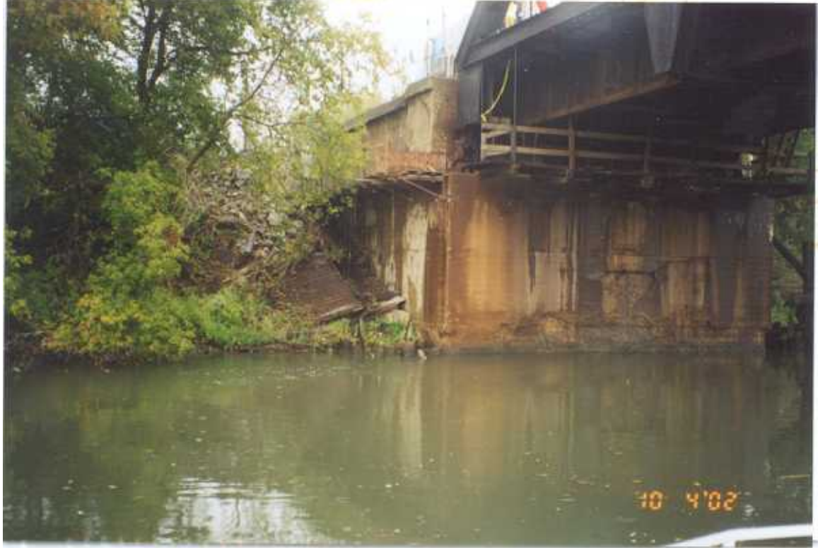
PHOTO 40 – October 4, 2002 – Kinnickinnic River Taken by Tor Hansen, Barr Engineering Railroad bridge abutment at downstream end of Parcel 425 downstream from photo 39. Looking north
