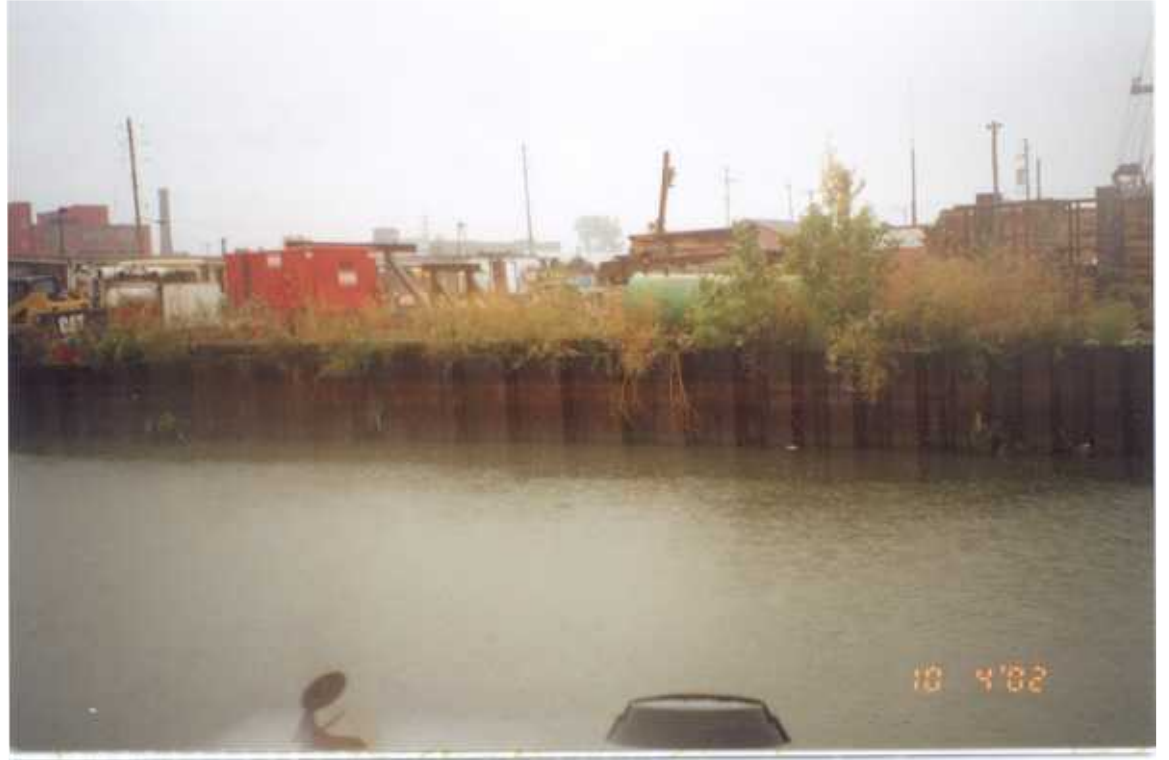
PHOTO 56 – October 4, 2002 – Kinnickinnic River Taken by Tor Hansen, Barr Engineering Steel sheet pile wall along Parcel 433. Looking south.
