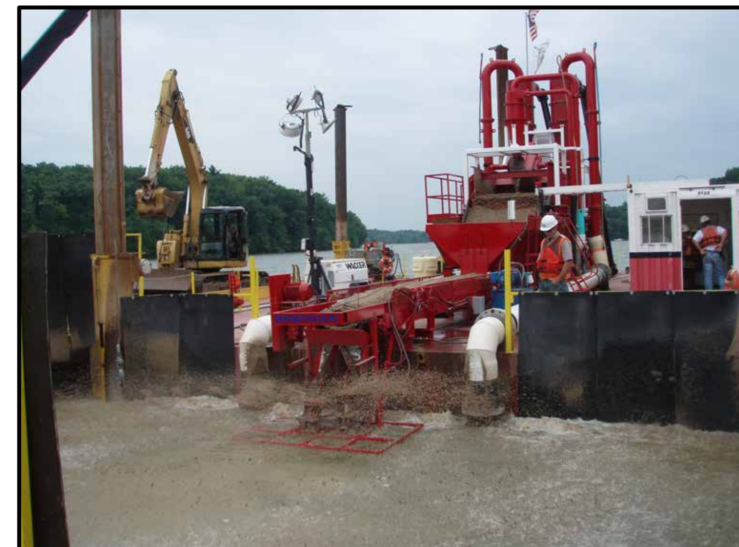
Placing Sand Cap
