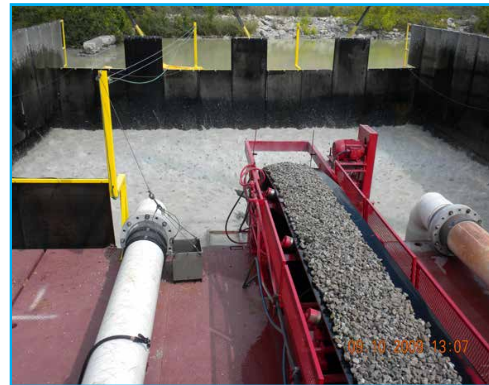
Placing Sand Cap Detail
