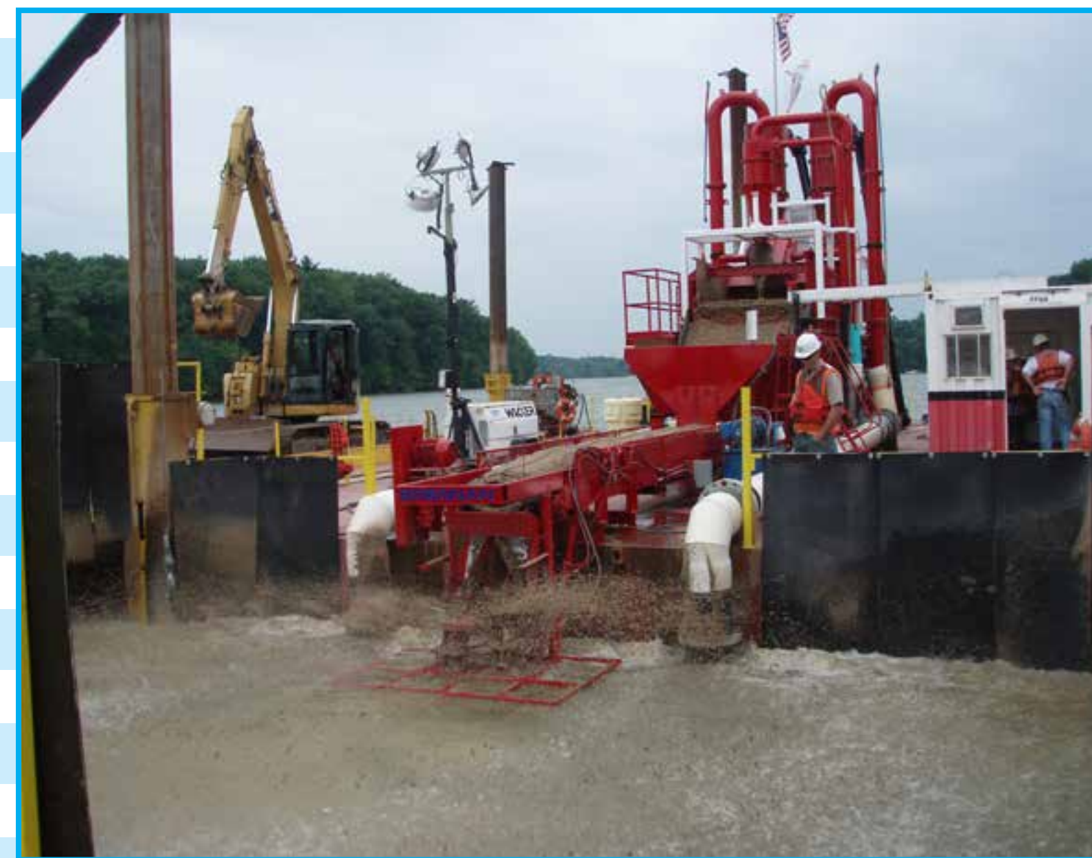
Placing Sand Cap
