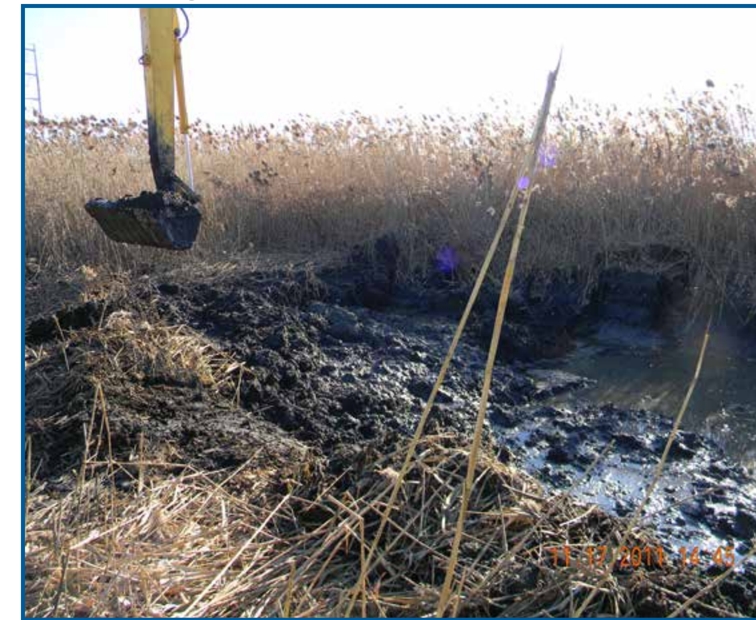
Excavating Marsh Sediment
