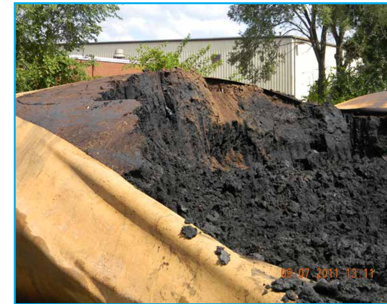
Sediment in Geotextile Tubes
