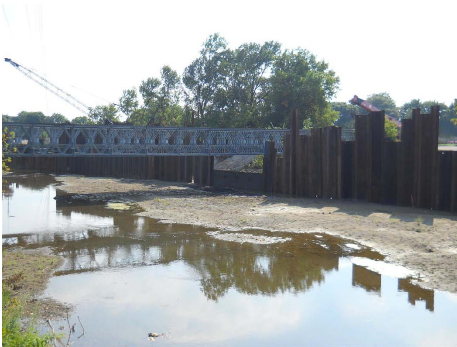
Figure 3: Completion of the inline sheeting under the tower access bridge (8/31/2011)
