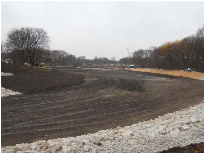
Figure 13: Zone 2A after completion of excavation activities (11/26/2011)
