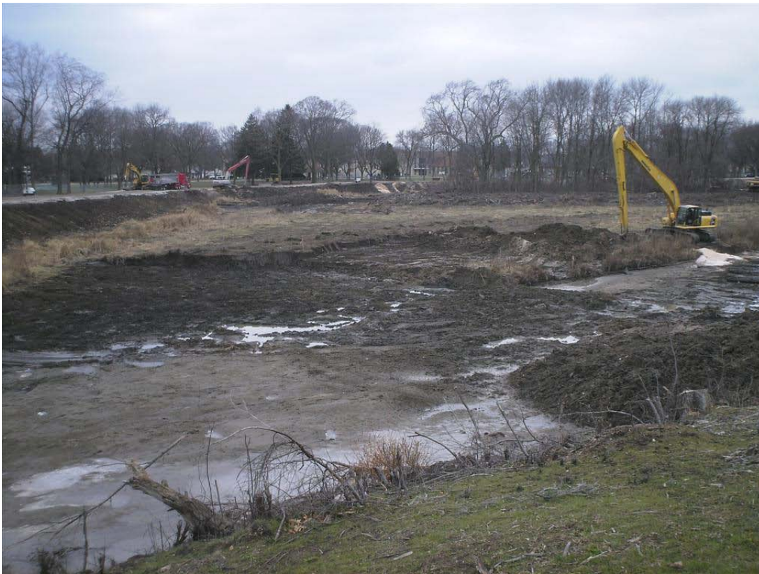
Figure 16: Excavation of sediments in the eastern end of Zone 2B (12/19/2011)
