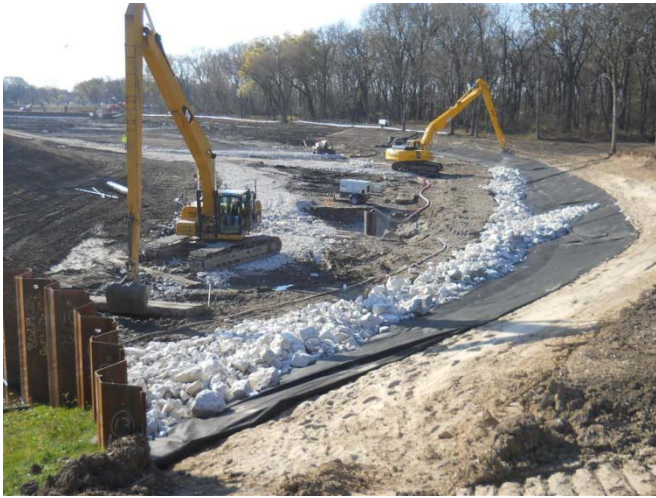
Figure 11: Riprap placement per detail 2 along the north bank of Zone 2A (11/15/2011)
