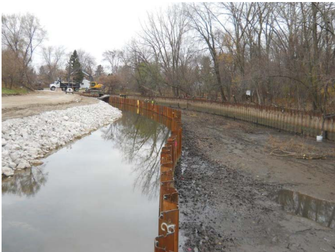
Figure 12: Zone 1 east dewatering and excavation (11/21/2011)
