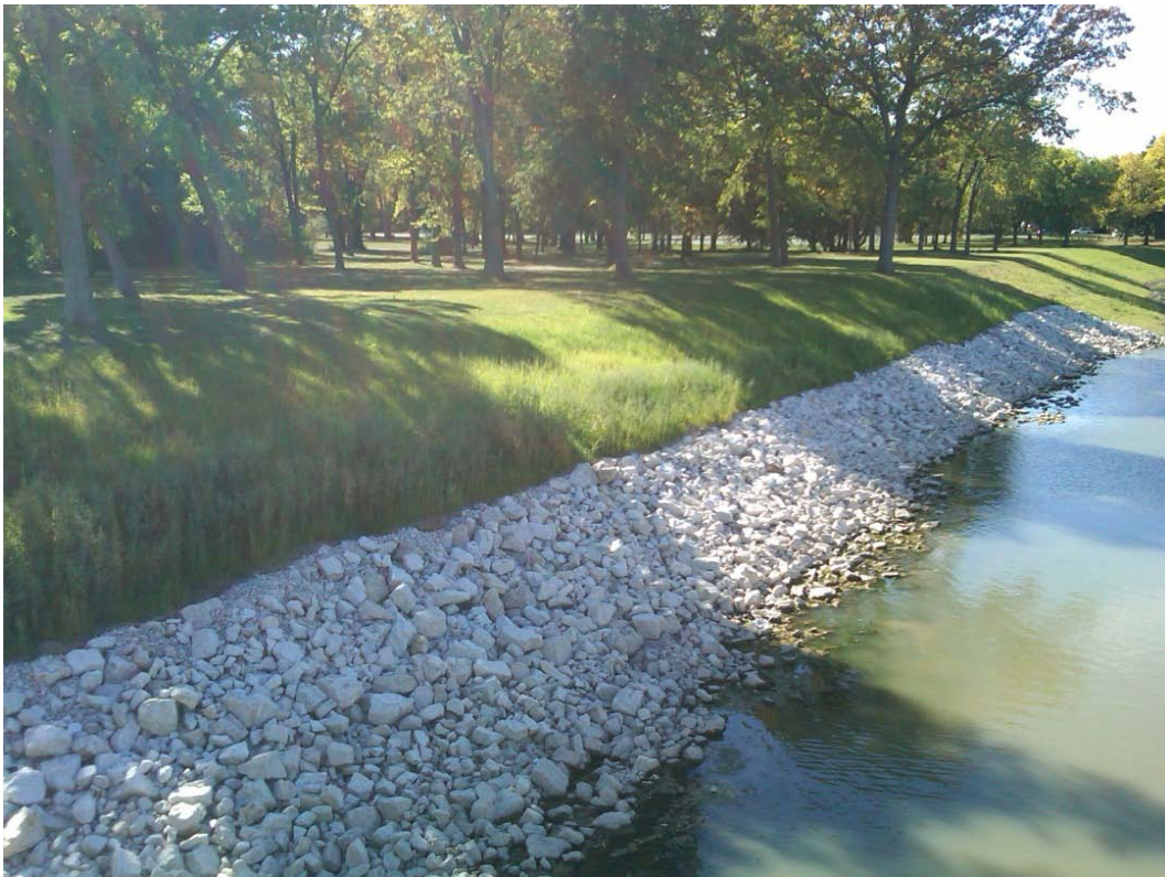
Figure 23: Zone 2B South – view from MKE Pkwy Bridge (September 2012)
