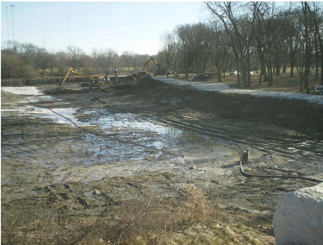
Figure 17: Excavation of sediments and dewatering activities in Zone 3A (1/5/2012)
