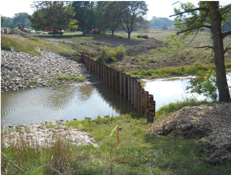
Figure 6: Sheet pile wall completed on the east end of Zone 2A (9/20/2011)
