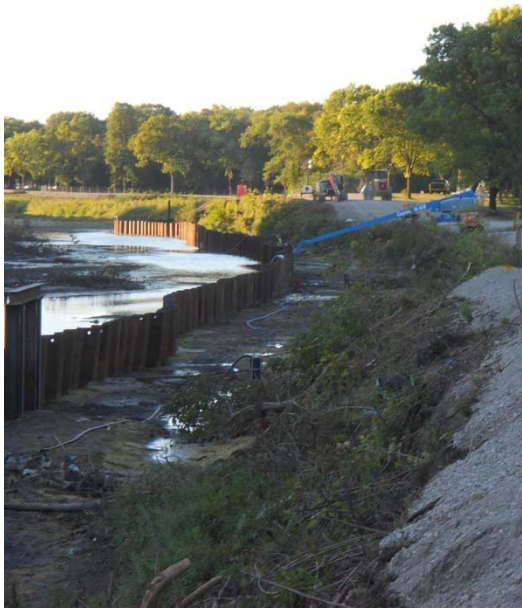
Figure 4: Dewatered west side of Zone 1 (9/15/2011)
