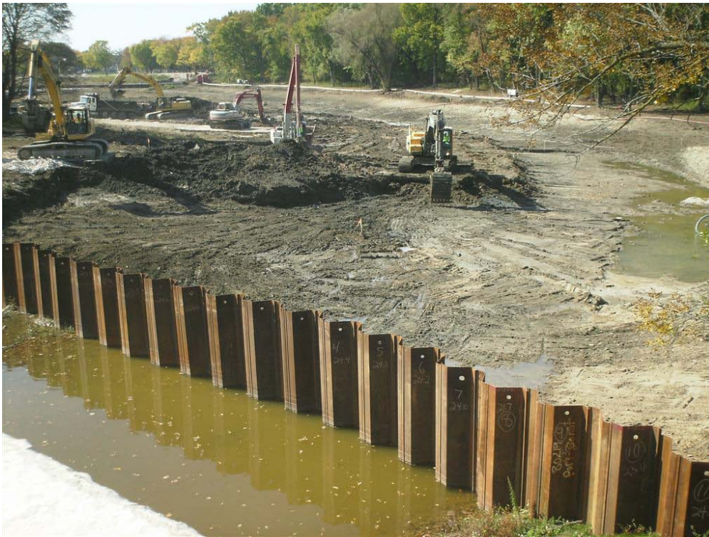
Figure 9: Eastern end of Zone 2A during excavation activities (10/8/11)
