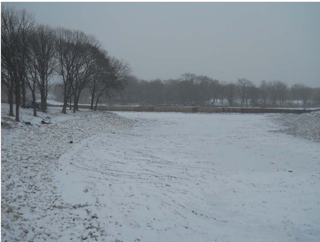
Figure 19: Completed riprap placement in Zone 3A (1/20/2012)
