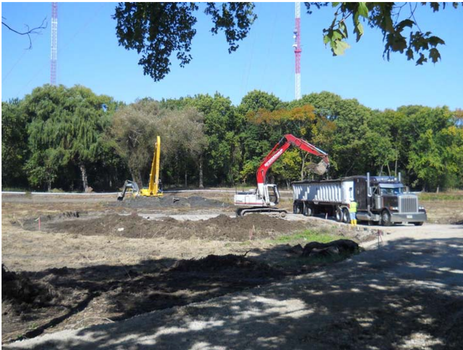
Figure 8: Excavation and hauling of TSCA material in Zone 2A (10/3/2011)
