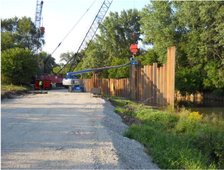
Figure 1: Sheet piling installation south of the overhead power lines (8/19/2011)
