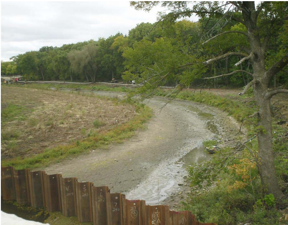
Figure 7: Post dewatering efforts in Zone 2A (9/30/2011)
