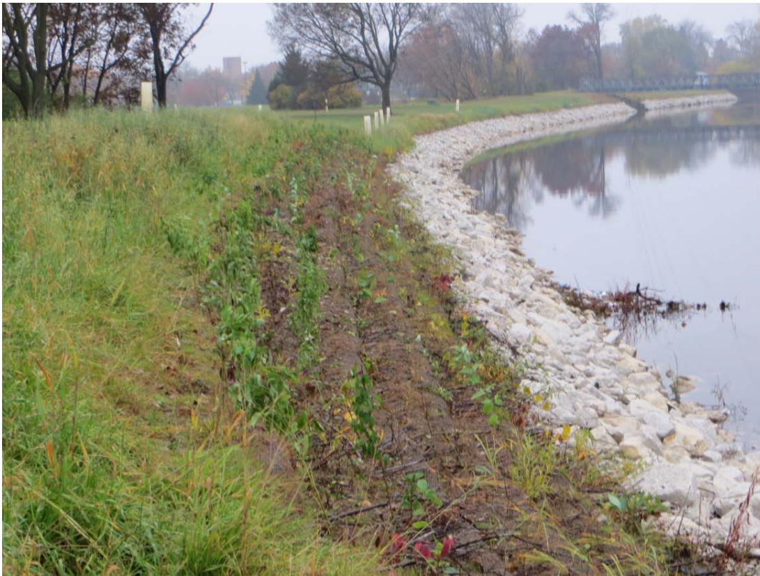
Figure 25, Zone 1, Soil lift planting, plugs and seedlings. (October 2012)
