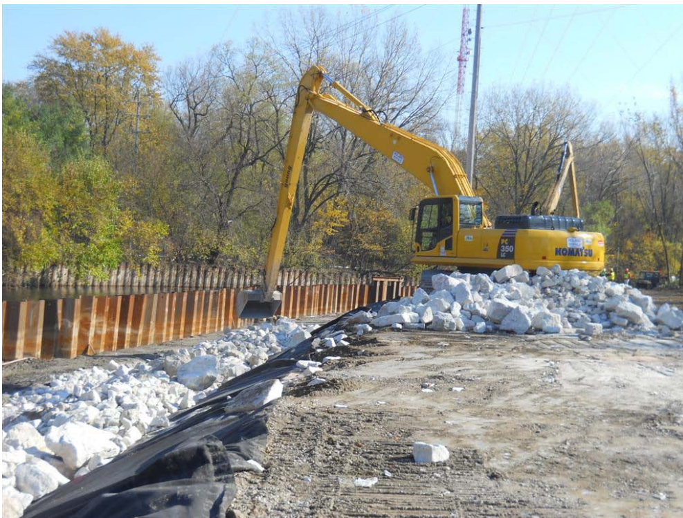
Figure 10: Riprap being placed south of Green Bay Ave. Bridge Zone 1 (11/1/2011)
