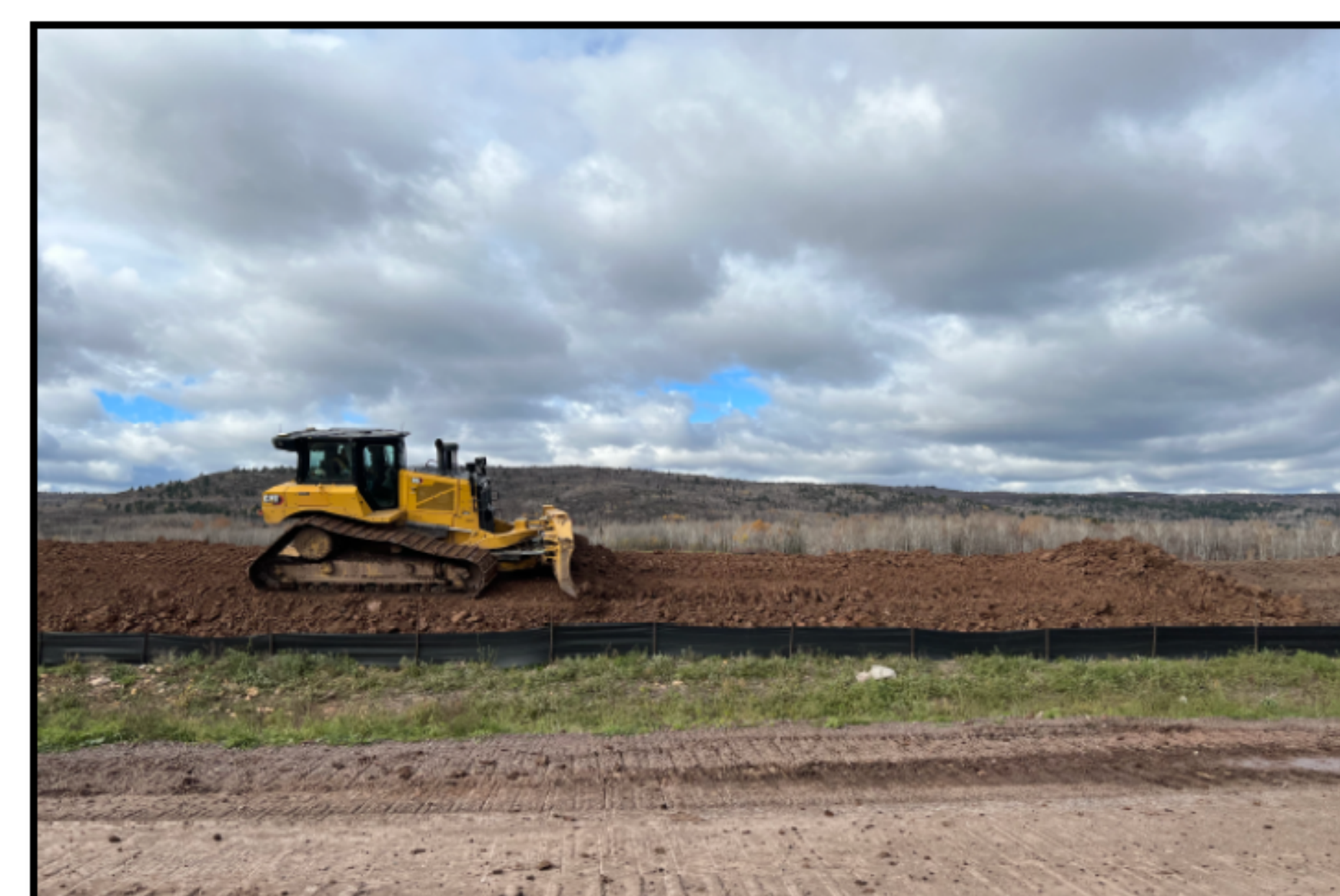
Berm construction for the OU-J CDF at Spirit Lake.
