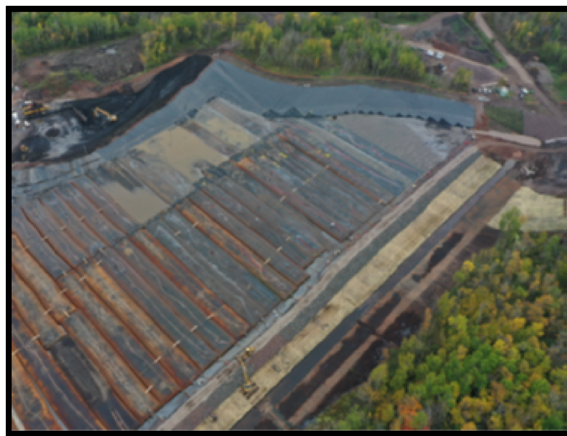
Dredge material is pumped into Geotubes® located in the Upland CDF. Geotubes® are specially engineered tubular, bag-like filters used to remove water from the dredge material before processing.
