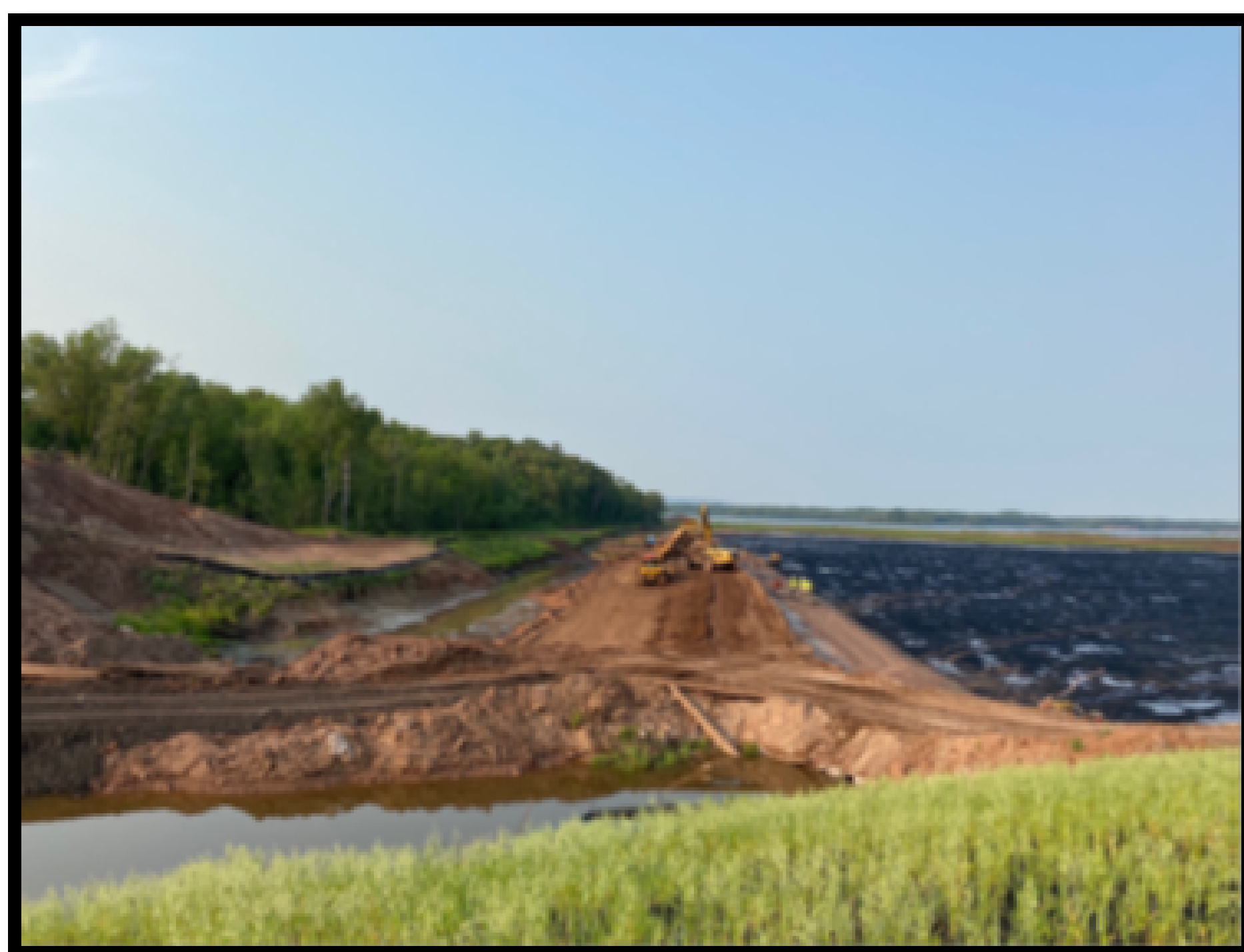
During construction, high strength fabric is placed over the Upland CDF.
