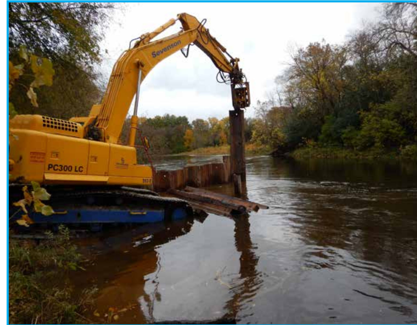
Install Sheetpile Dam
