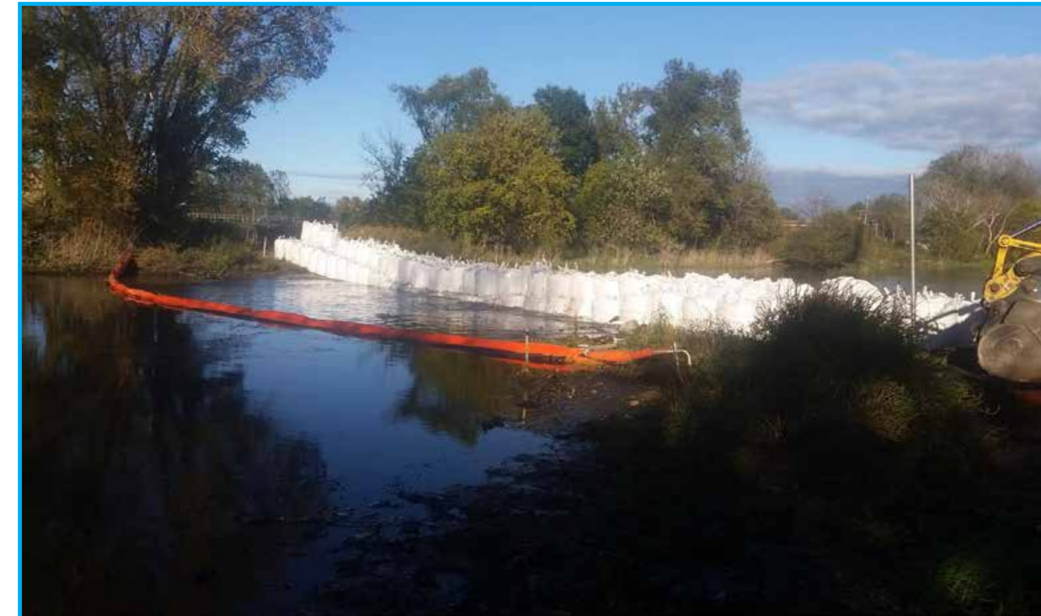
Install Super Sack Dam
