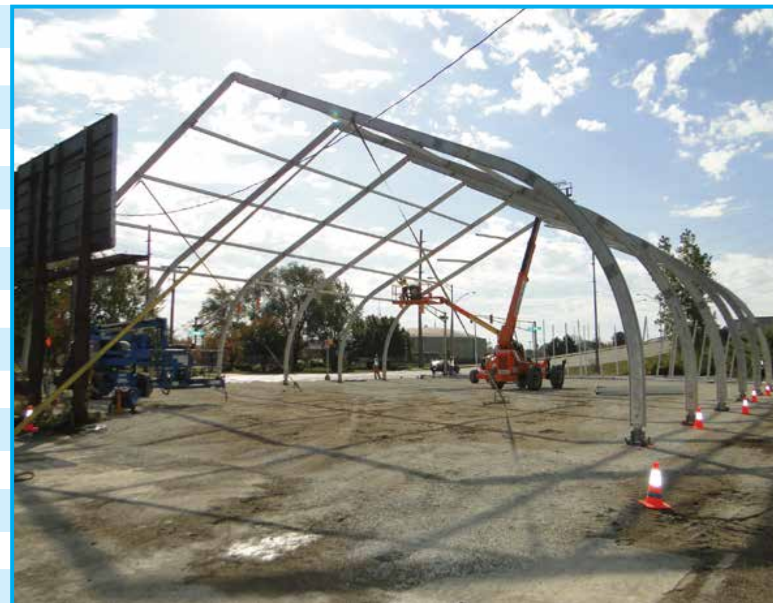
Framing Temporary Structure
